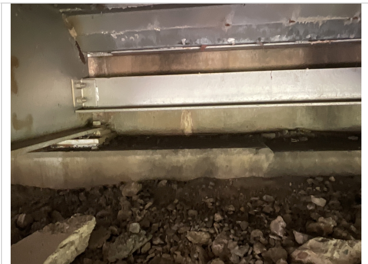
Bent 1 cracks with efflorescence in back wall.
