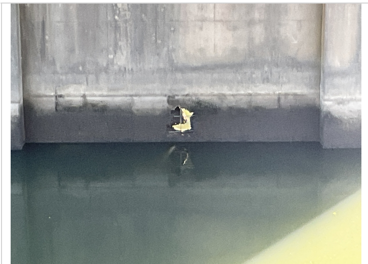
Pier wall 5 severe abrasion.
