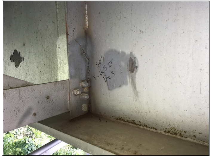
sp7 g3 dia3 repair welds have broken and crack has migrated through diaphragm clip/stiffner
