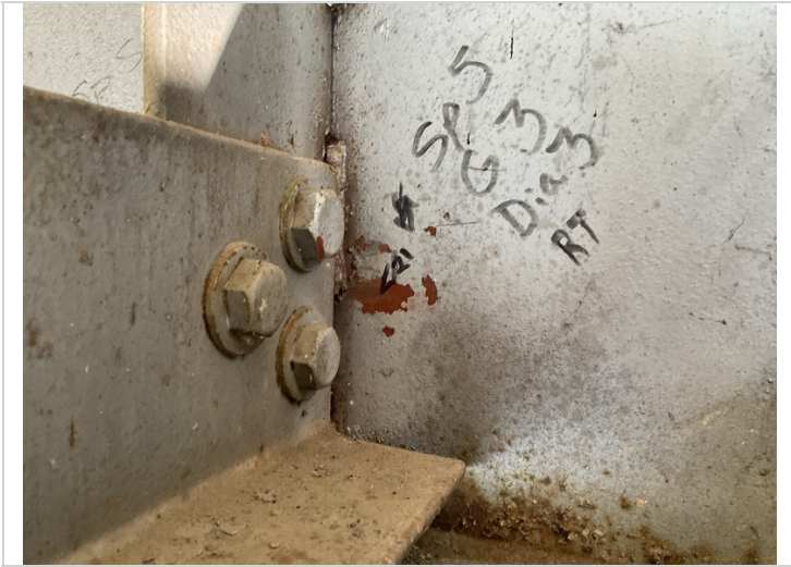
Span 5 girder 3 diaphragm 3 right side ahead. Crack in the web. Common both sides of girder ahead and back.
