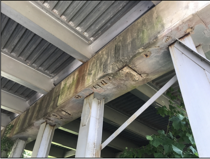
Bent 3, spalls with exposed rebar on the cap.
