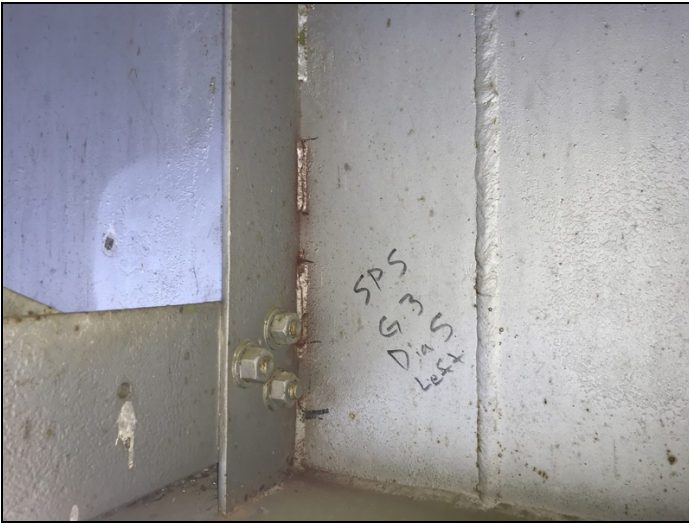
Span 5, girder 3, diaphragm 5, cracks in welds.
