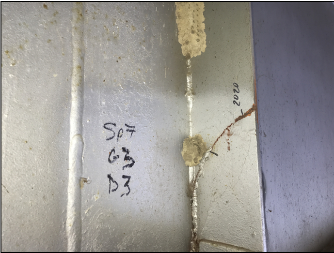
Span 7, girder 3 diaphragm 3, crack in diaphragm stiffener has grown.
