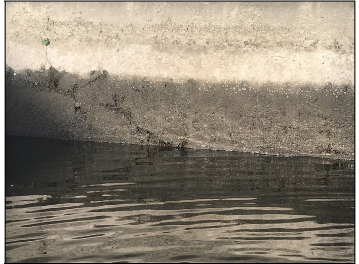
Pier 2 ahead abrasion with exposed rebar to pier wall.
