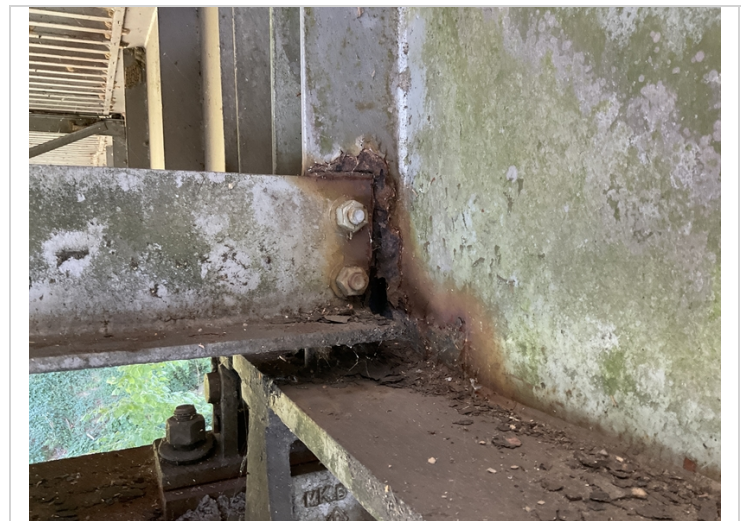
Pier 2 girder 2 span 4, section loss to lower web and hole in stiffener at diaphragm connection.
