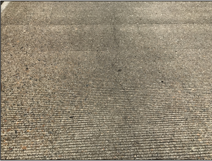
Span 9 longitudinal cracks.
