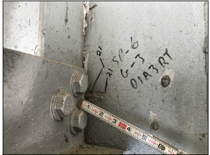
Span 6 girder 3 right side at diaphragm 3 ahead crack in the web.
