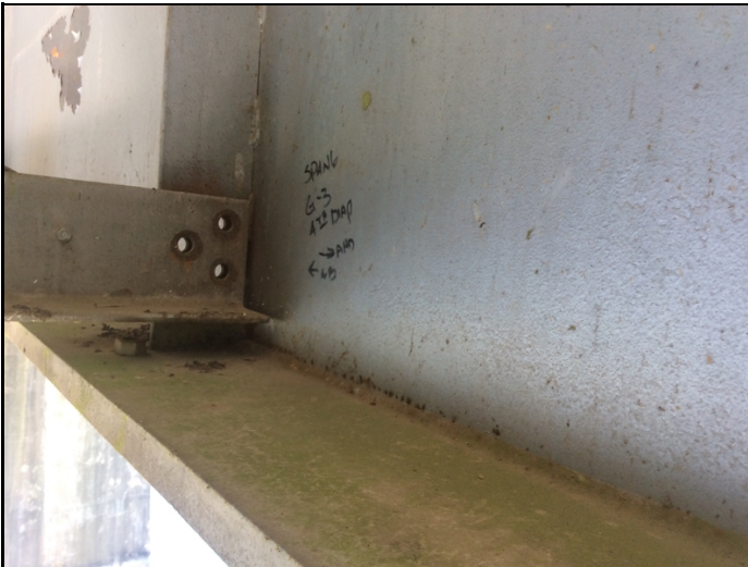
Span 6 girder 3 4th diaphragm has missing bolts
