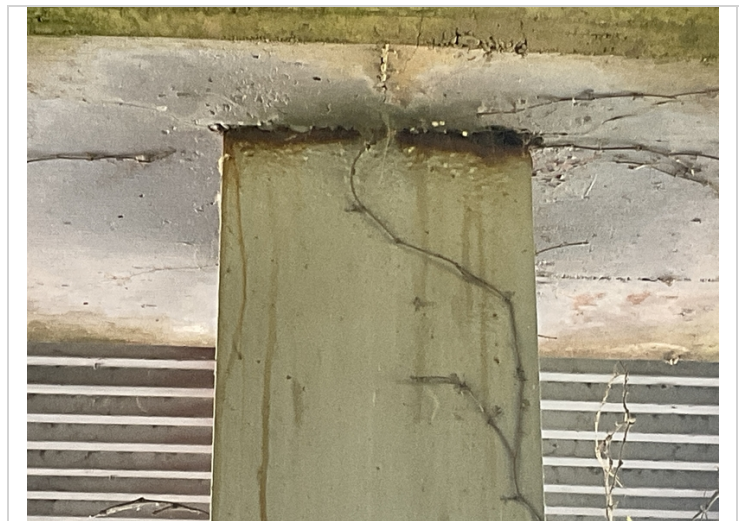
Bent 3 steel pile 3 deep pitting to flange at cap.
