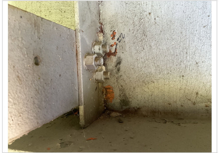
Span 7 girder 3 diaphragm 4 left side back of diaphragm cracks in the web.
