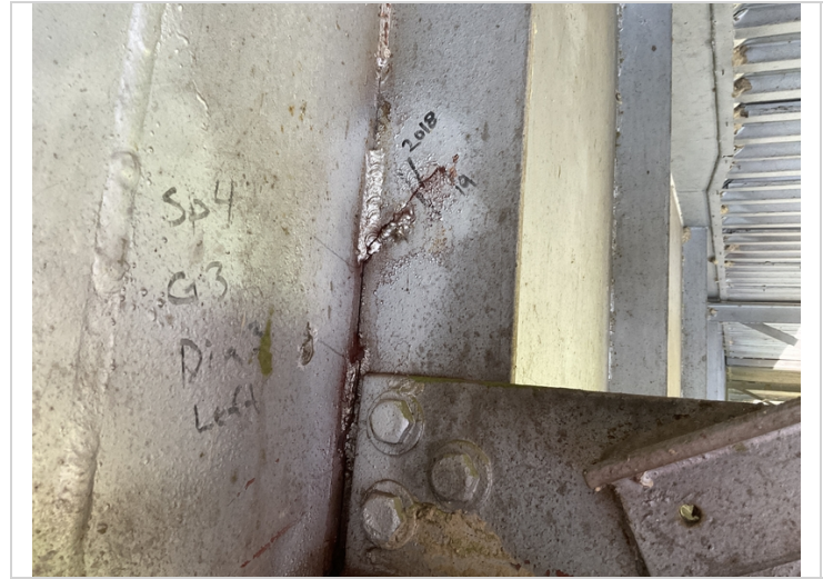
Span 4 girder 3 diaphragm 3 crack in the vertical diaphragm brace.
