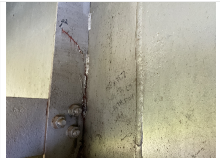
Span 7 girder 3 diaphragm 5 left side vertical diaphragm bracket at web crack has propagated 1" 1/8"
