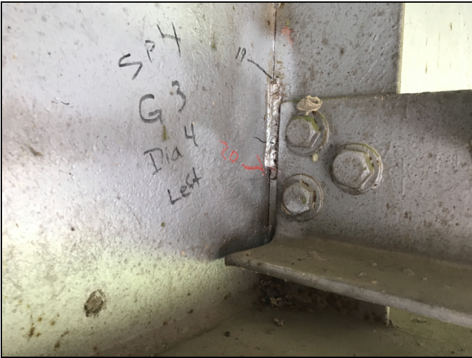
Span 4, girder 3, diaphragm 4, crack in weld has grown.
