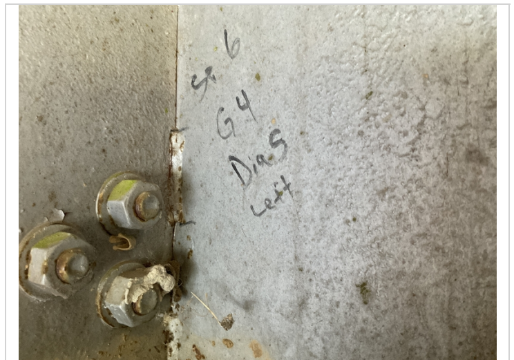
Span 6 girder 4 diaphragm 5 back broke weld.
