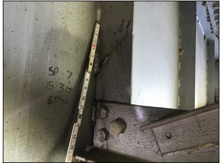
Span 7 girder 3 left side at diaphragm 6 cracked welds and crack in the vertical diaphragm stiffener. Crack has propagated a half inch since last inspection
