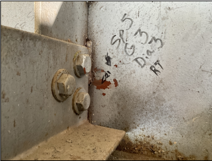
Span 5 girder 3 diaphragm 3 right side ahead. Crack in the web. Common both sides of girder ahead and back.
