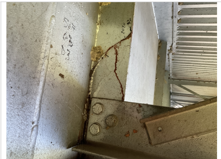
Span 7 girder 3 diaphragm 3 left side crack has propagated all the way thru the diaphragm vertical diaphragm bracket at web.
