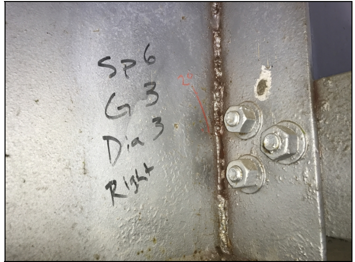
Span 6 girder 3 diaphragm 3, cracks in weld.
