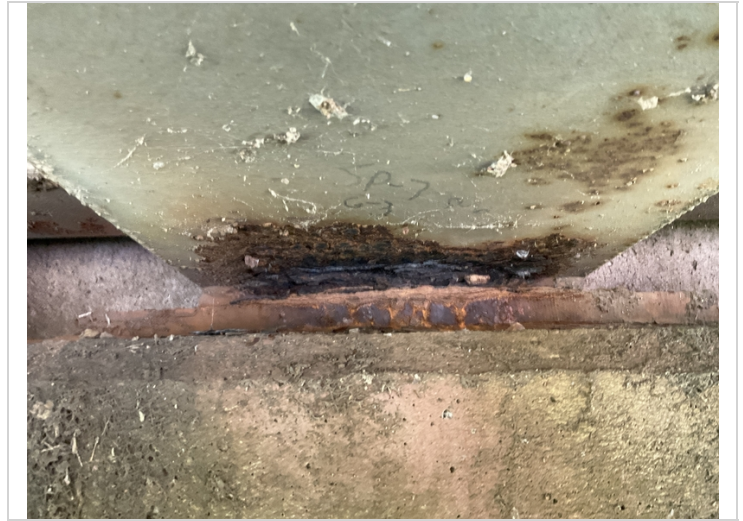
Span 7 at pier 5 girder 3 bottom flange deep pitting.
