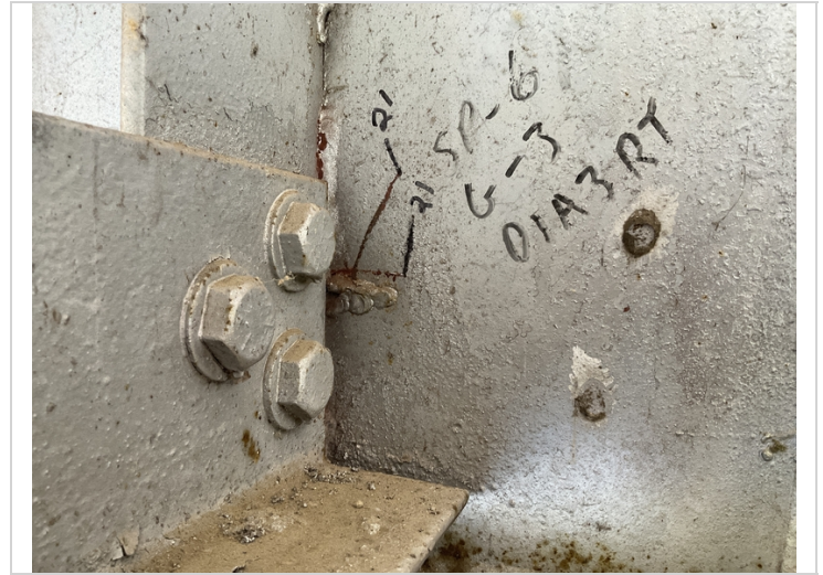
Span 6 girder 3 diaphragm 3 right side ahead cracks in the web.
