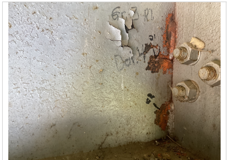
Span 7 girder 3 diaphragm 4 right side back of diaphragm cracks in the web.
