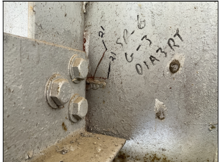
Span 6 girder 3 diaphragm 3 right side ahead cracks in the web.
