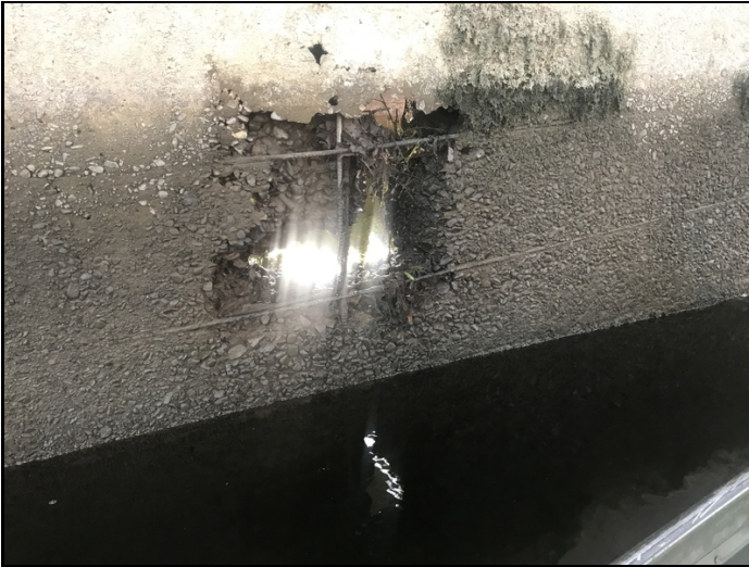
Pier wall 5 has severe abrasion with exposed rebar.
