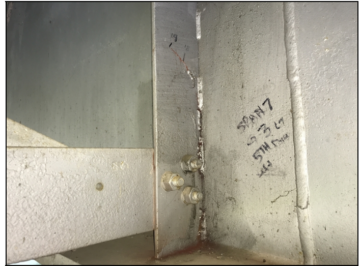
span 7 g3 d5 crack in diaphragm clip/ stiffener has 1 3/4" of growth
