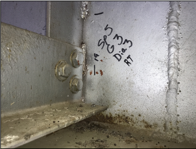
Span 5 g3 d3 has a 1 1/2" Crack in web
