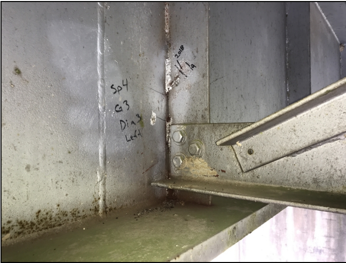
Span 4 g3 dia 3 crack in diaphragm clip/stiffener has 3/4" growth
