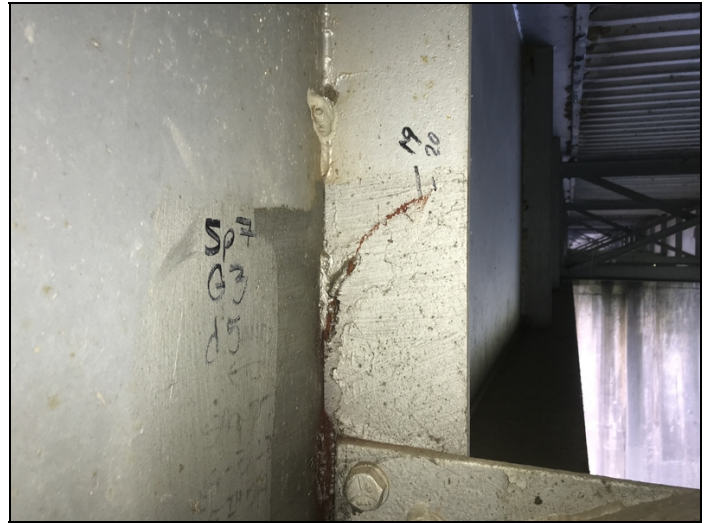
Span 7, girder 3, diaphragm 5, crack in stiffener has grown.
