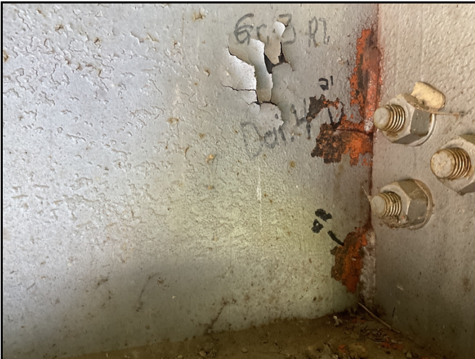
Span 7 girder 3 diaphragm 4 right side back of diaphragm cracks in the web.
