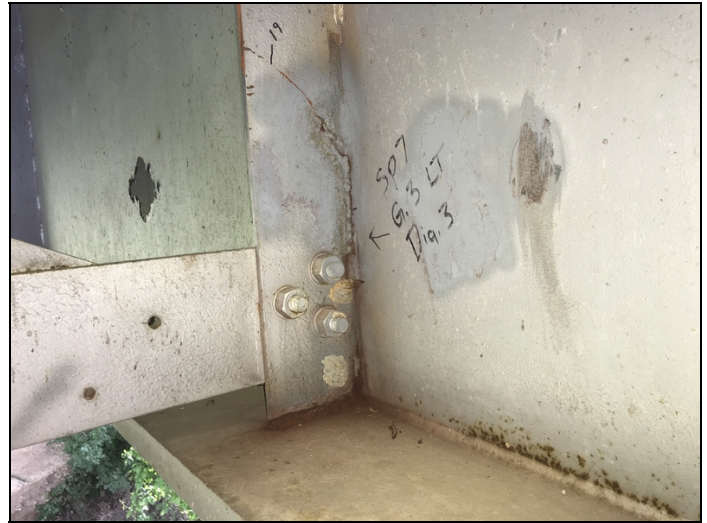
sp7 g3 dia3 repair welds have broken and crack has migrated through diaphragm clip/stiffener
