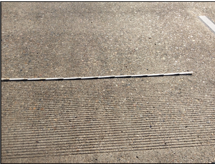
Span 3, longitudinal cracks up to .025".
