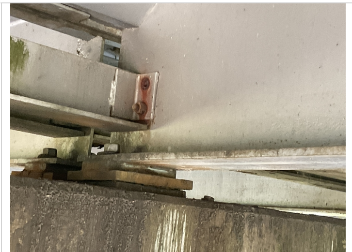
Span 2 beam 3 missing diaphragm bolt.
