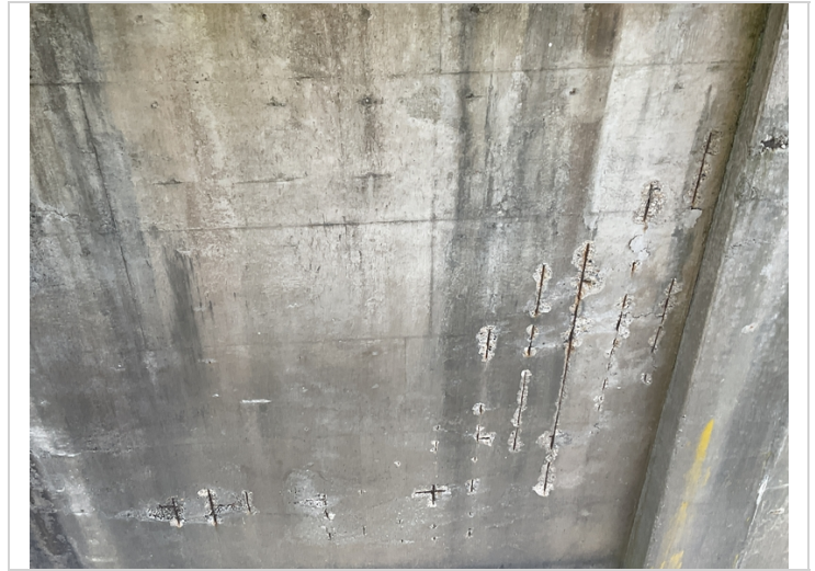
Pier wall 4 back spalls with exposed rebar.
