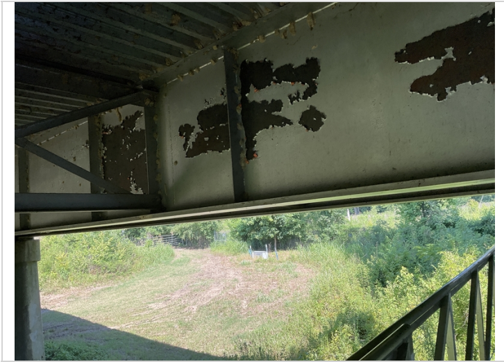
Span 3 girder 2 peeling paint. Common all spans.
