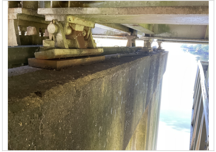
Pier 4 bearing are rotated back.
