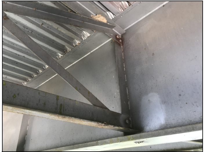
Span 5, loose bolts in top of diaphragm
