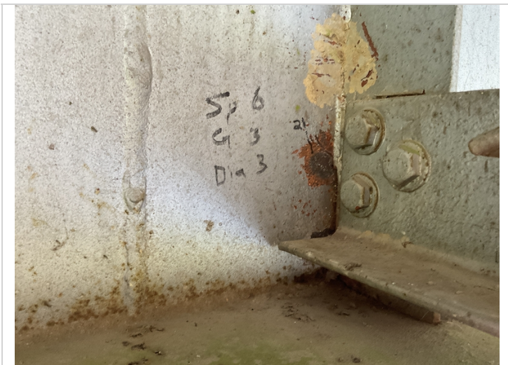
Span 6 girder 3 diaphragm 3 left side ahead crack in the web. Common back side of diaphragm this location.
