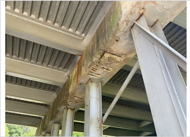
Bent 3 spalls with exposed rebar in bottom of pier cap.
