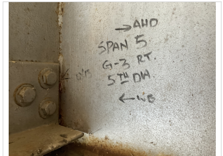
Span 5 girder 3 diaphragm 5 broke welds. Common ahead and back both sides of girder.
