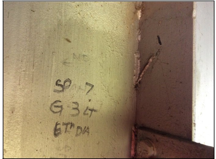
Span 7 girder 3 diaphragm 6, crack in stiffener.
