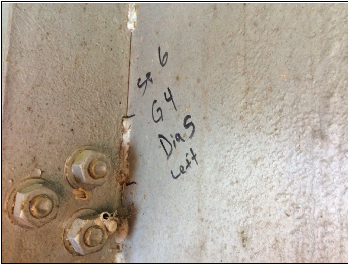
Span 6 girder 4 diaphragm 5 crack in weld.
