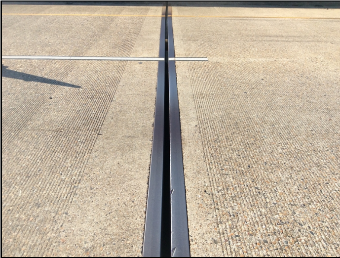
Pier 4, joint seal has fallen out.
