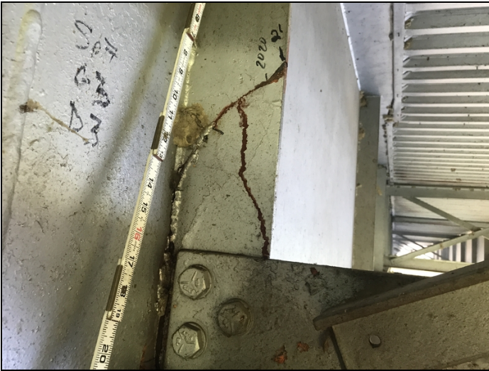
Span 7 girder 3 left side at diaphragm 3 cracked welds and crack in the vertical diaphragm stiffener. Crack has propagated a one and quarter inch since last inspection. Crack has propagated all the way thru vertical diaphragm stiffener.
