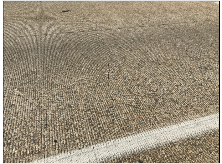
Span 7, large transverse cracks.
