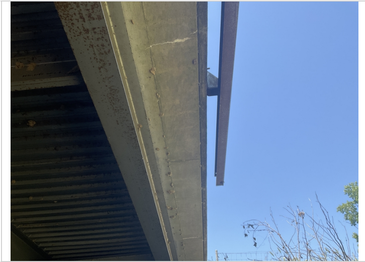
Cracks with efflorescence on left side overhang.
