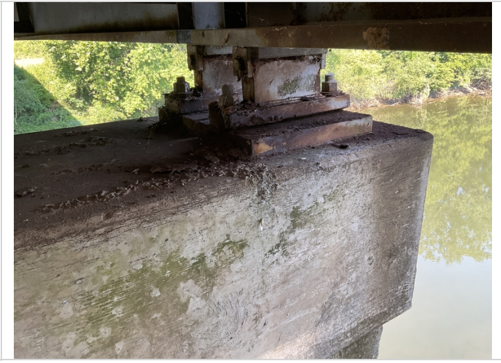
Pier 3 movable bearing under girder 1 corrosion.
