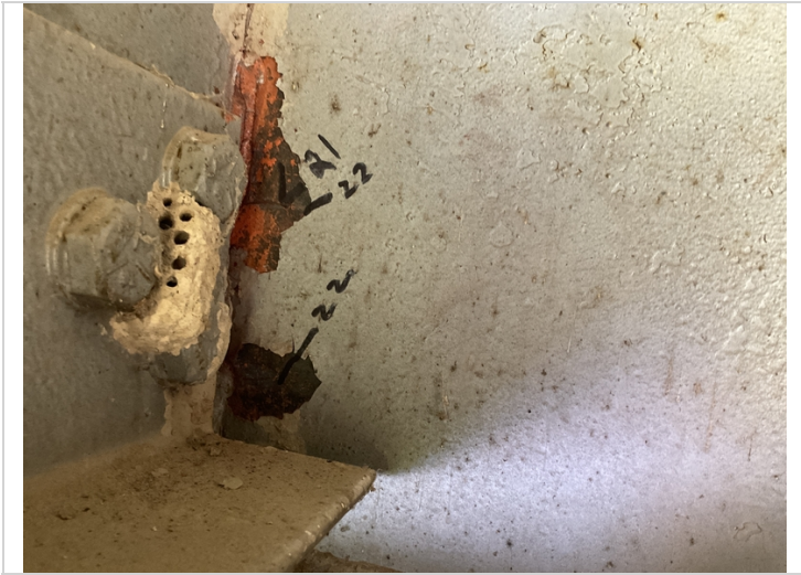
Span 7 girder 3 diaphragm 4 right side ahead of diaphragm cracks in the web.
