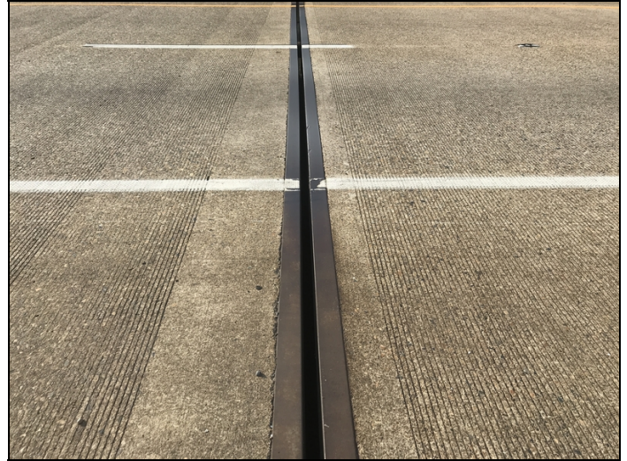
Pier 4, missing joint seal.
