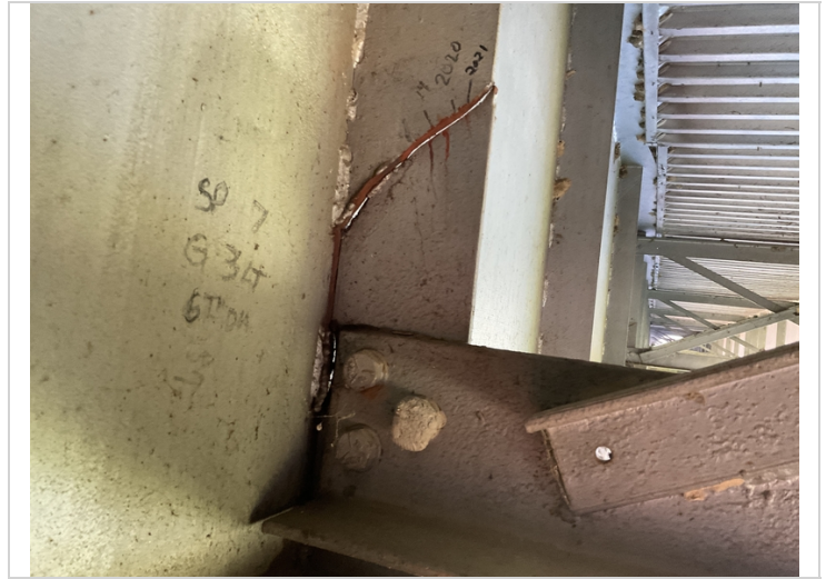
Span 7 girder 3 diaphragm 6 left side crack has propagated all the way thru the diaphragm vertical diaphragm bracket at web.
