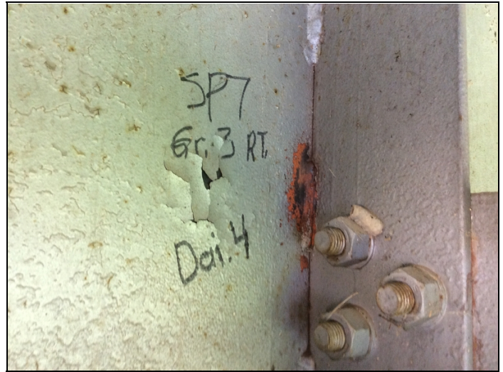
Span 7 girder 3 diaphragm 4 crack in weld.
