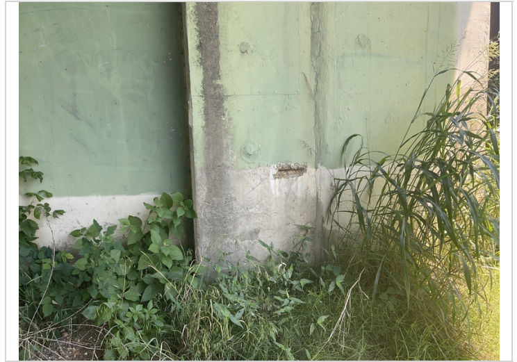
Pier wall 6 right column back spall with exposed rebar.
