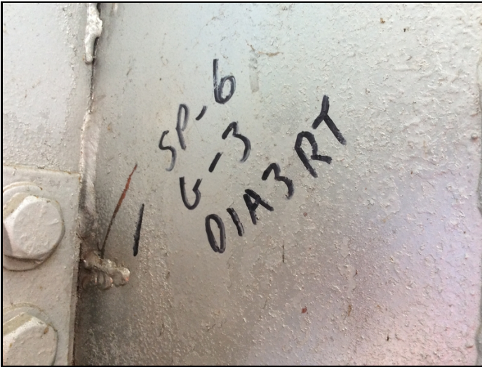
Span 6 girder 3 diaphragm 3 crack in web.
