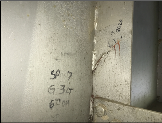
Span 7, girder 3, diaphragm 6, crack in stiffener has grown.
