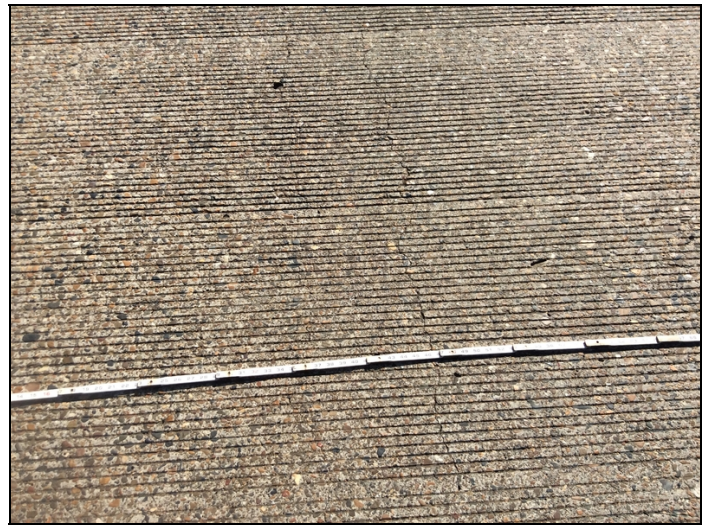
Span 8, longitudinal & transverse cracks up to .020".
