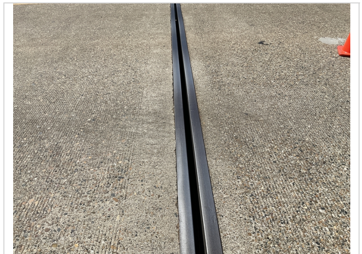
Joint seal missing b ent 4.
