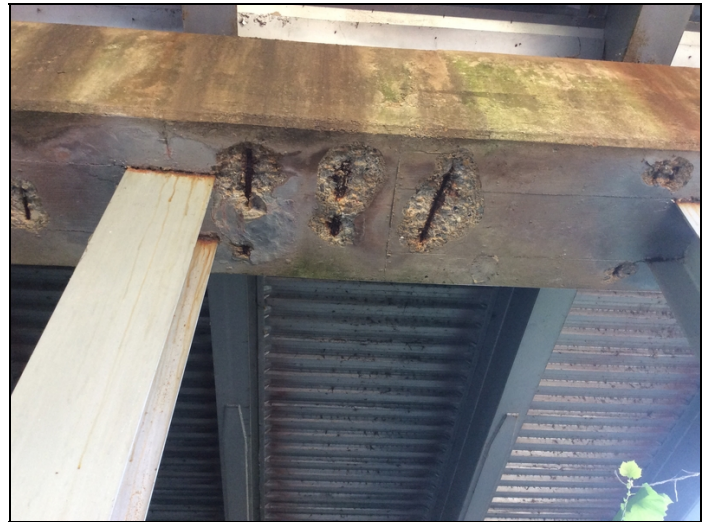
Bent 3 between piles 4 and 5 spalls with exposed reinforcing steel.
