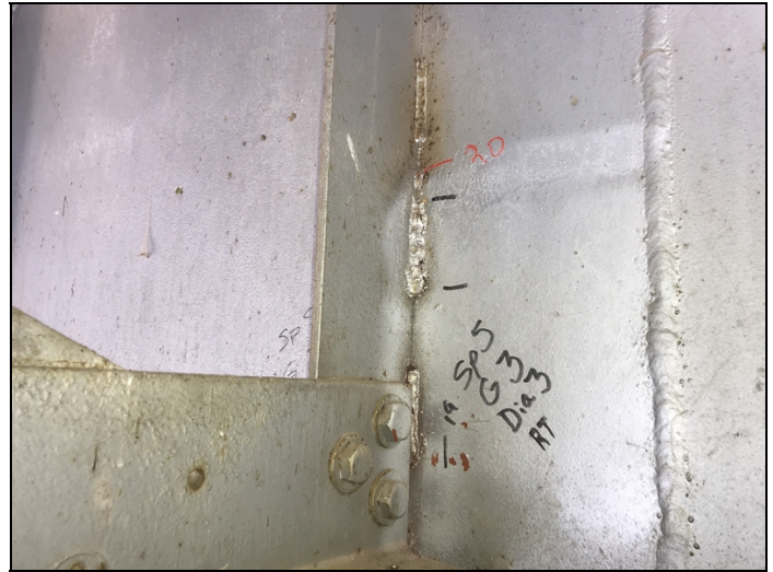
Span 5, girder 3, diaphragm 3, crack in weld has grown.
