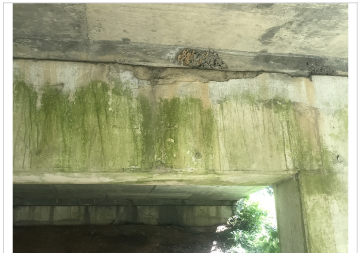
Bent 4 cap back has spalled area.
