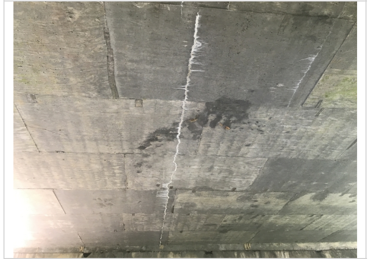
Span 1 soffit has cracks with efflorescence at centerline.
