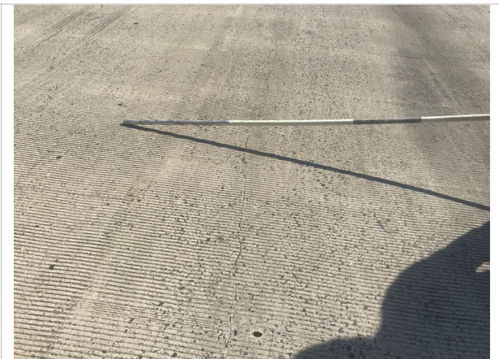
Span 1 has unsealed longitudinal crack that reflects through to the soffit.
