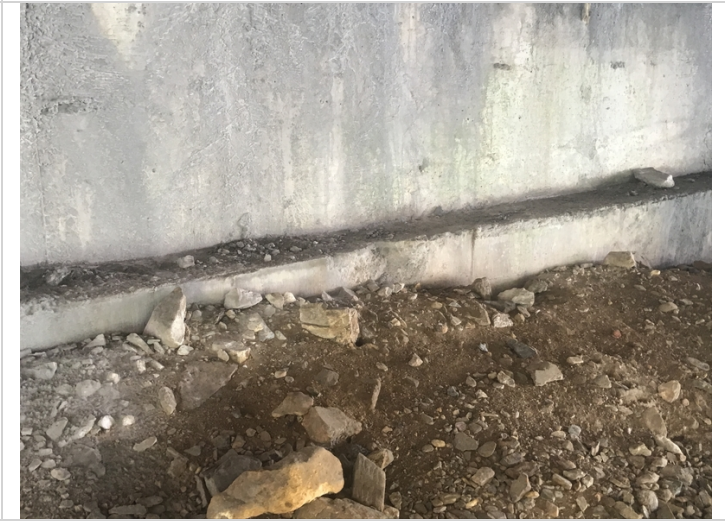
Bent 1 abutment has small spalls.
