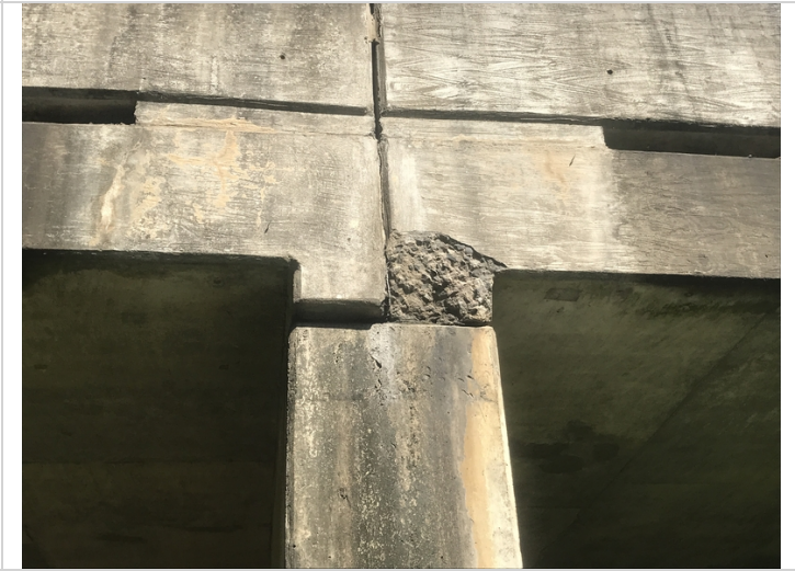
Spall in slab at span 4 above bent 4 cap right side.
