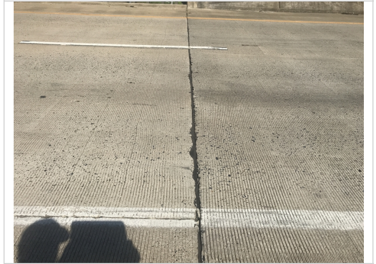
Bent 1 joint seal has lost bond and is leaking, common all joint seals.
