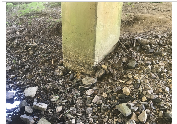
Bent 3 column 2 has abrasion, common all columns at bents 3&4.
