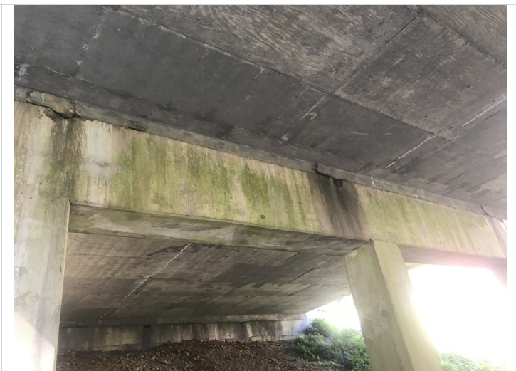
Deck haunch above bent 2 has large delams.
