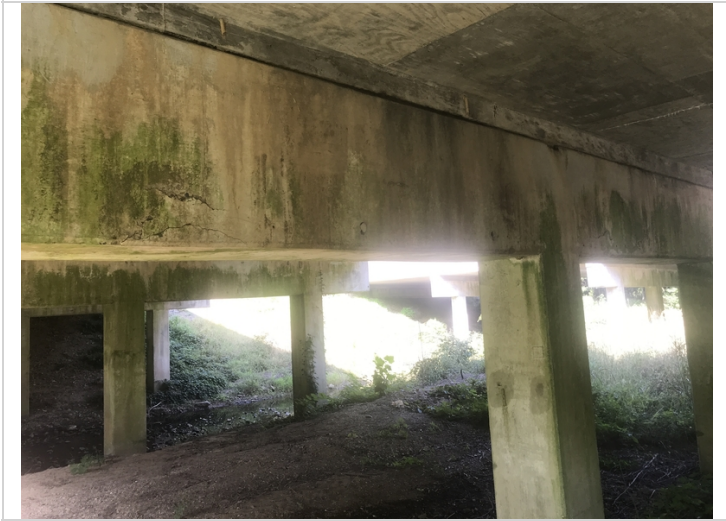
Bent 4 cap ahead has delams.
