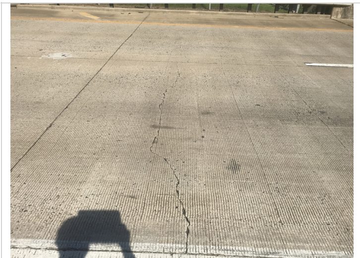
Large unsealed cracks in west approach slab.
