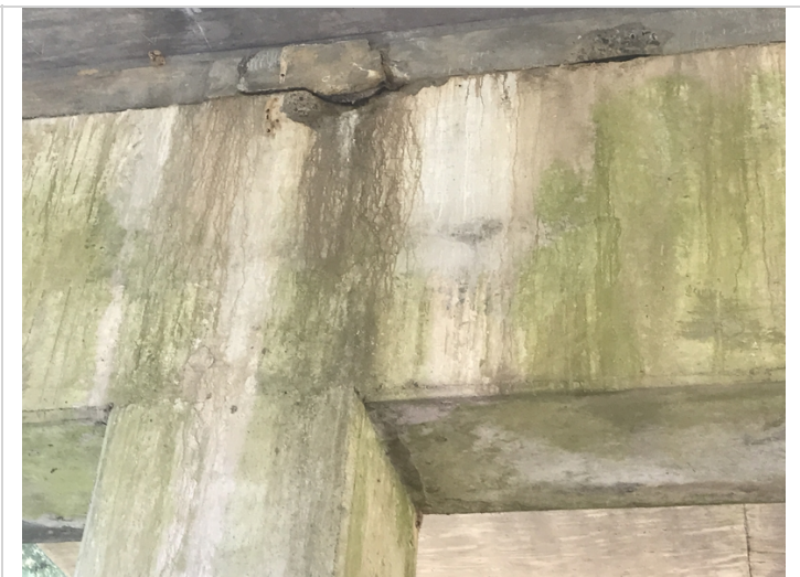
Bent 2 cap ahead has contact spall above column3.
