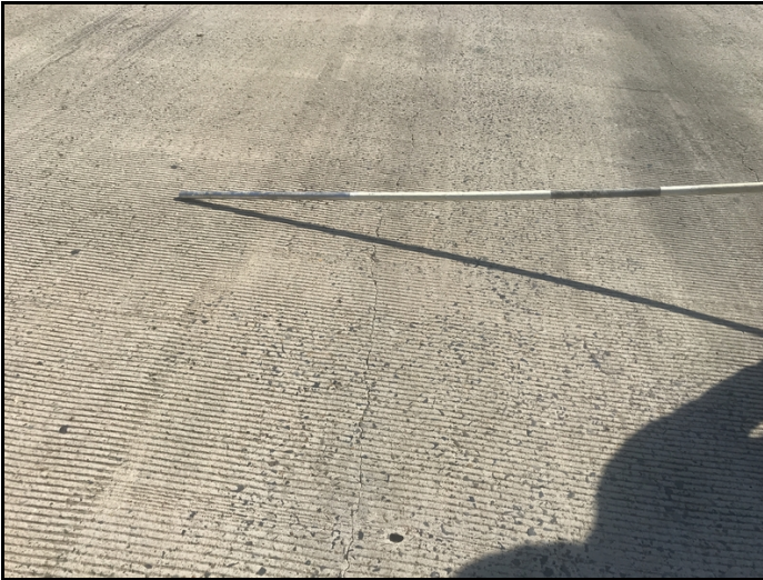
Span 1 has unsealed longitudinal crack that reflects through to the soffit.
