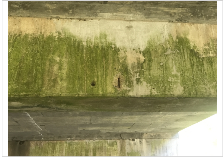
Bent 3 cap ahead has spall with exposed rebar.
