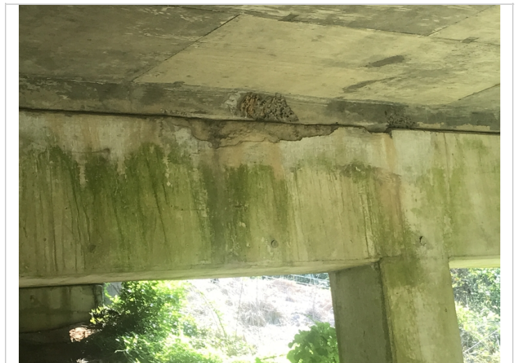
Deck haunch above bent 4 back has spalls.
