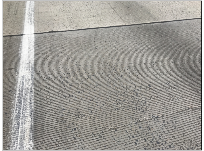
Span 3, large unsealed crack.
