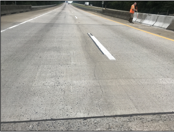
Large longitudinal crack.
