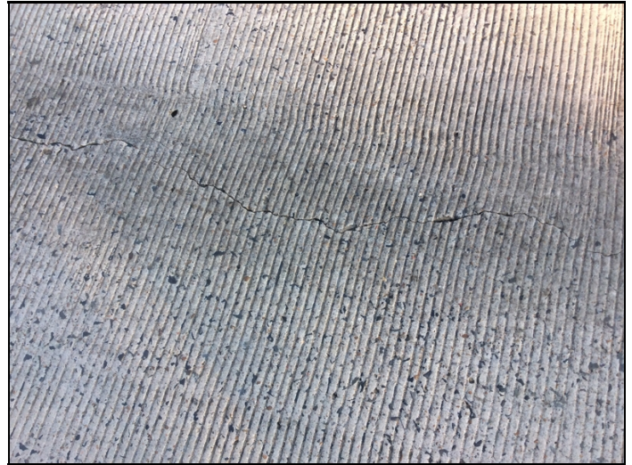
Deck has large unsealed cracks
