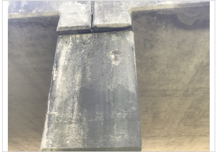
Bent 4 cap left end has small spall with exposed rebar.
