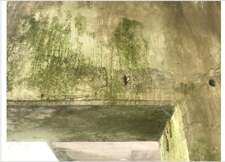
Bent 2 cap back has spall with exposed rebar.
