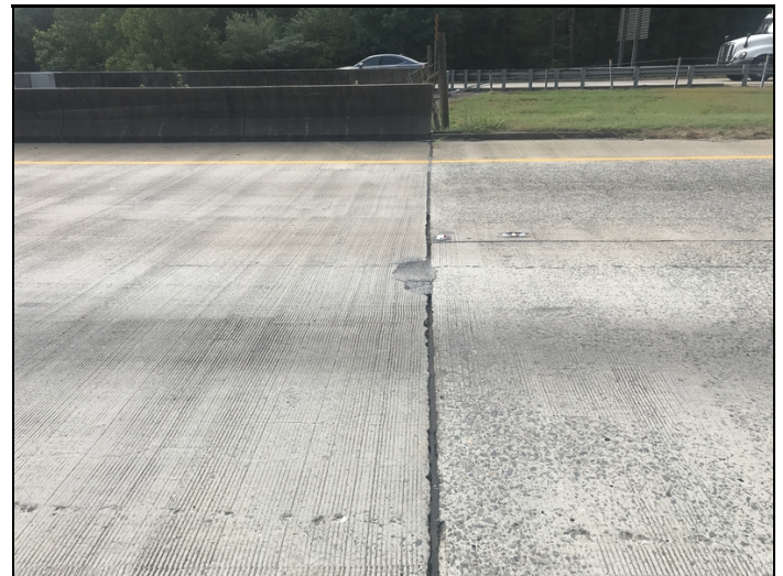
Asphalt patch span 1.
