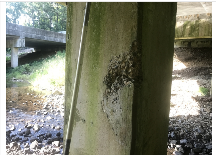
Bent 3 column 2 has spall.
