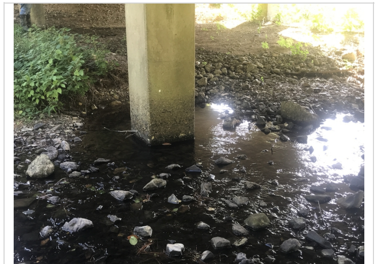
Bent 3 column 1 has abrasion, common columns 2&3.
