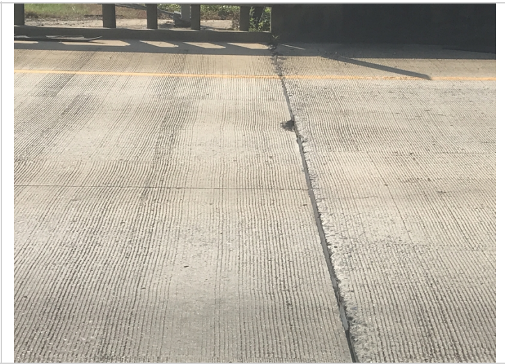
East approach slab spall
