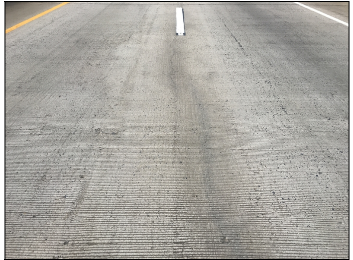
Span 4, longitudinal cracks.
