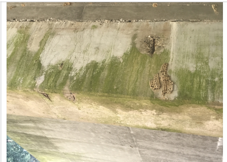
Bent 3 cap ahead and bottom have spalls with exposed rebar.
