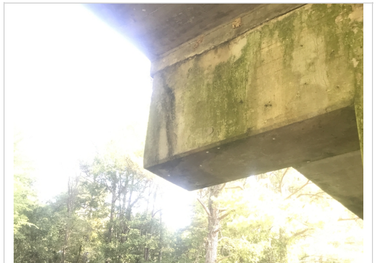
Bent 3 cap left side has patched area.
