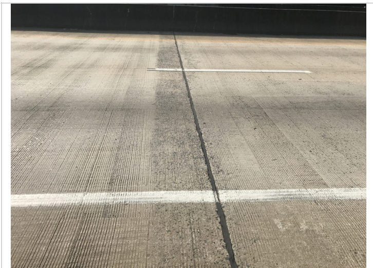
Deck at bent 3 has abrasion, common bent 2.
