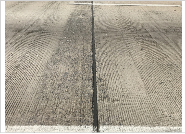
Joint seal at bent 3 has lost bond and is leaking common all joints.
