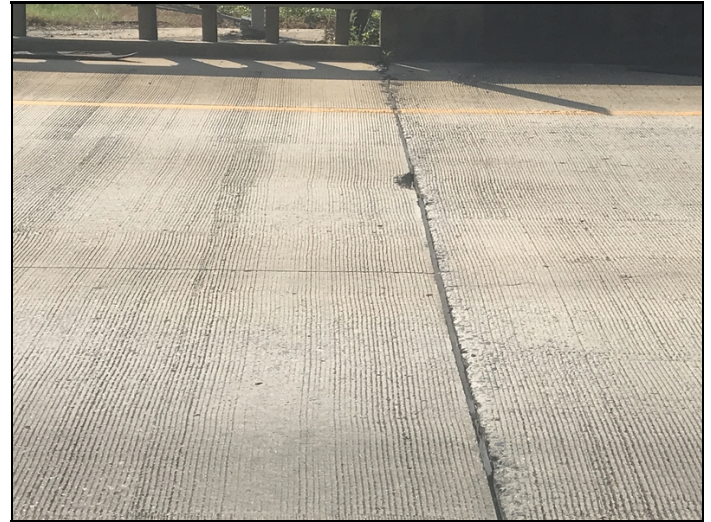
East approach slab spall
