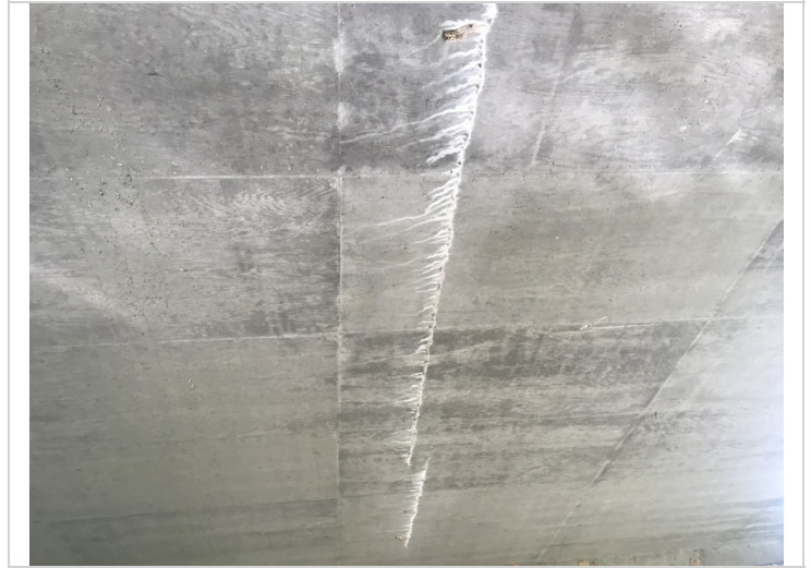
Span 2 soffit has cracks with efflorescence.
