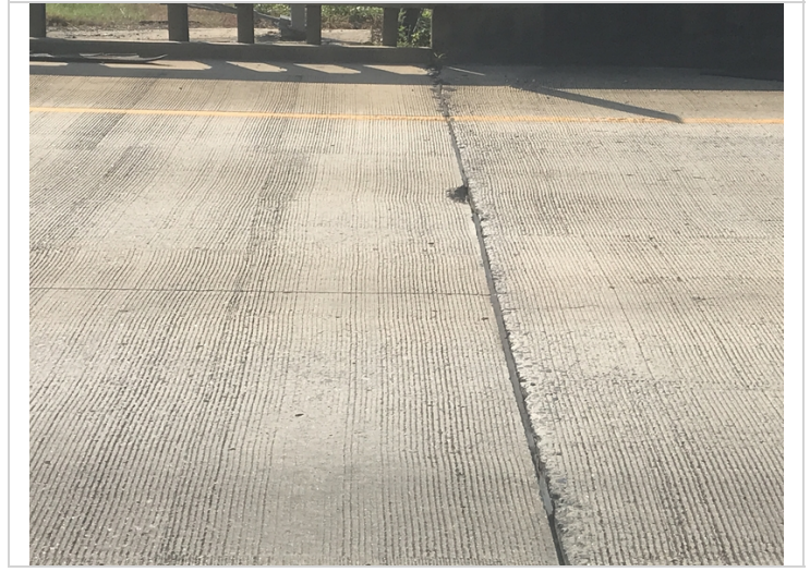
East approach slab spall
