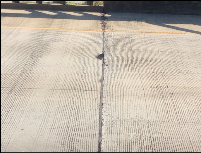
Spalls in east approach slab
