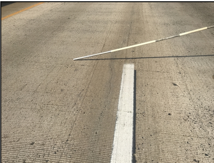
Deck span 2 has unsealed longitudinal crack that reflects through to the soffit.
