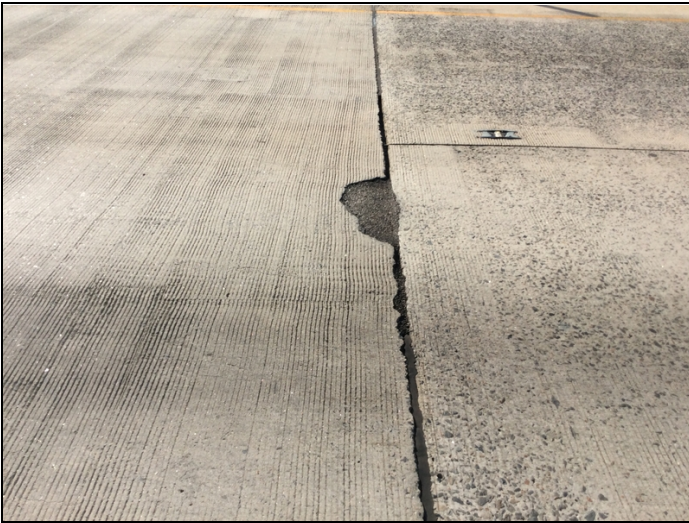
Deck has a spall filled with asphalt at west end of bridge.
