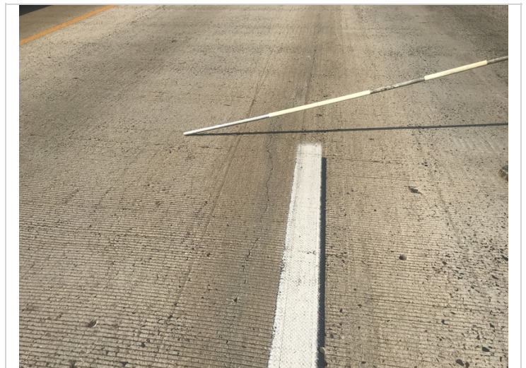
Deck span 2 has unsealed longitudinal crack that reflects through to the soffit.
