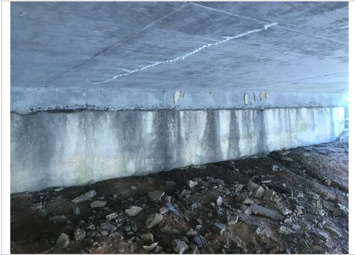
Bent 5 slab haunch has spalls entire length.
