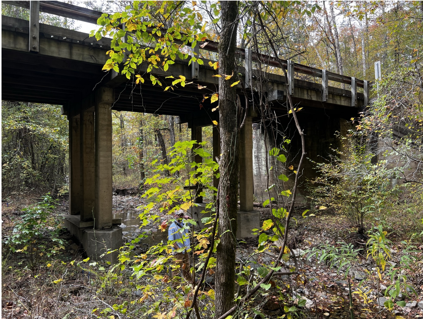
East side of bridge looking west (downstream) (October 2022)
