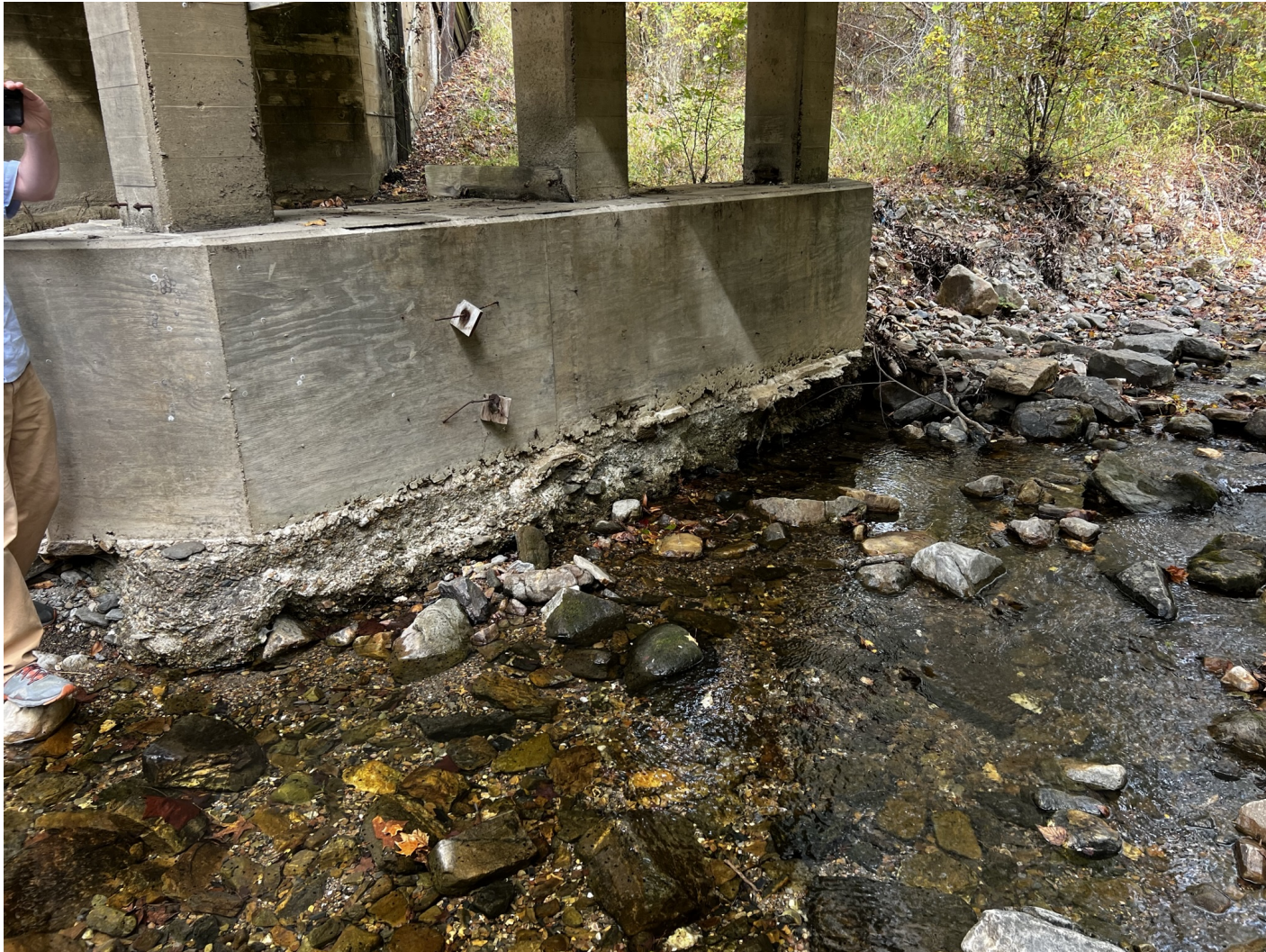
South pier footing (looking south) (October 2022)
