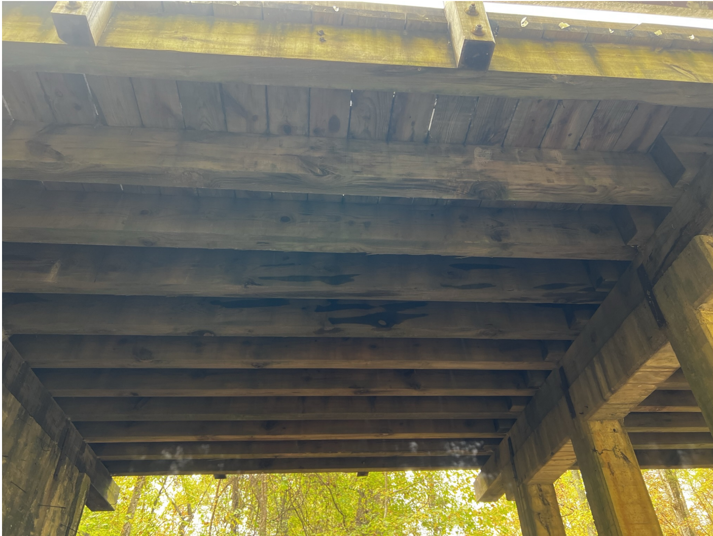
Underside of deck of the southern span (October 2022)
