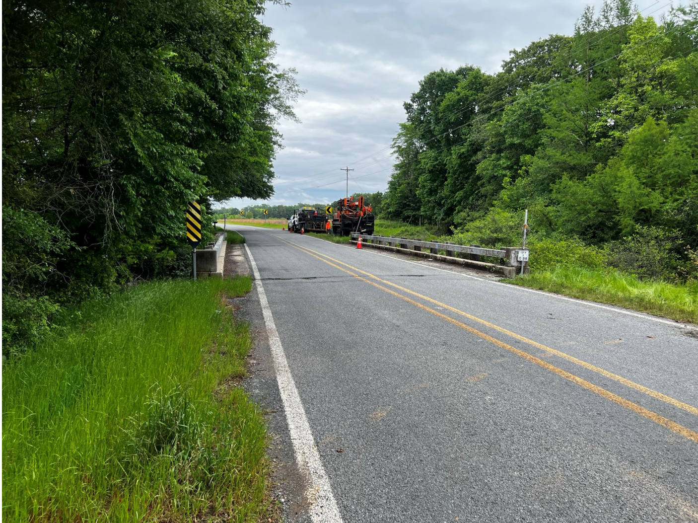
Existing Bridge - Looking North (April 2023)
