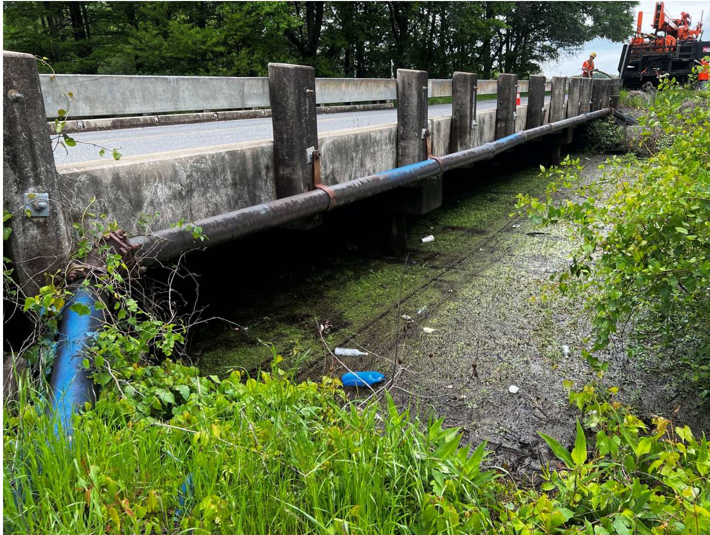
East Side of the Existing Bridge - Looking North (April 2023)
