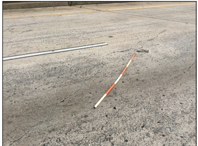
Span 3 large unsealed cracks. Common in all spans.
