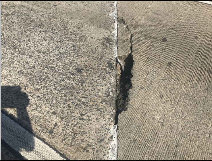
large spall at bent 6 in approach slab
