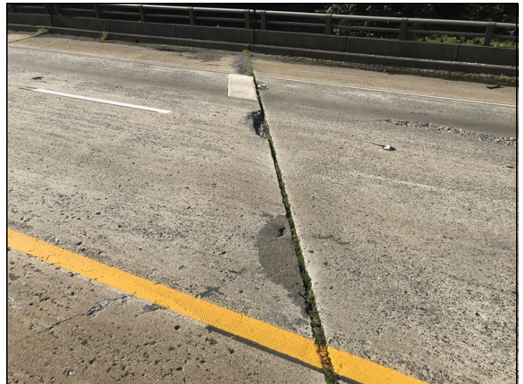
Large open spall with exposed rebar at bent 2, span 3
