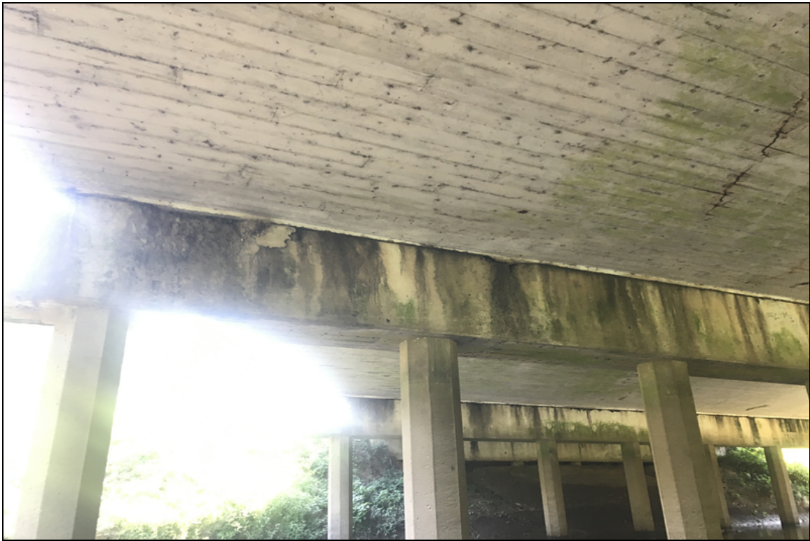
Bent 4 cap large spalls
