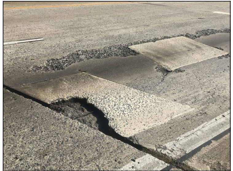
Span 2 large open spall in wheel path
