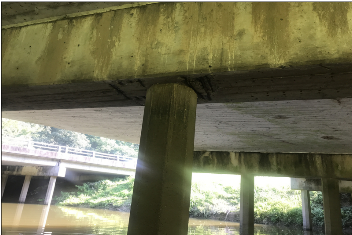
Bent 3 exposed rebar around pile 4
