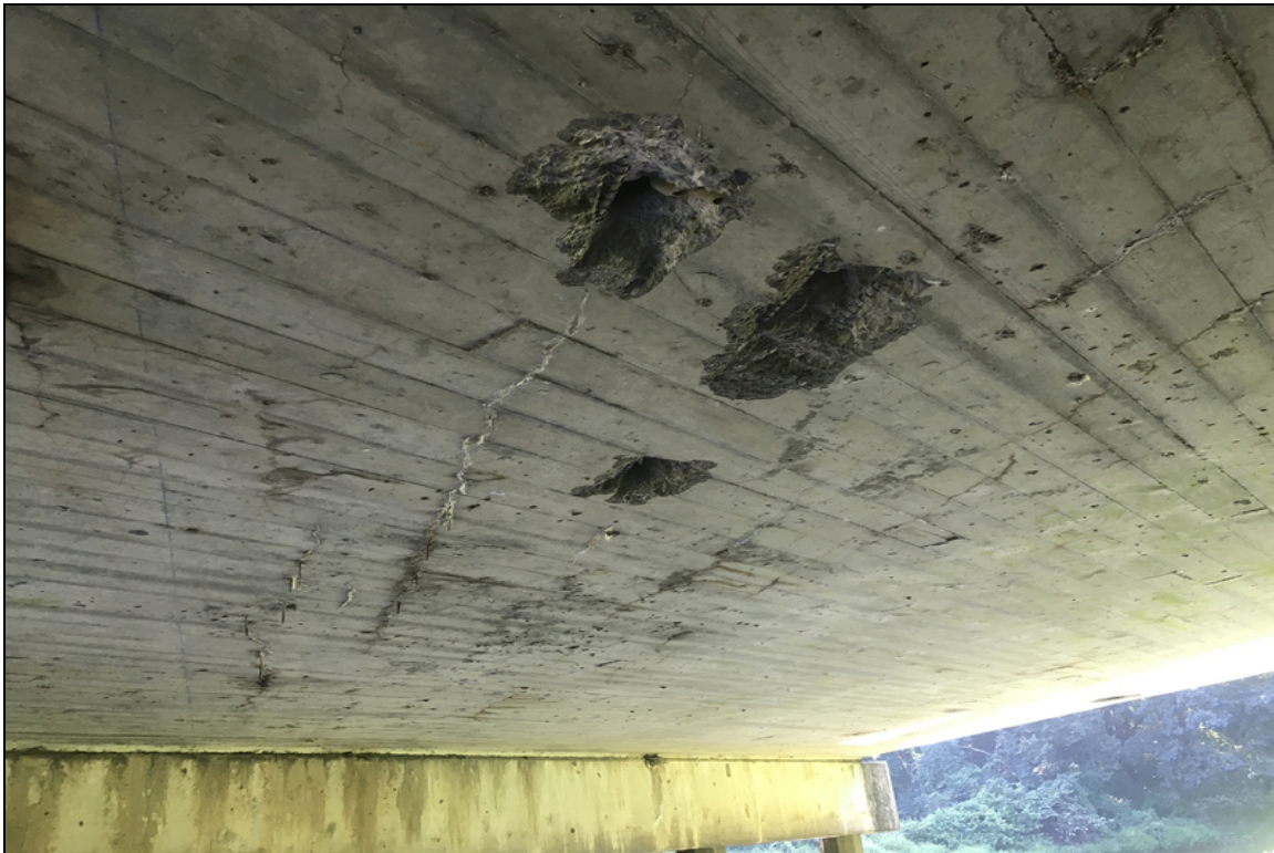
Span 2 spalls with exposed rebar on soffit
