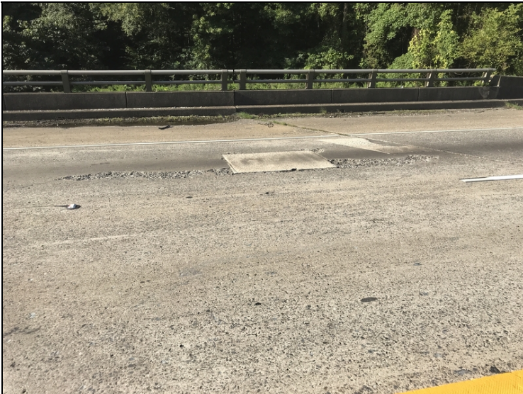
Span 2: right lane has large spall almost the entire length of span. Also spall with asphalt patch
