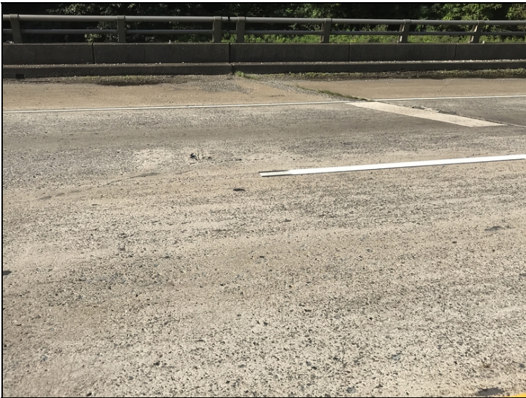
Span 3: large crack at the center line with an open spall.
