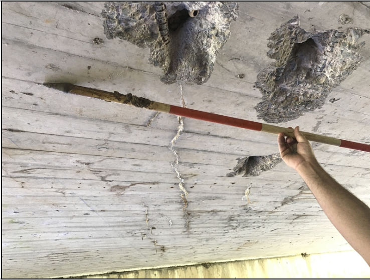
Span 2: spalls with exposed rebar in the soffit. Also multiple cracks with efflorescence staining
