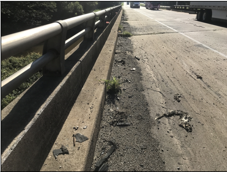
Left gutter line full of debris
