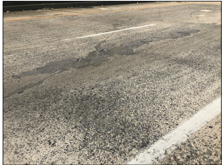
Span 2 spalls and spalls filled with asphalt
