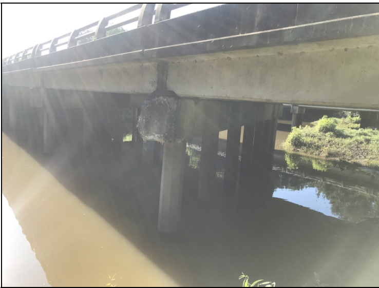
Left side of bent 2 is spalled and cracked with efflorescence build up
