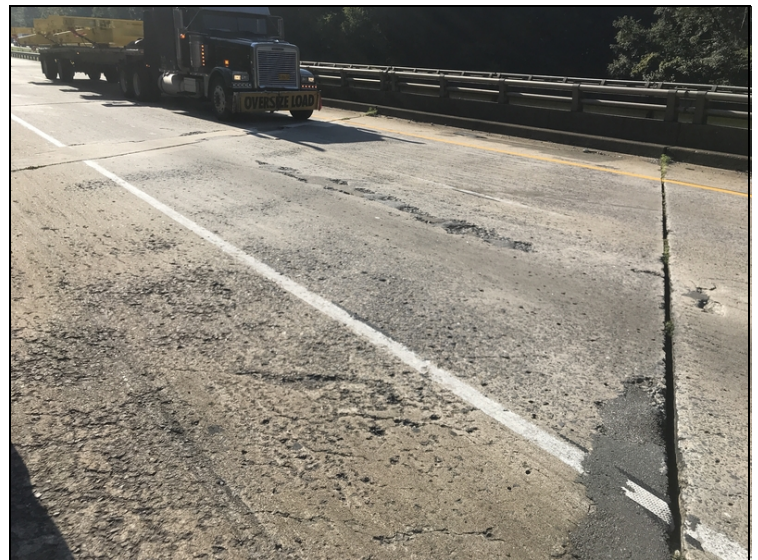
Span 2: Multiple spalls and spalls filled with asphalt that is deteriorating
