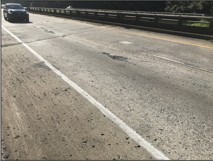
Span 1: open spall in outside lane
