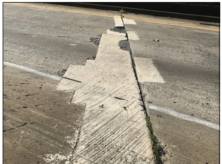
Span 3: large open spall that was patched with asphalt has deteriorated exposing steel
