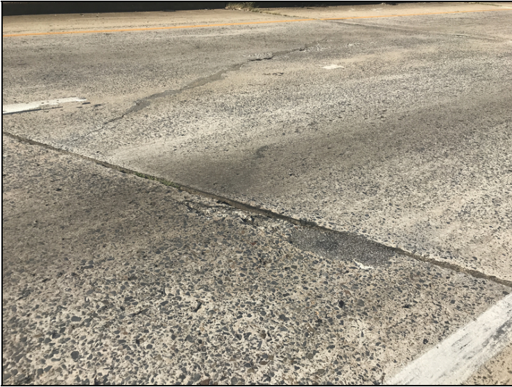
Span 4&5 spalls
