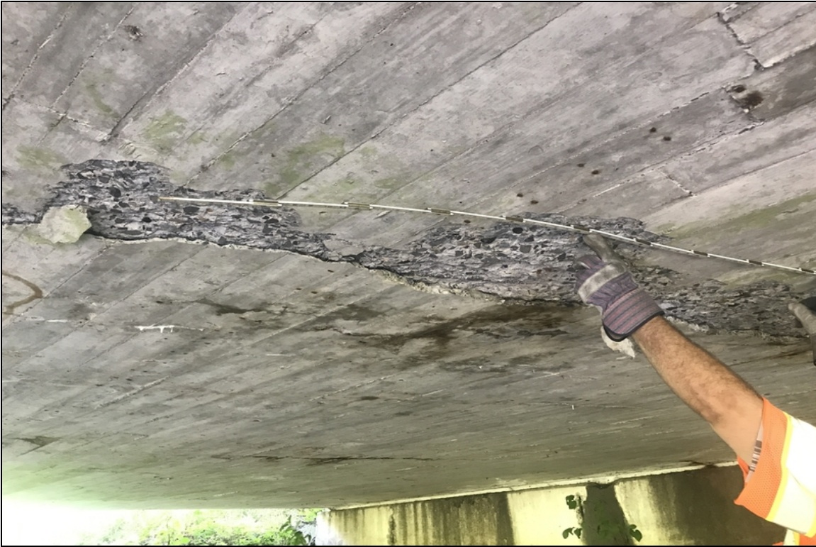
Span 5 large spall with exposed rebar and delam
