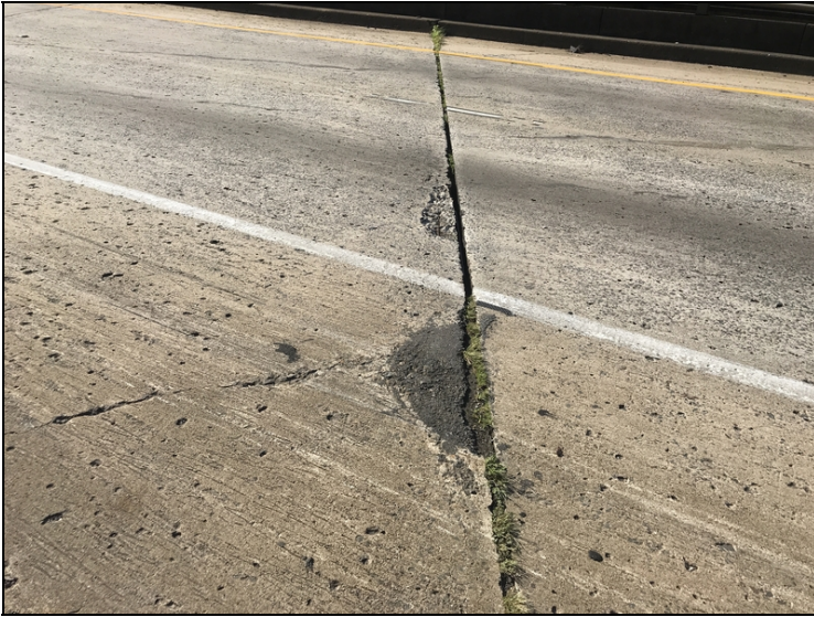
Span 5 at bent 5: spall with exposed rebar in travel lane
