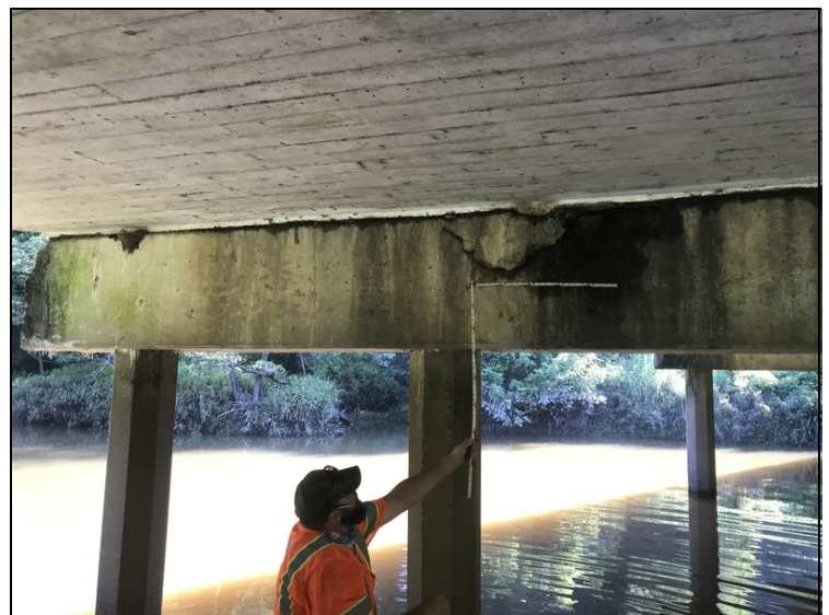
Bent 3: Large spall with exposed rebar and large delam above pile 2 at the key way
