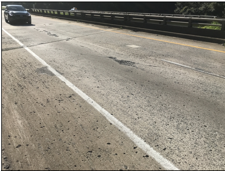
Span 1: open spall in outside lane
