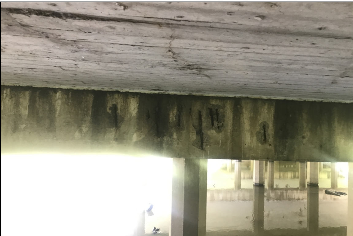
Bent 5 spalls with exposed rebar on ahead face
