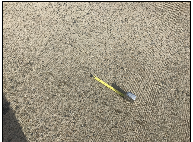
Span 1 longitudinal cracks
