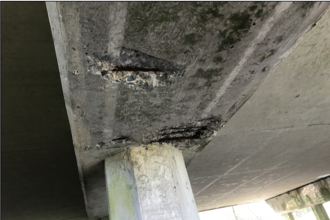
Spalls with exposed rebar at Bent 3 bottom of cap.
