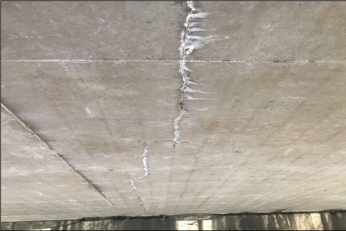
Cracks with efflorescence at centerline in Span 3.
