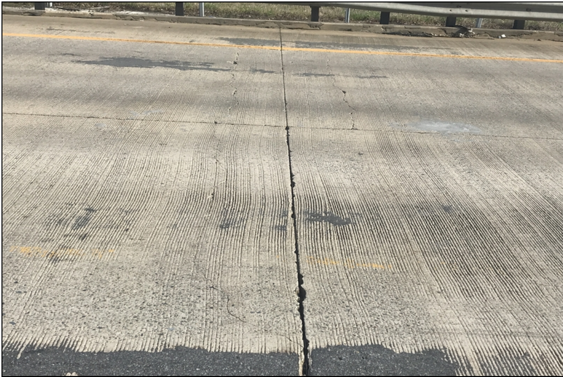
Cracks in West approach slab
