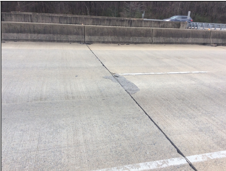
Span 2 at bent 3: large spall that has an asphalt patch.
