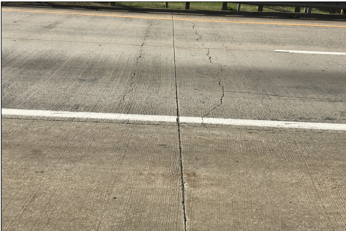
Large cracks in East approach slab
