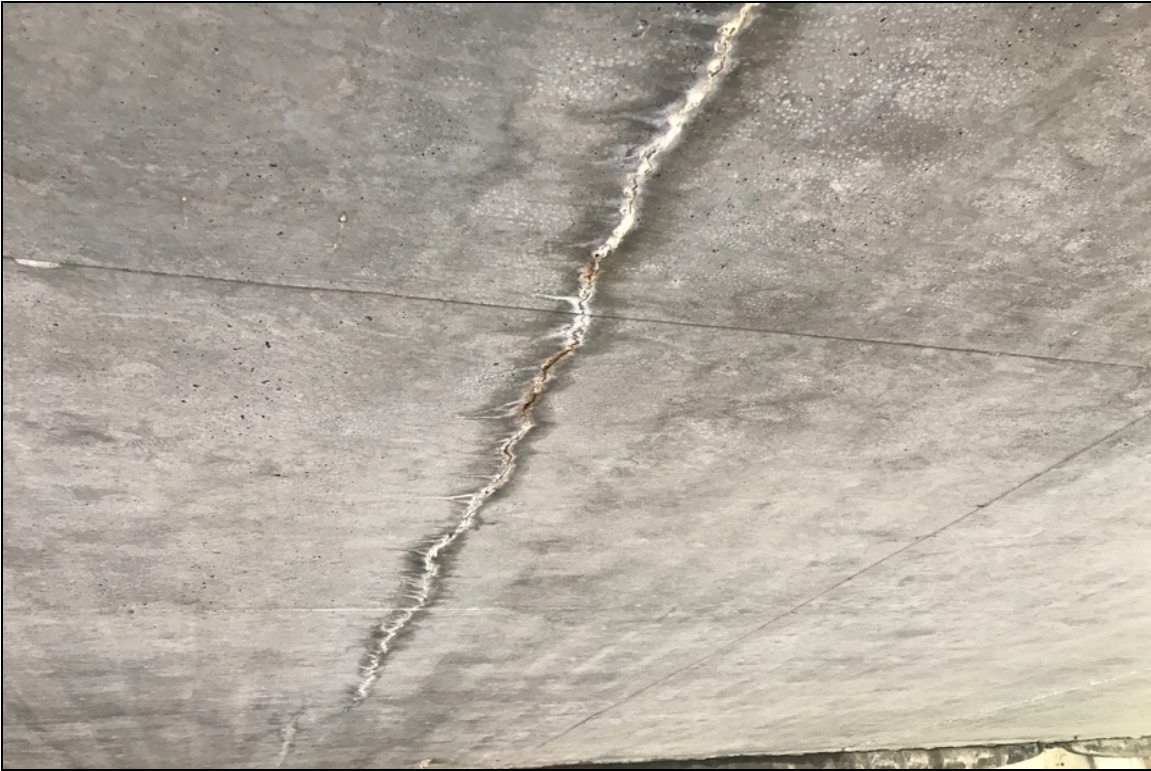
Cracks with efflorescence at centerline of span 3.
