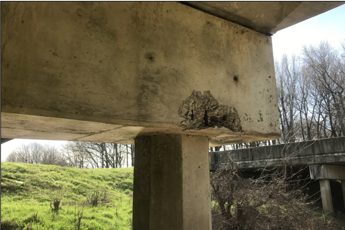
Spall with exposed rebar on bent 2 cap
