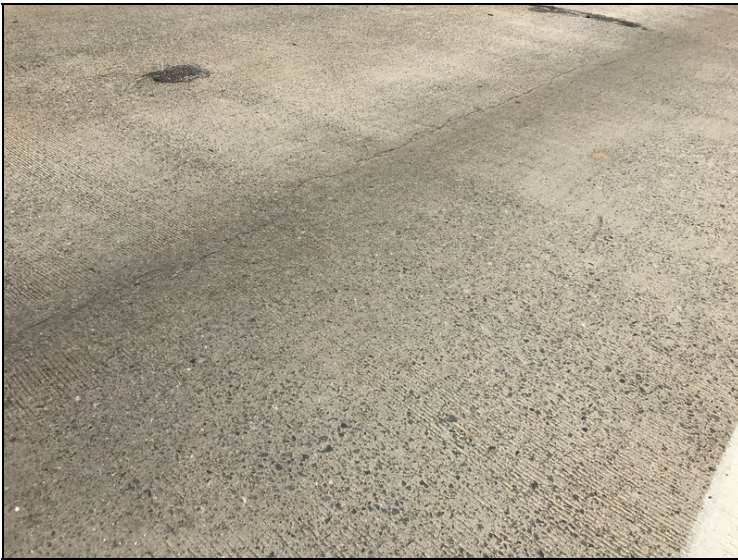
Span 3 unsealed crack at centerline
