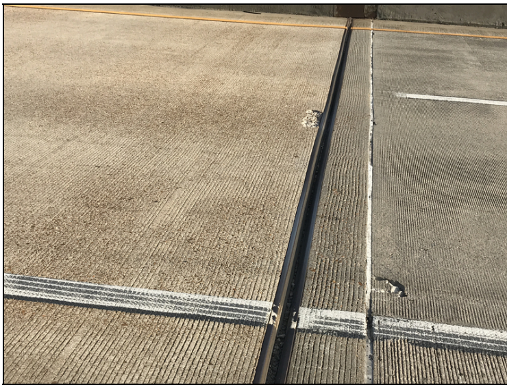
Span 4 at bent 5 small spall
