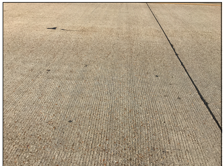
Span 3 unsealed deck cracks up to 0.025"
