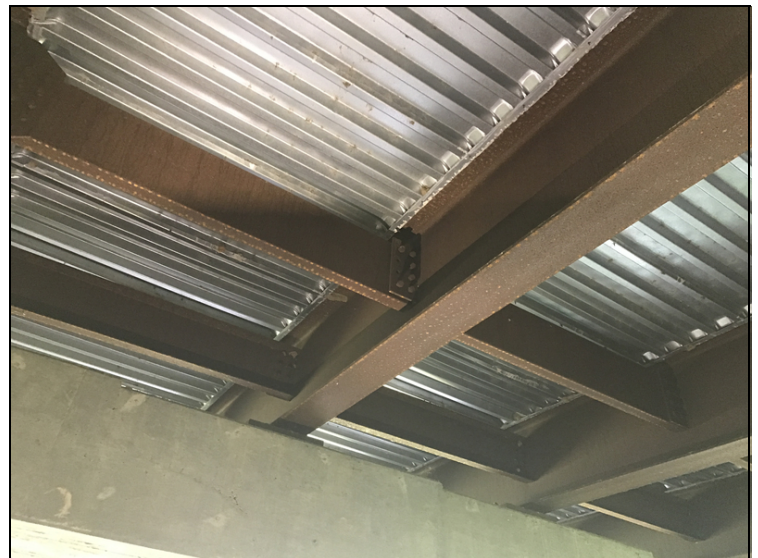
Span 5 beam 4 right side first diaphragm, 6 bolts loose. 2 missing
