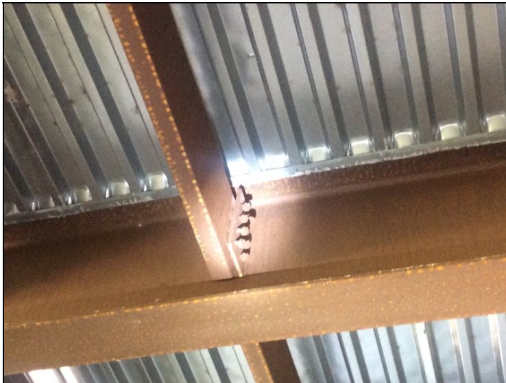
Span 5 beam 4 right side first diaphragm, bolts loose.
