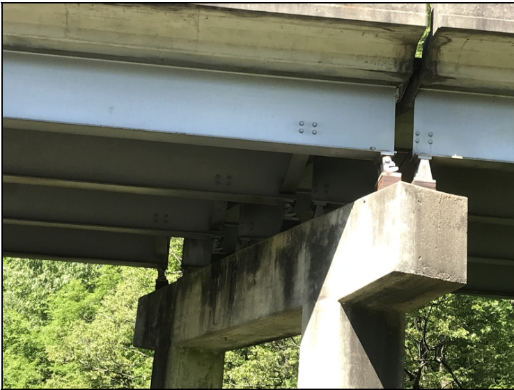
Span 2, bent 3: all bearings are rotated fully to their max inwards.
