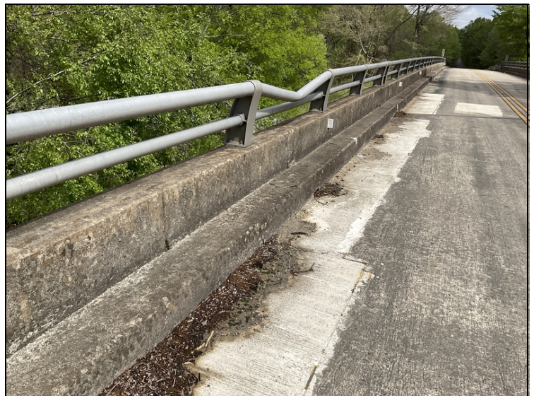
Span 3, left metal guard rail damaged.
