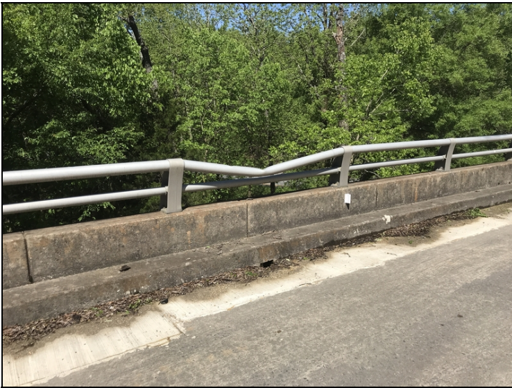
Span 3, left metal guard rail damaged.
