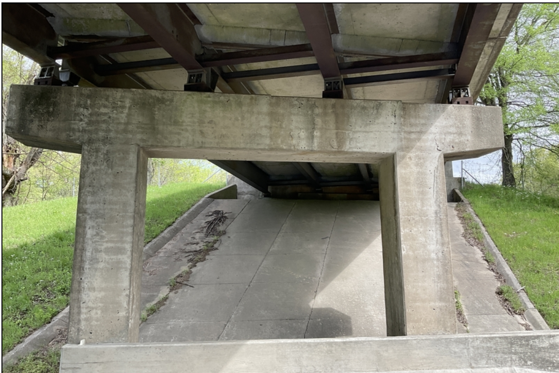
Bent 6 delams on back face
