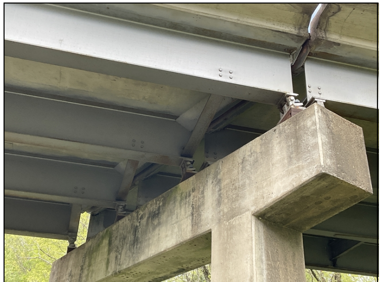
Bearings are fully rotate at bent 3 on span 2 and joint is open up to 4 ½ inches.
