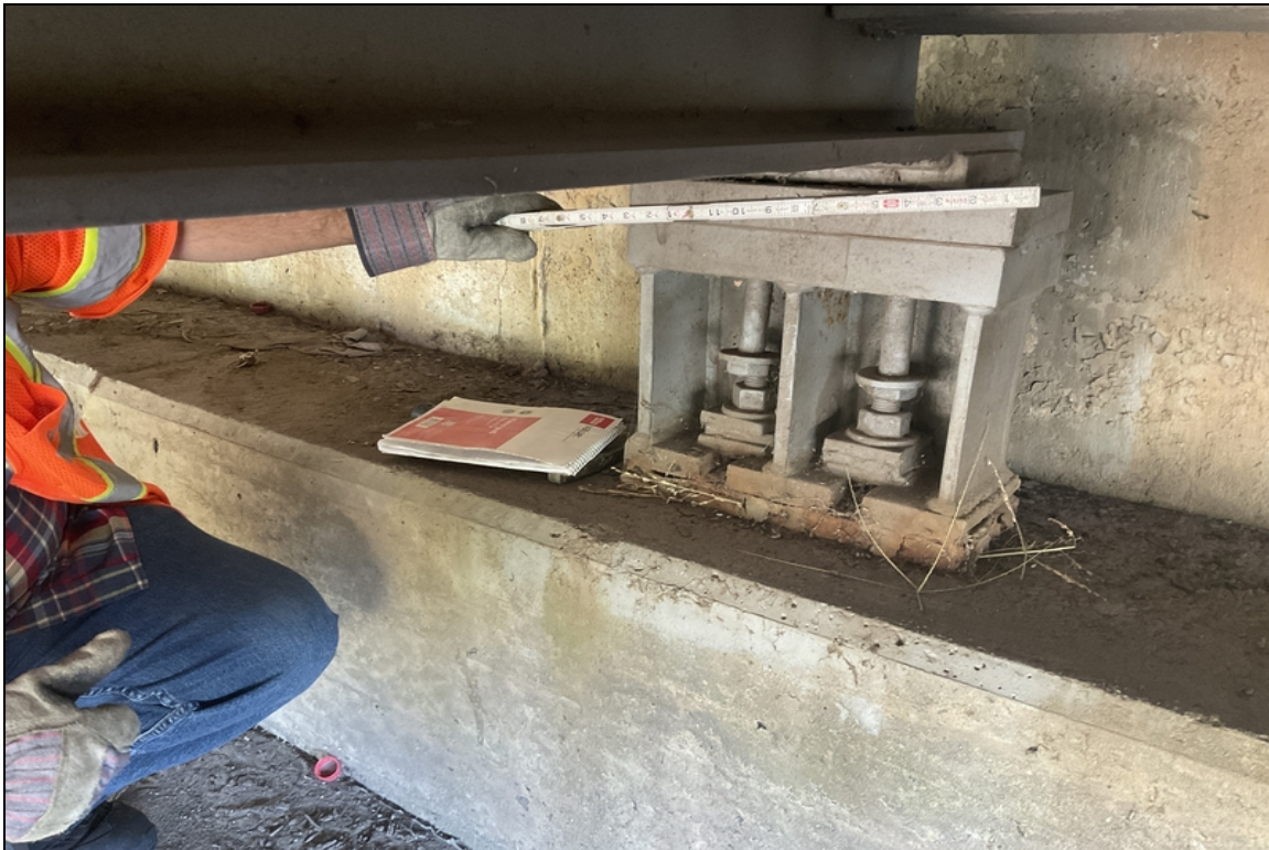
Bent 5 bearing 4 has 2 missing anchor nuts
