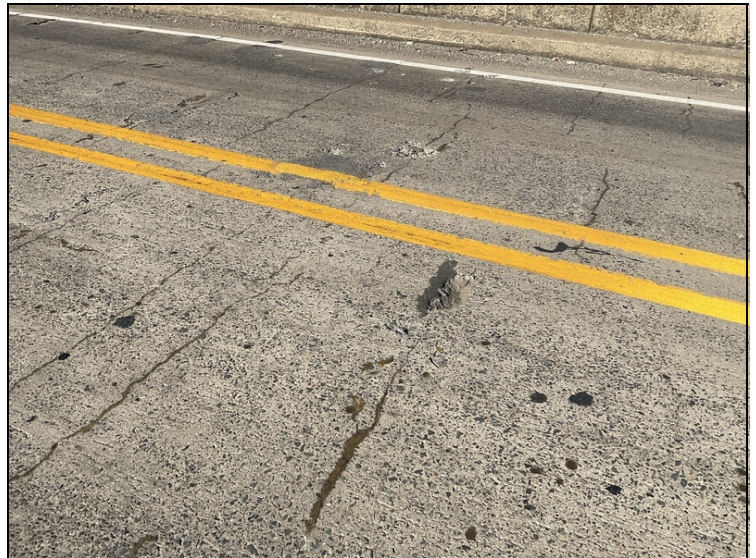
Span 3 spalls and spalls filled with asphalt
