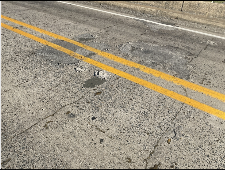
Span 2 spalls and spalls filled with asphalt
