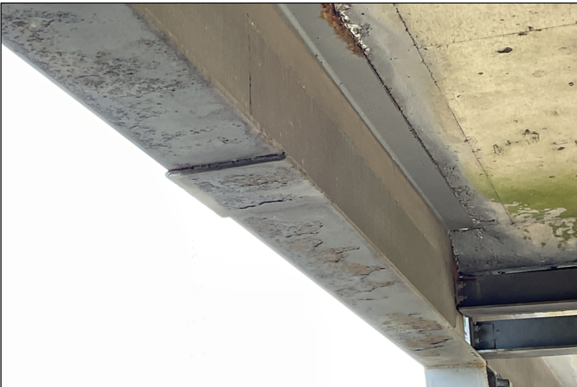
Span 1 beam 1 repair, weld is cracked on added bottom plate. No change since last inspection.
