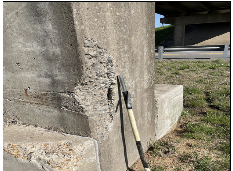
Bent 3 column 2 large spall
