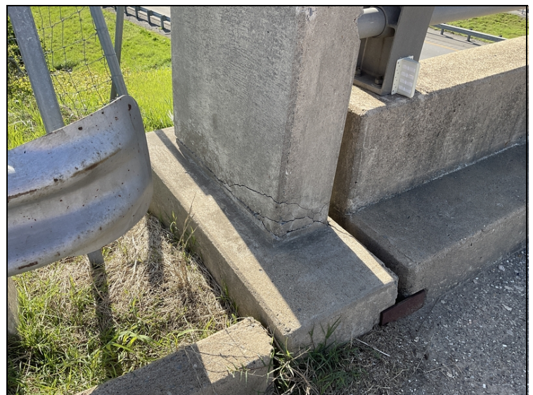
Bent 5 right end post cracked at bottom.
