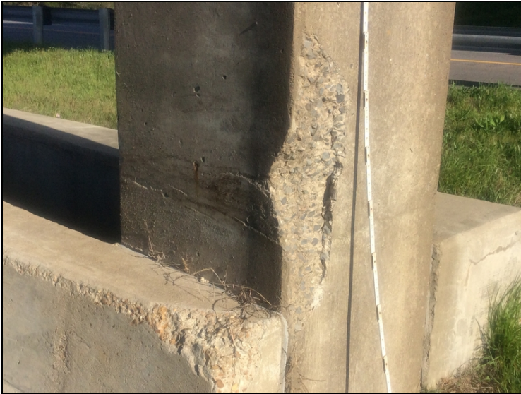
Bent 3 column 2 has spall due to traffic impact.
