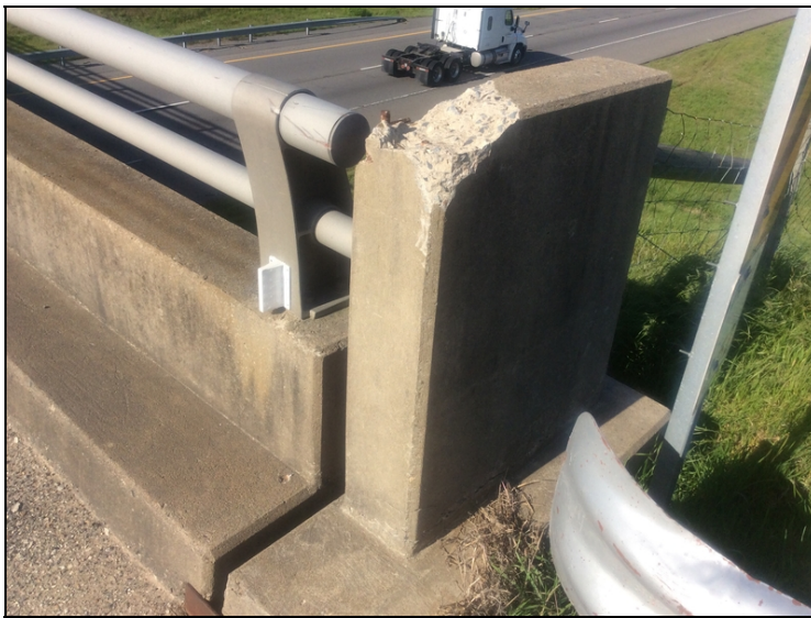
Left end post at bent 5 has spall with exposed rebar and is cracked at the bottom. Common left end post bent 1.
