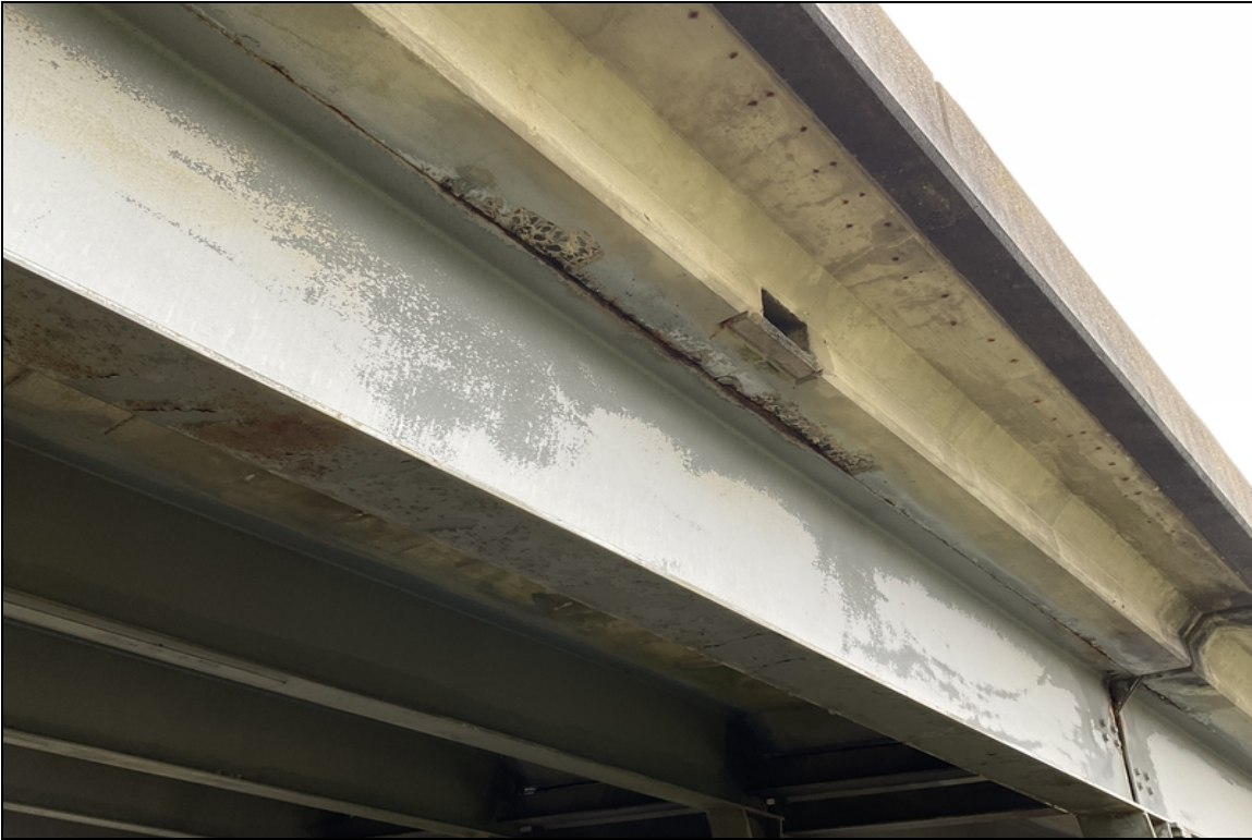
Span 1 small spalls along top flange
