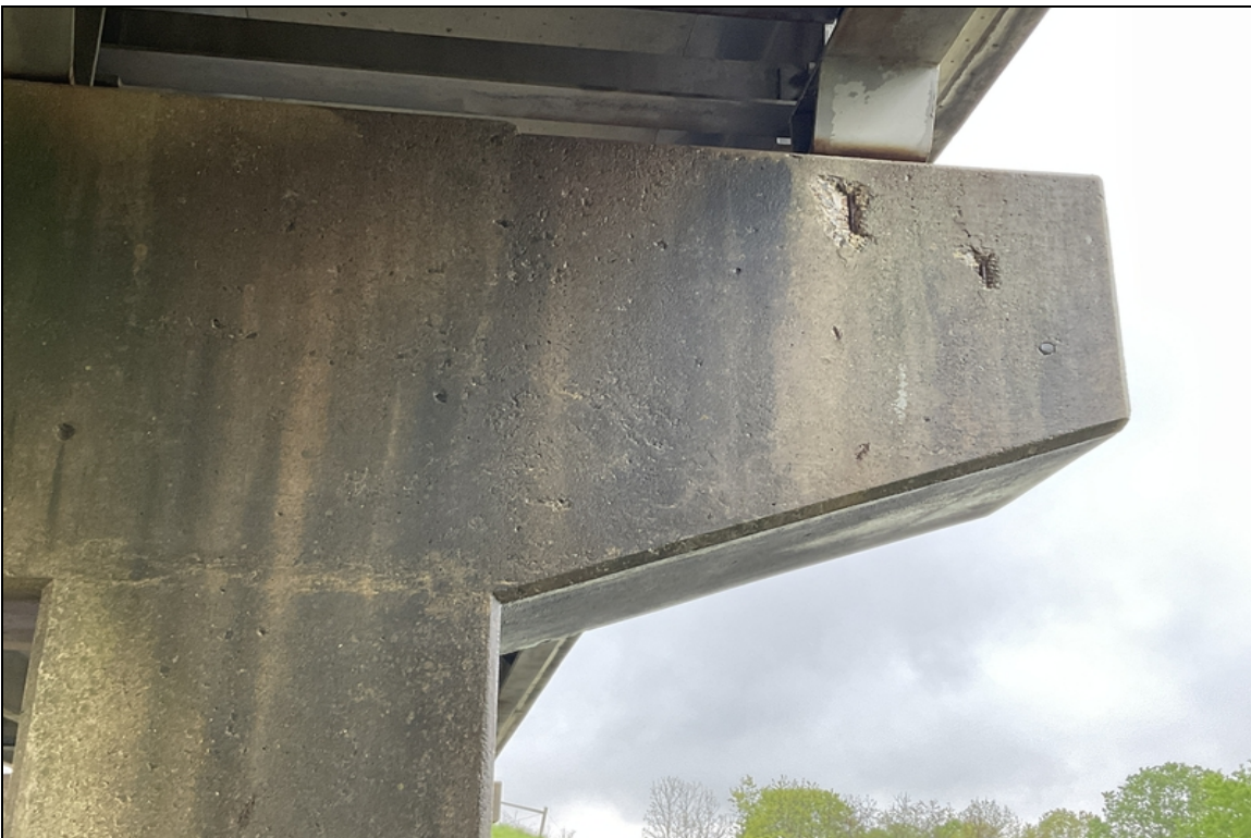
Bent 4 exposed rebar on ahead face
