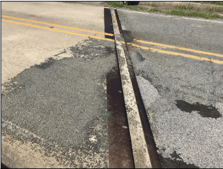
Bent 5: top of back wall is spalled
