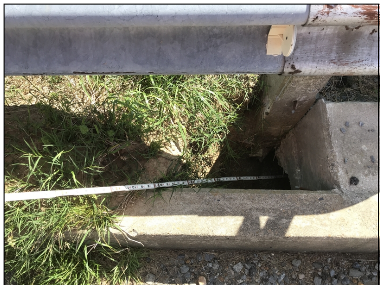
North abutment right approach gutter void.
