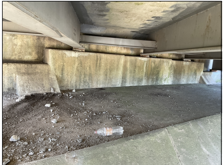
Most of the broken concrete has been removed
