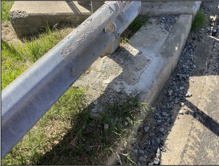
State forces have poured concrete in void
