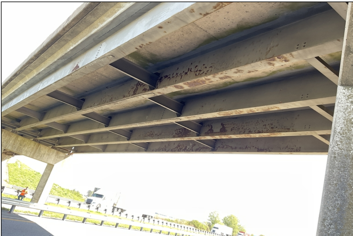
Span 2 typical paint condition
