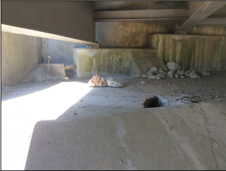
Broken pieces of concrete at bent 5, south abutment.
