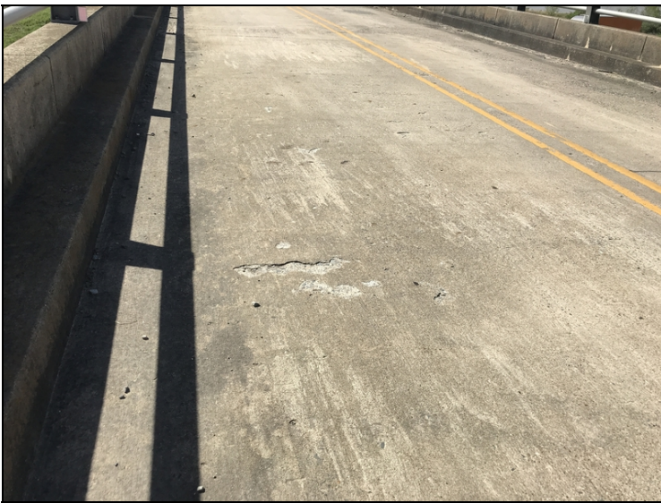
Span 3: deck spalls
