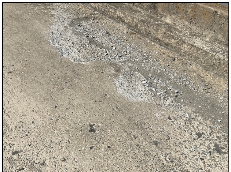
Span 3 spalls in left lane
