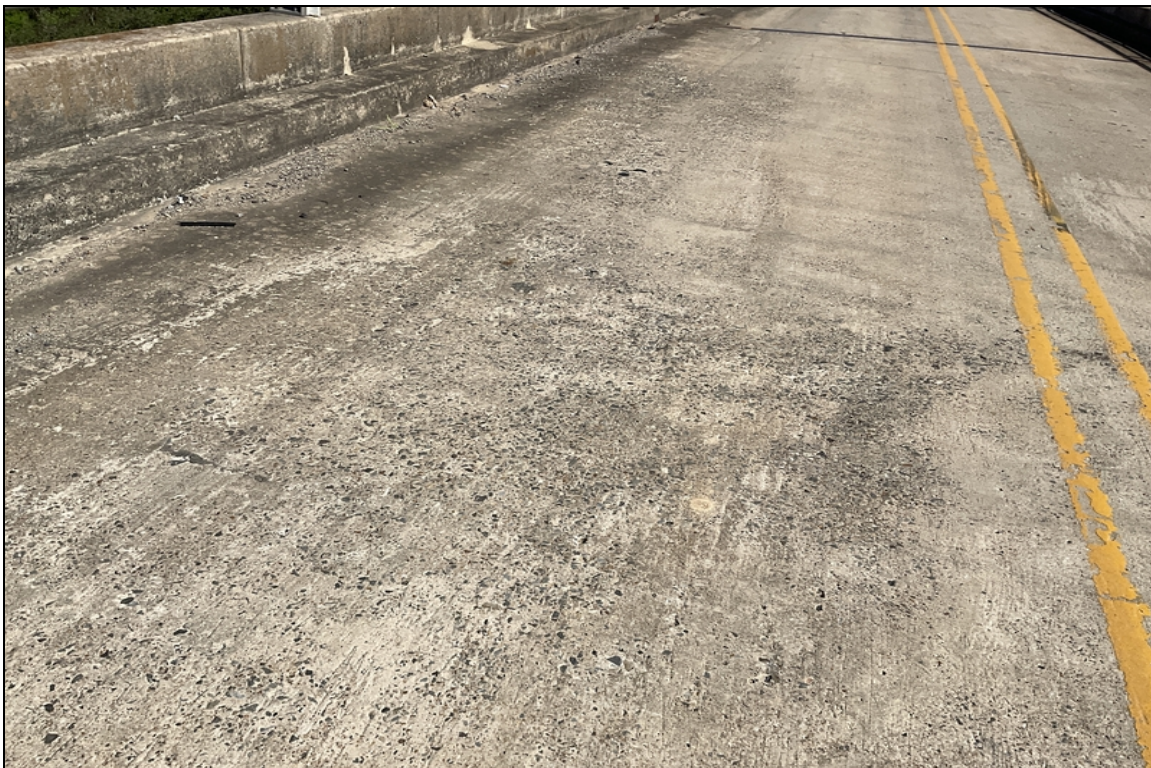
Span 3 abrasion/wear in left lane
