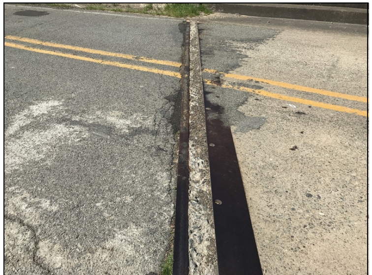
Bent 1 top of back wall has spalled
