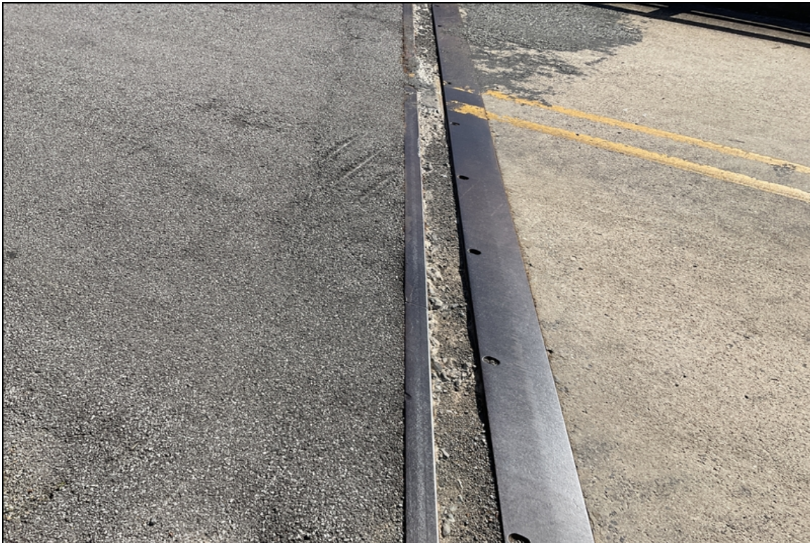
Bent 5 top of backwall is spalled
