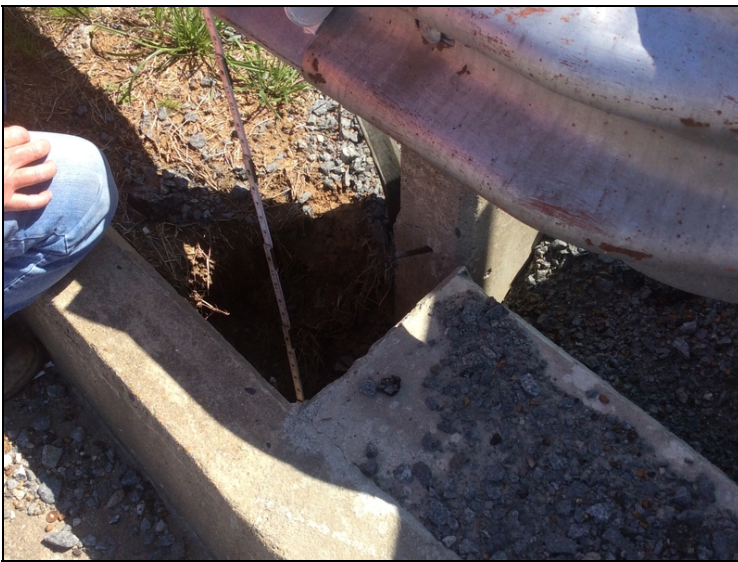
North abutment right approach gutter void.
