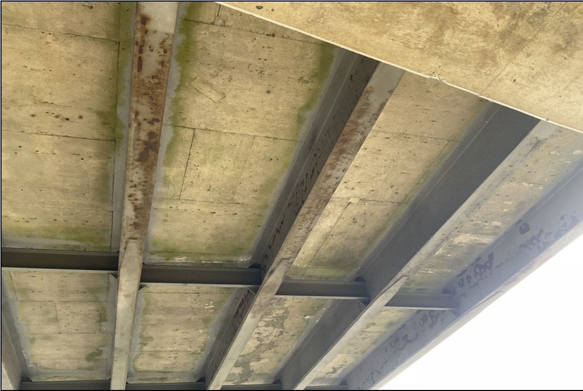
Protective coatings span Span 2 scattered areas of surface rust to webs and bottom flanges
