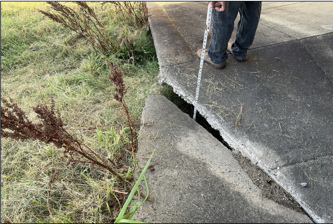
Void under slope pavement at bent 1
