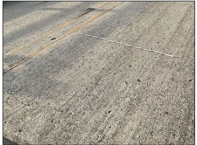
Deck cracks in span 4
