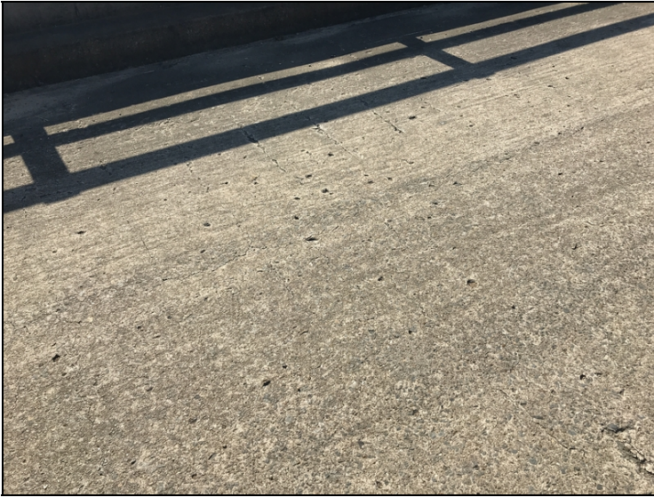
Span 4 transverse and longitudinal cracks up to 0.040"
