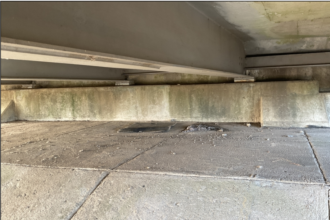
Bearings at bent 1 typical condition of most
