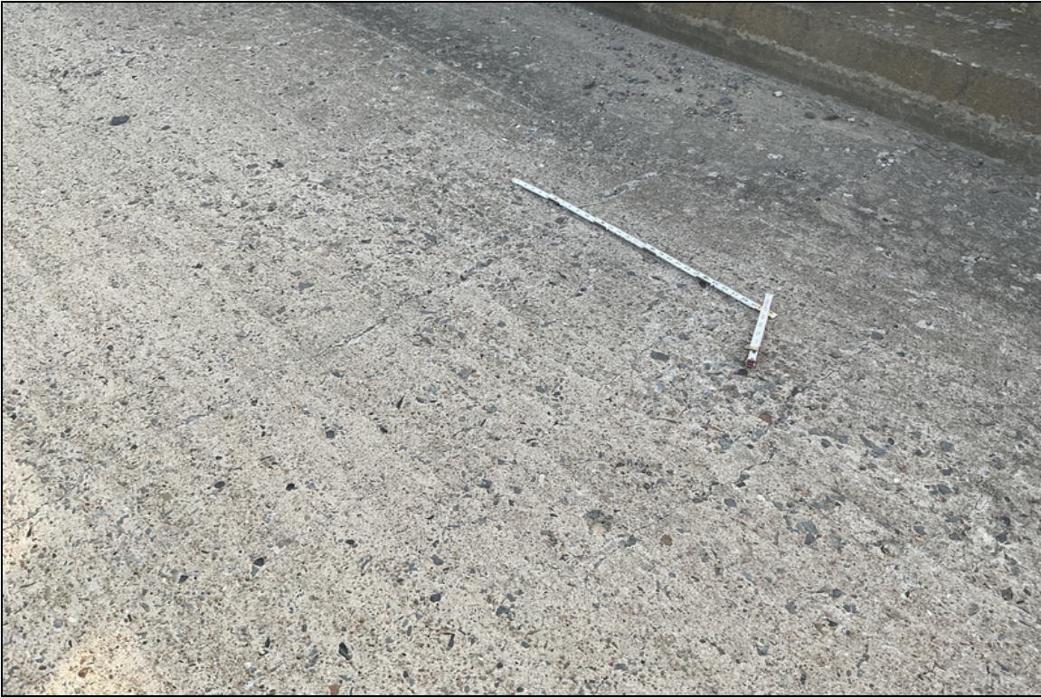
Large cracks in span 2
