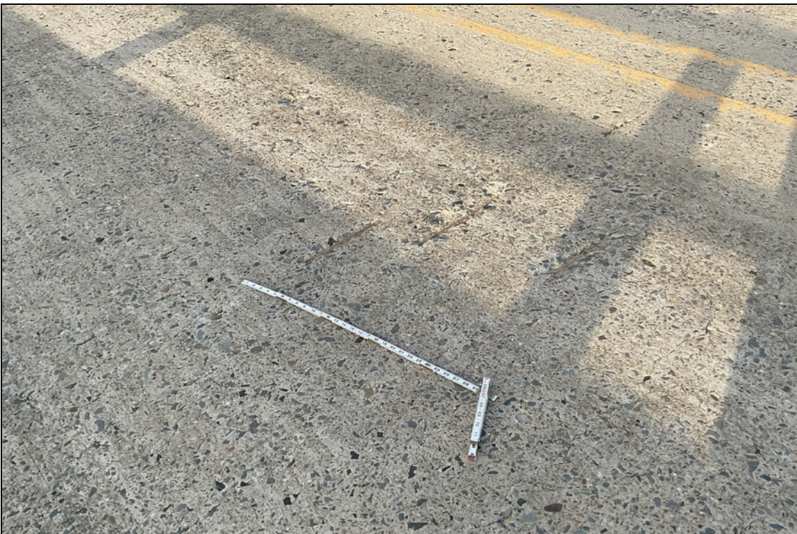
Rebar exposed in span 2
