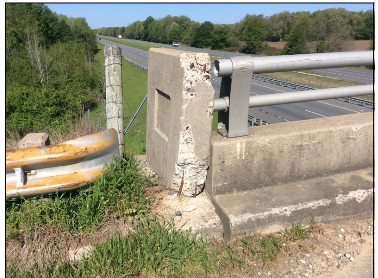
Left end post span 1 has spalls with exposed rebar.
