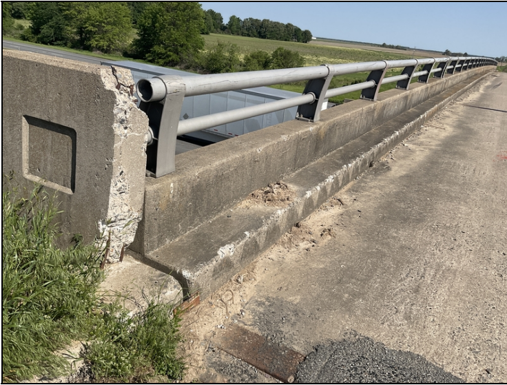
Left concrete end post at South abutment and both Bridge rails on spans 1 and 2 have traffic damage.
