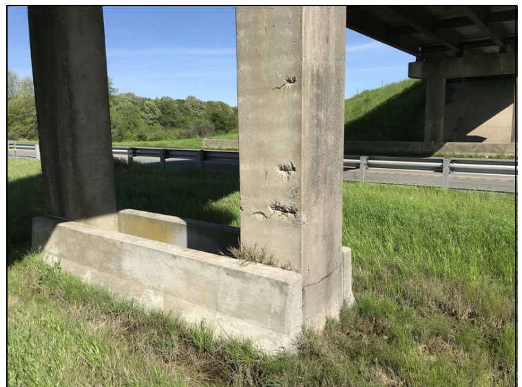
Bent 3, right column has spalls with exposed rebar
