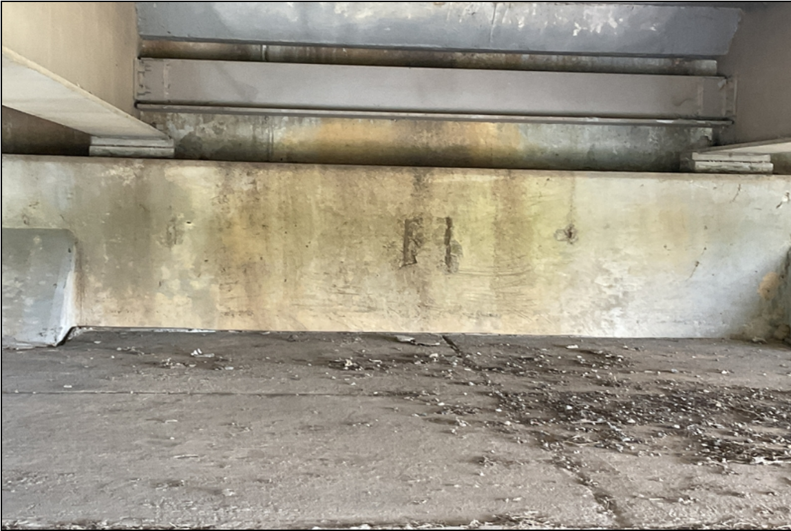
Bent 5 exposed rebar
