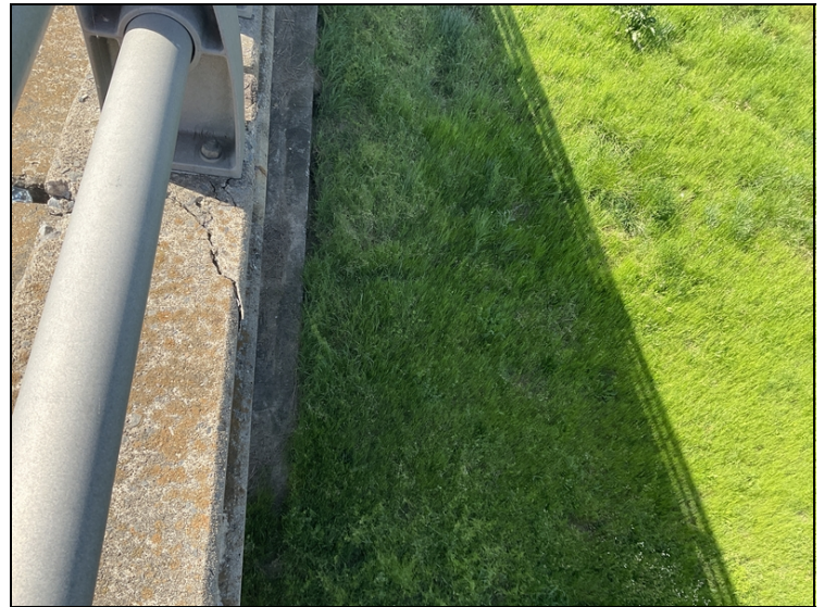
Span 2 at bent 2 left rail is spalled from traffic impact
