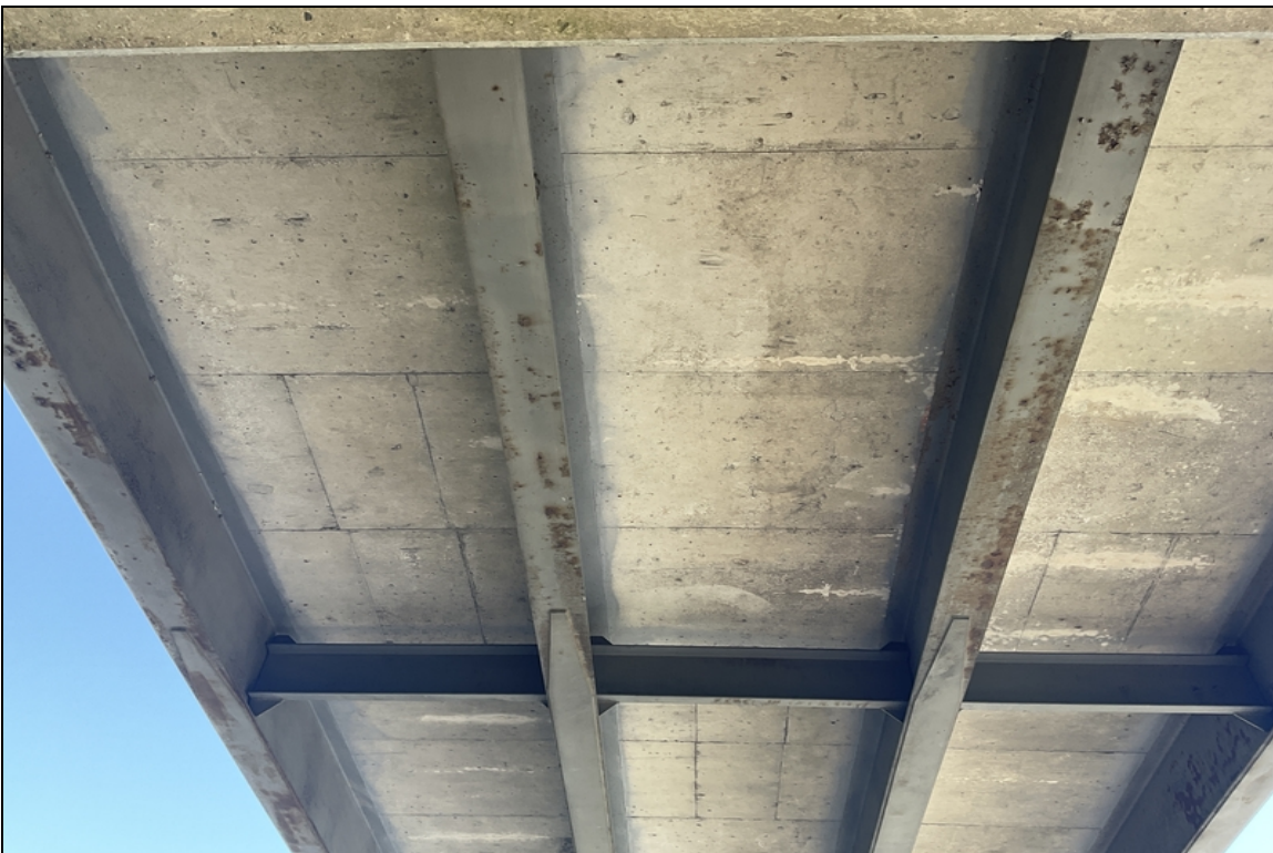
Span 2 freckled rust on bottom flanges
