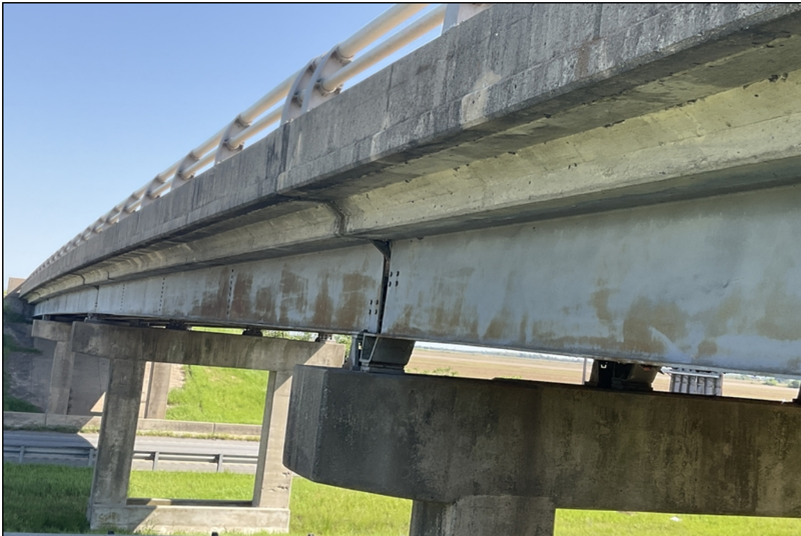
Typical paint condition
