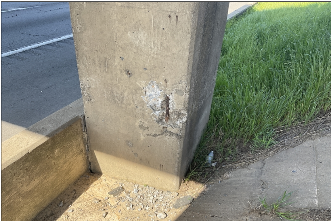
Bent 4 Left column has spall with exposed rebar
