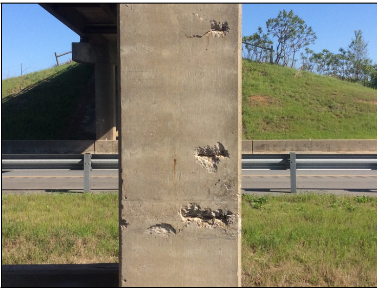
Bent 3 right column has spalls with exposed rebar.
