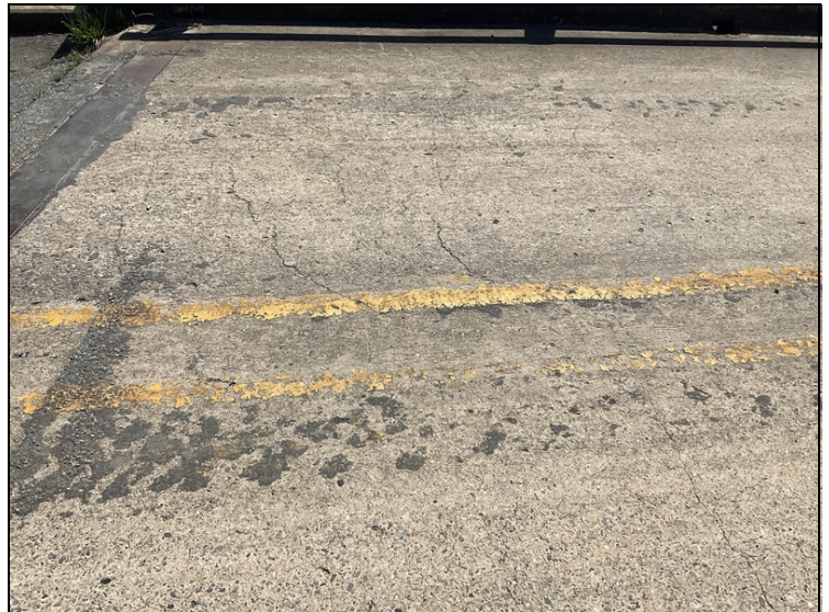
Span 4 deck cracking up to .040"
