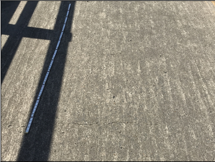
Deck has unsealed cracks up to 0.040 inch wide.
