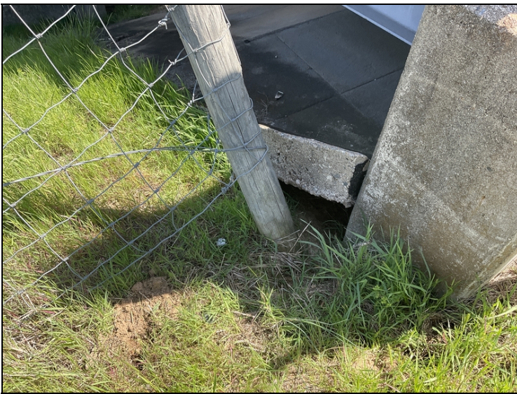
Void under slope paving on south abutment
