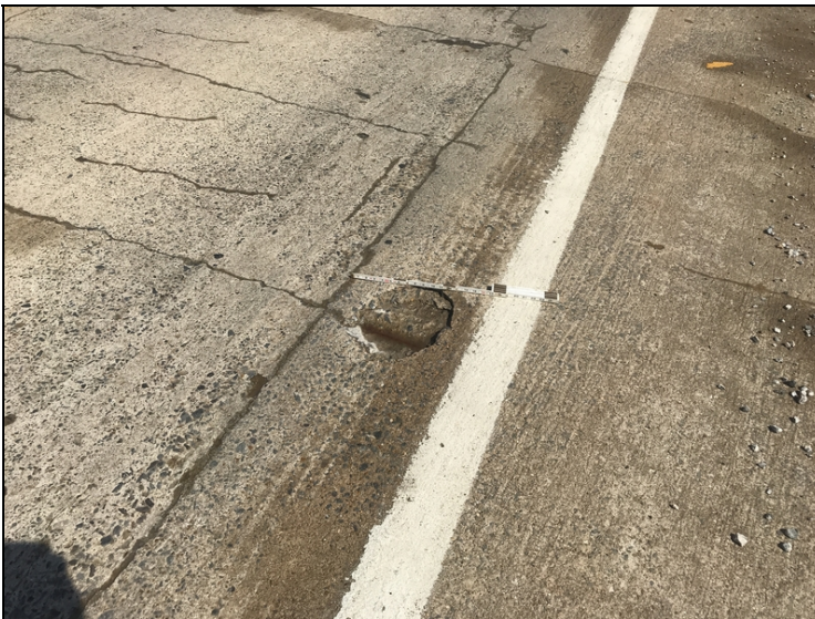
Span 6 with an open spall in northbound lane
