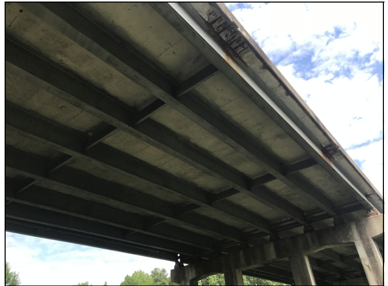
Spalls with exposed rebar on the right side of span
