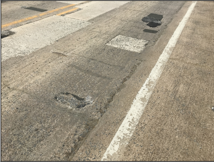
Span 1 spalls and spall# filled with asphalt
