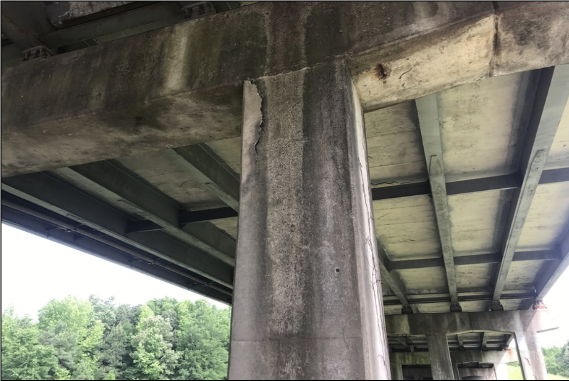
Bent 3 column 3 large delam
