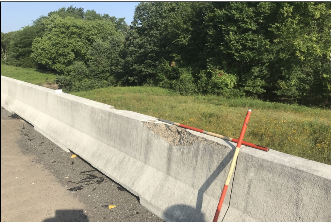
Damage to the right barrier wall in span 2.
