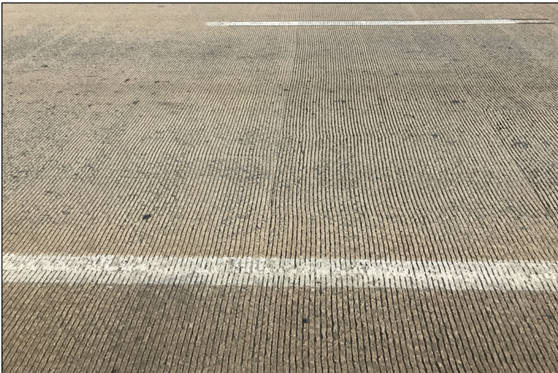
Span 1 unsealed transverse crack
