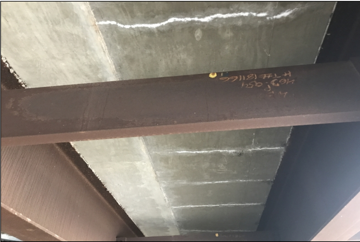
Efflorescence between beams 4&5
