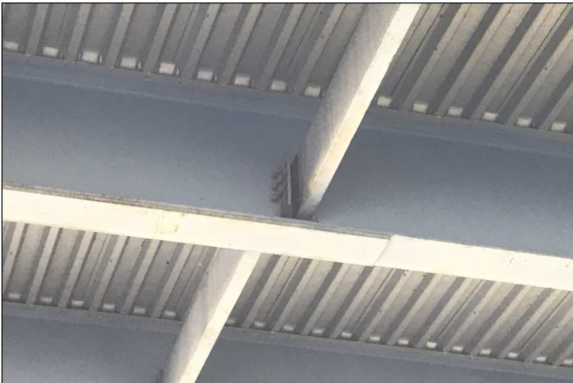
Span 8, girder 2, 1st diaphragm: all bolts are loose with no nuts connected
