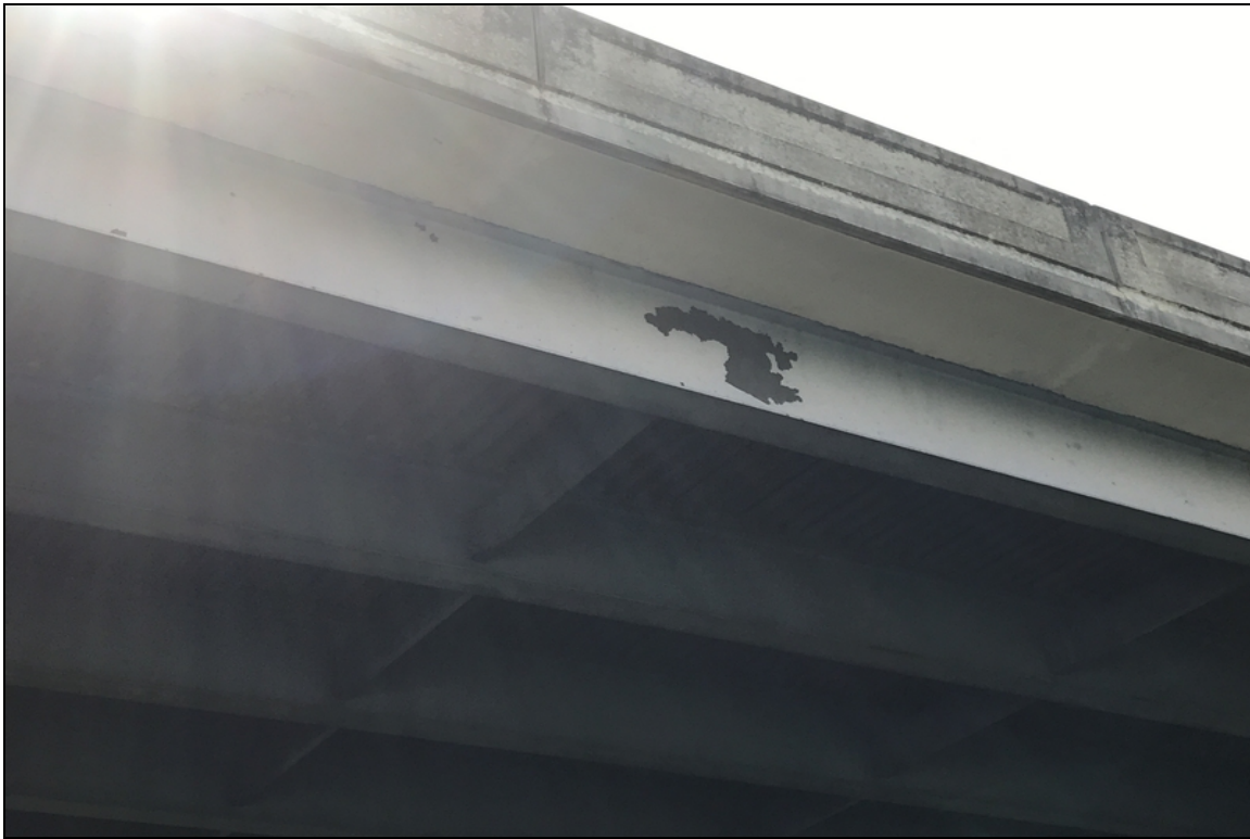
Span 10, girder 1: outside of beam with flaking paint. Multiple locations in similar condition
