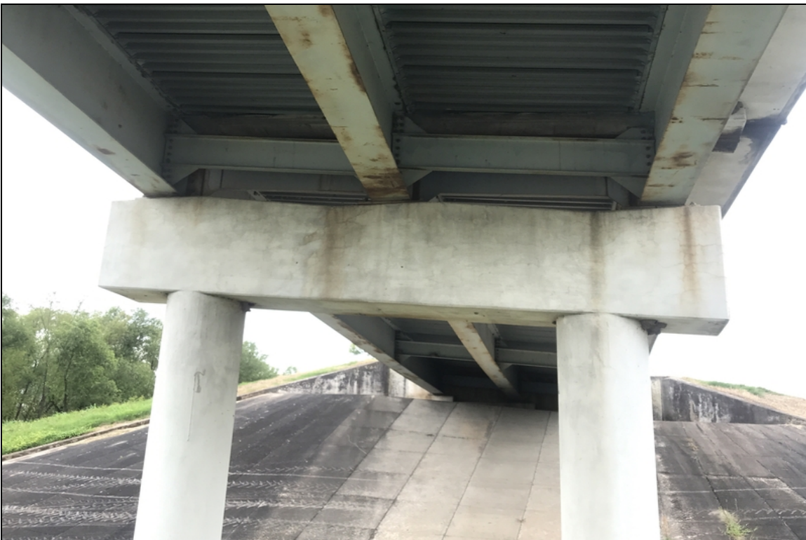
Bent 2 ahead: entire length of cap is map cracked
