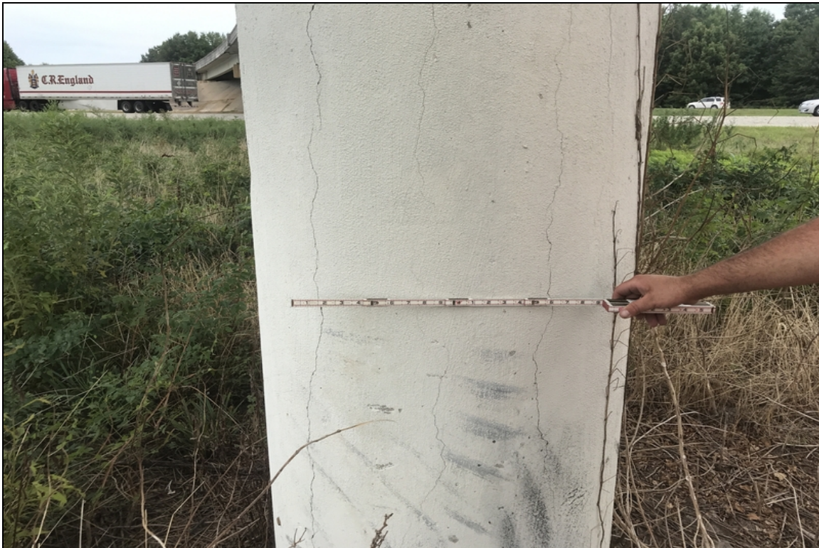
Bent 5, column 1: numerous full height vertical cracks on 6" centers. All columns on this structure are in similar condition
