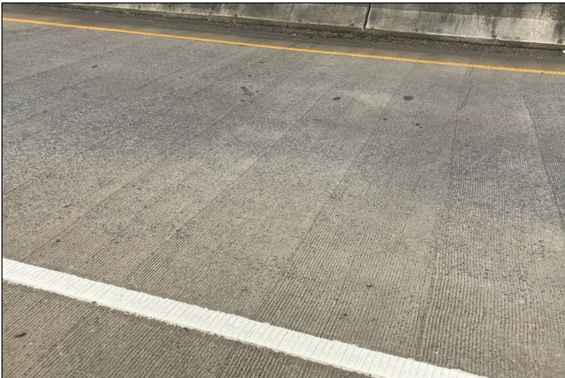
Span 4: transverse cracks common at this span. (3' spacing)
