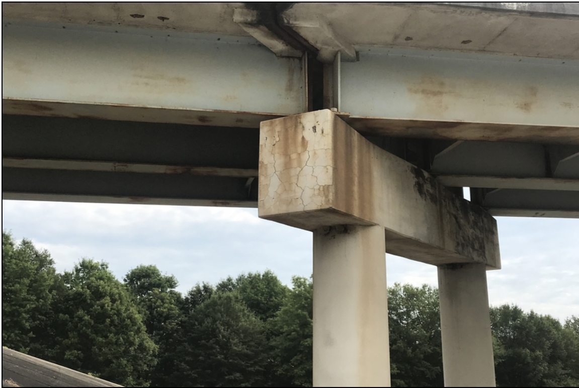
Bent 7, left end of cap is map cracked.
