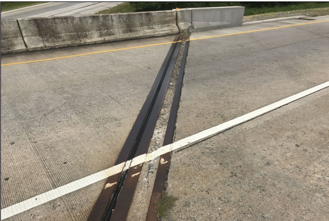
Bent 8: back wall spalled
