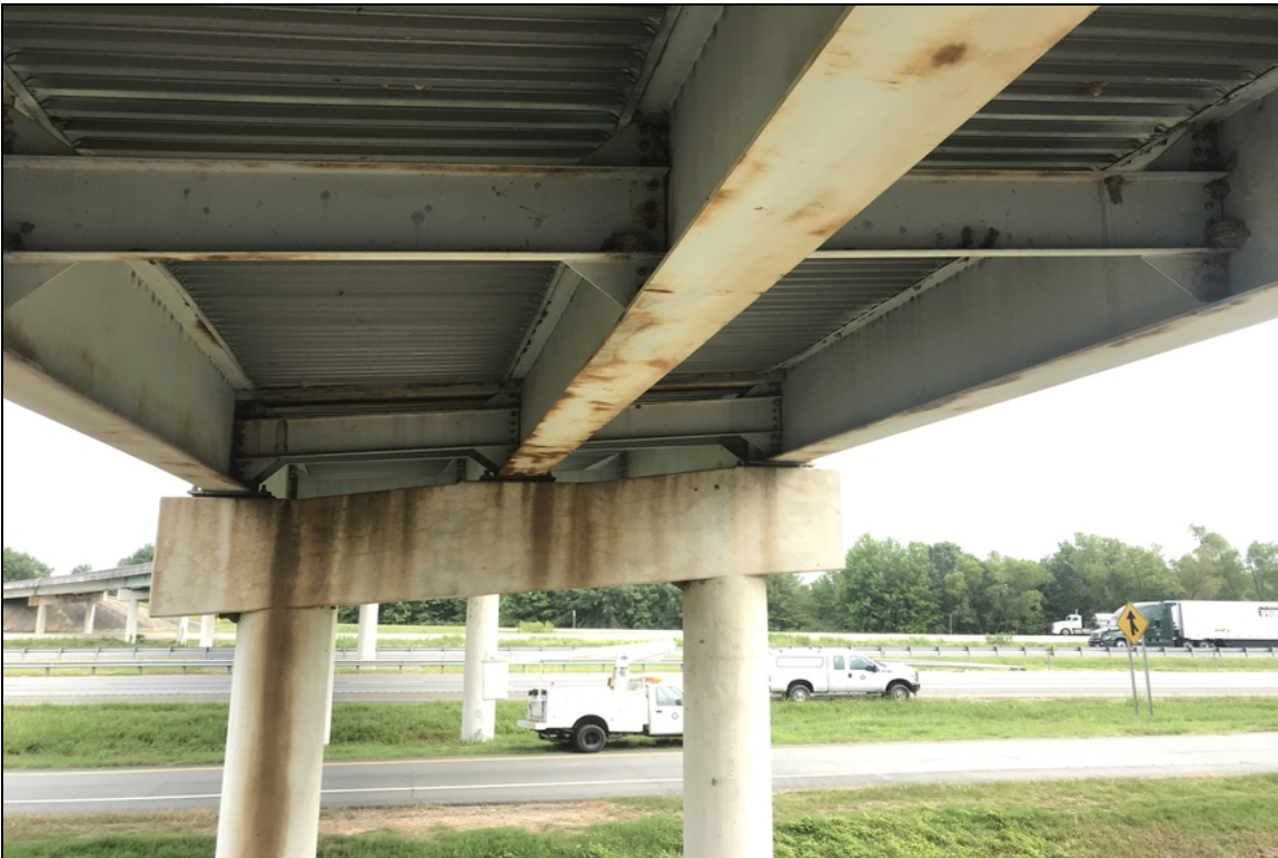
Span 1: common paint condition of girders on this structure
