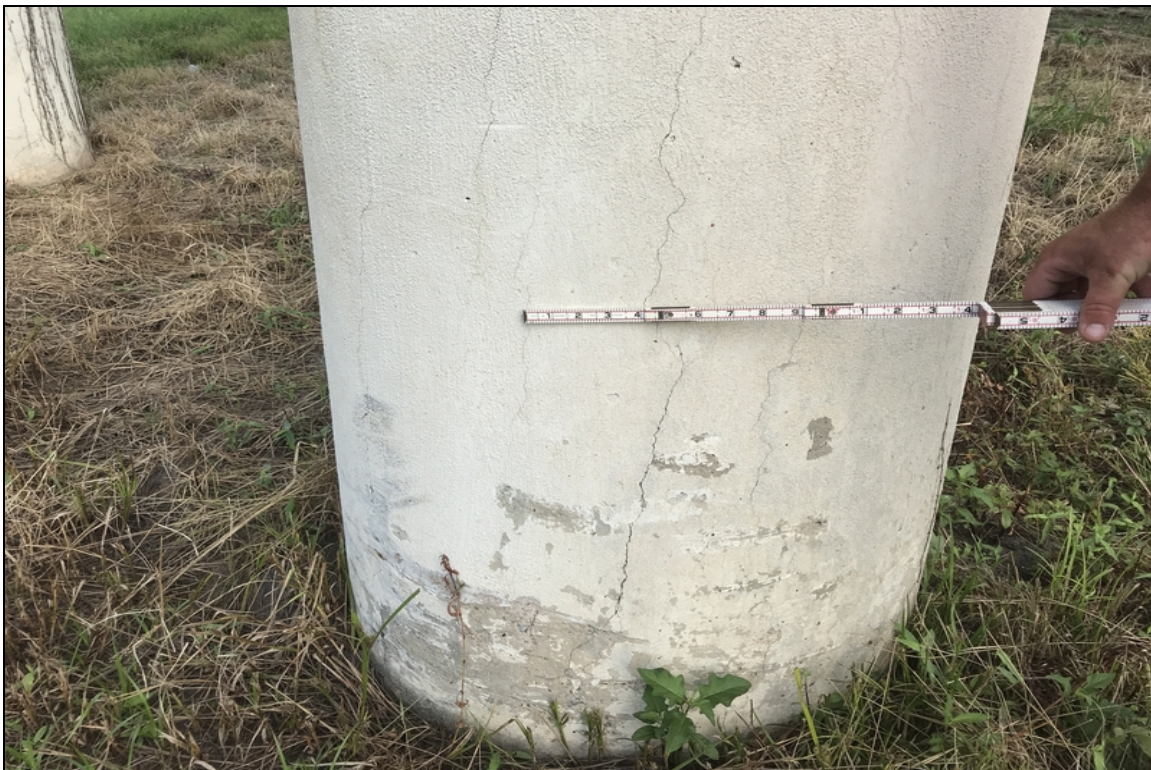
Bent 3, column 1: the column has numerous full height vertical cracks on 6" centers. All columns are in similar condition
