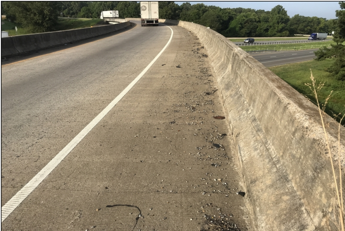
A large amount of debris accumulating on deck
