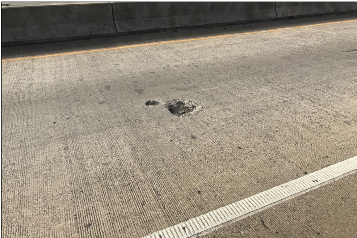
Span 4: spall in the deck surface
