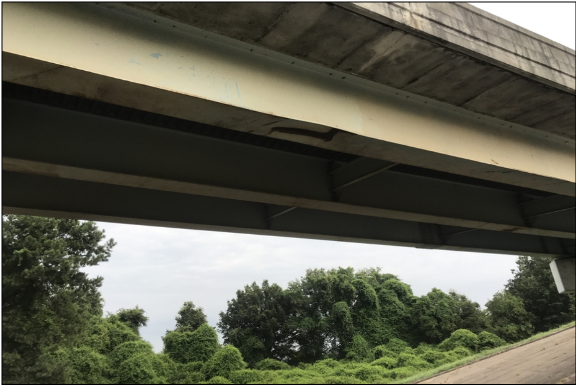
Span 4, girder 3: damage due to vehicle impact to the lower flange.
