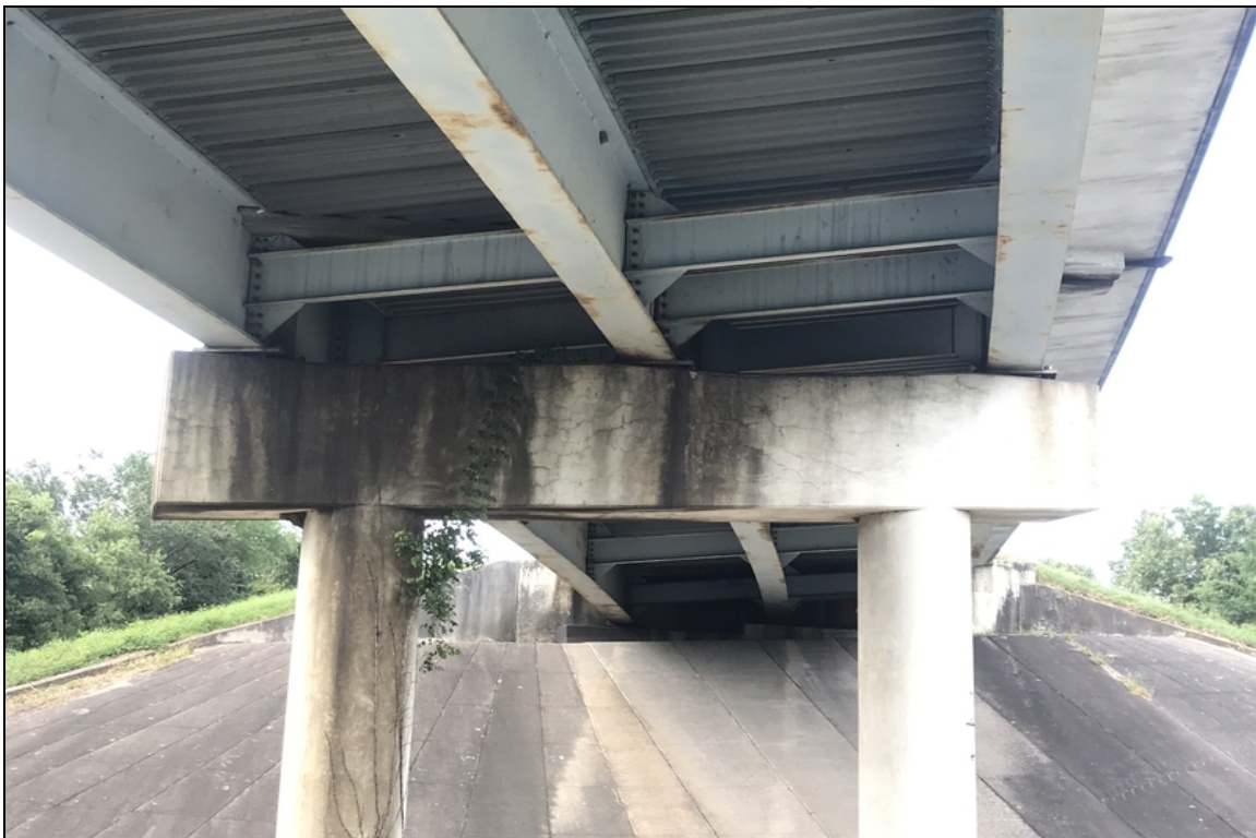
Ahead side of bent 2: the entire face of cap is map cracked
