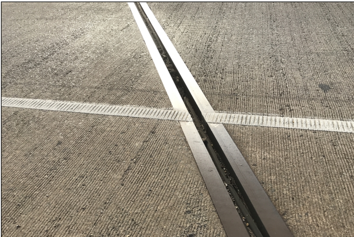
Bent 2: left side of the compression joint has lost bond allowing water to flow through
