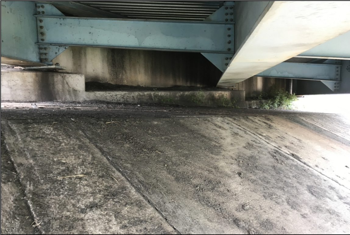
Bent 6: the beam seat has map cracking through the entire face. Also, the beam seat has a large amount of dirt and vegetation a top of it
