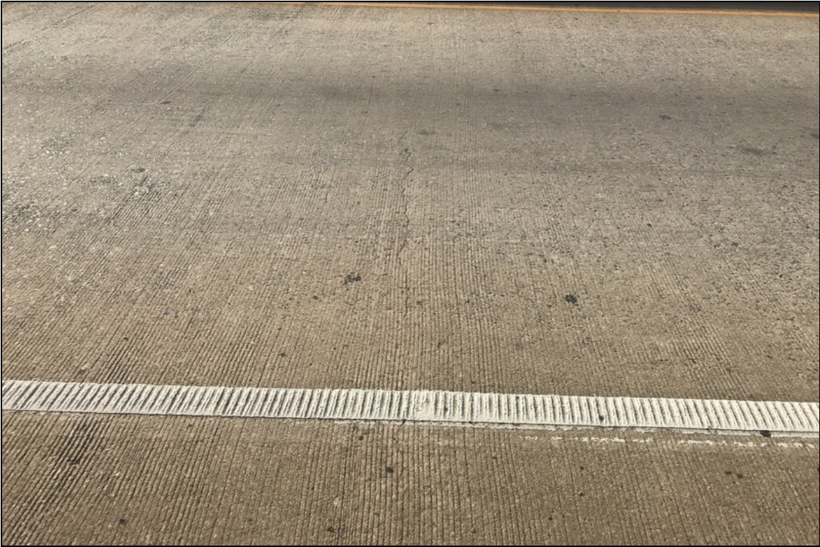
Span 5: large transverse crack
