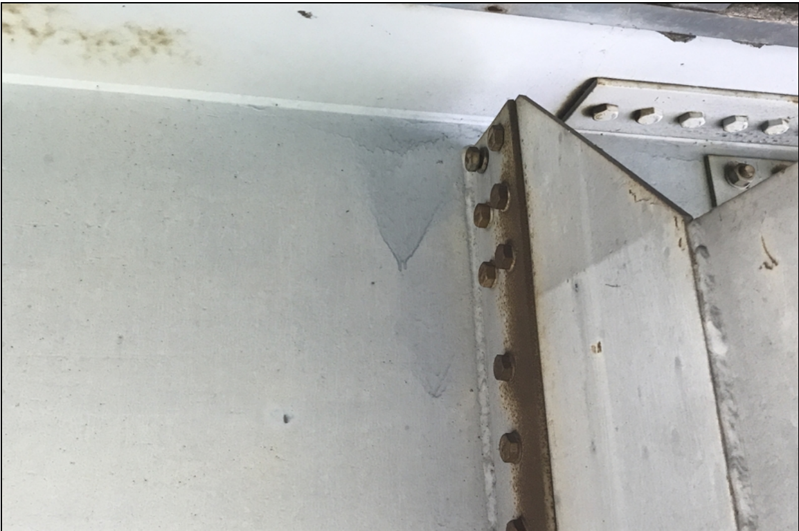
Span 4, girder 2, 2nd dia. Loose bolt at the top of diaphragm
