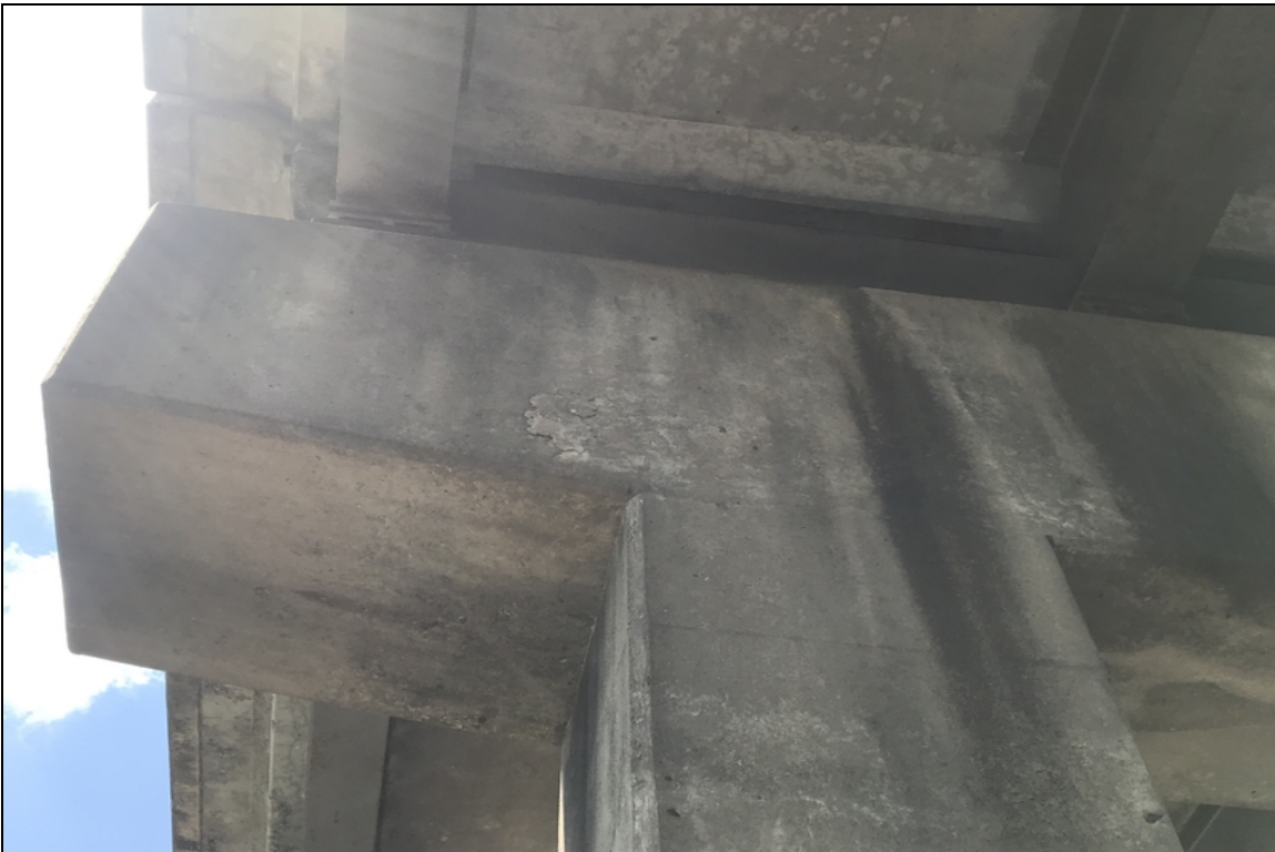
Bent 2 cap ahead has delam.
