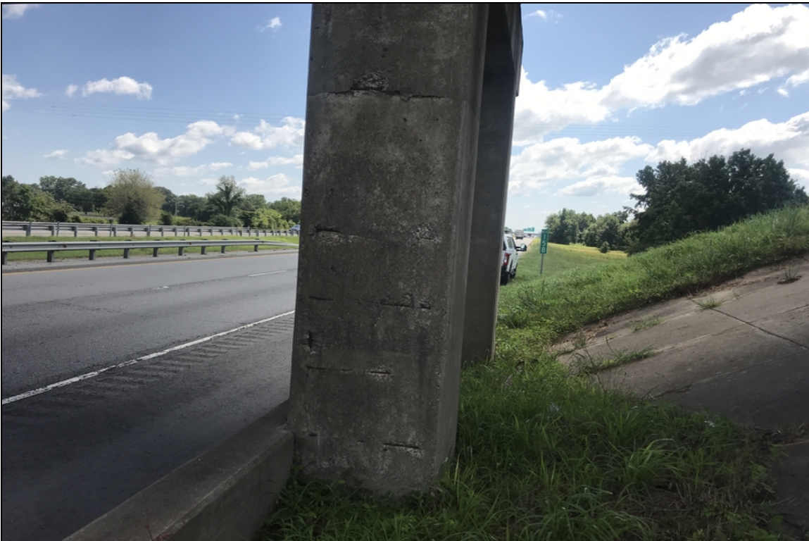
Bent 2 column 1 has spalls with exposed rebar. Common column 2.
