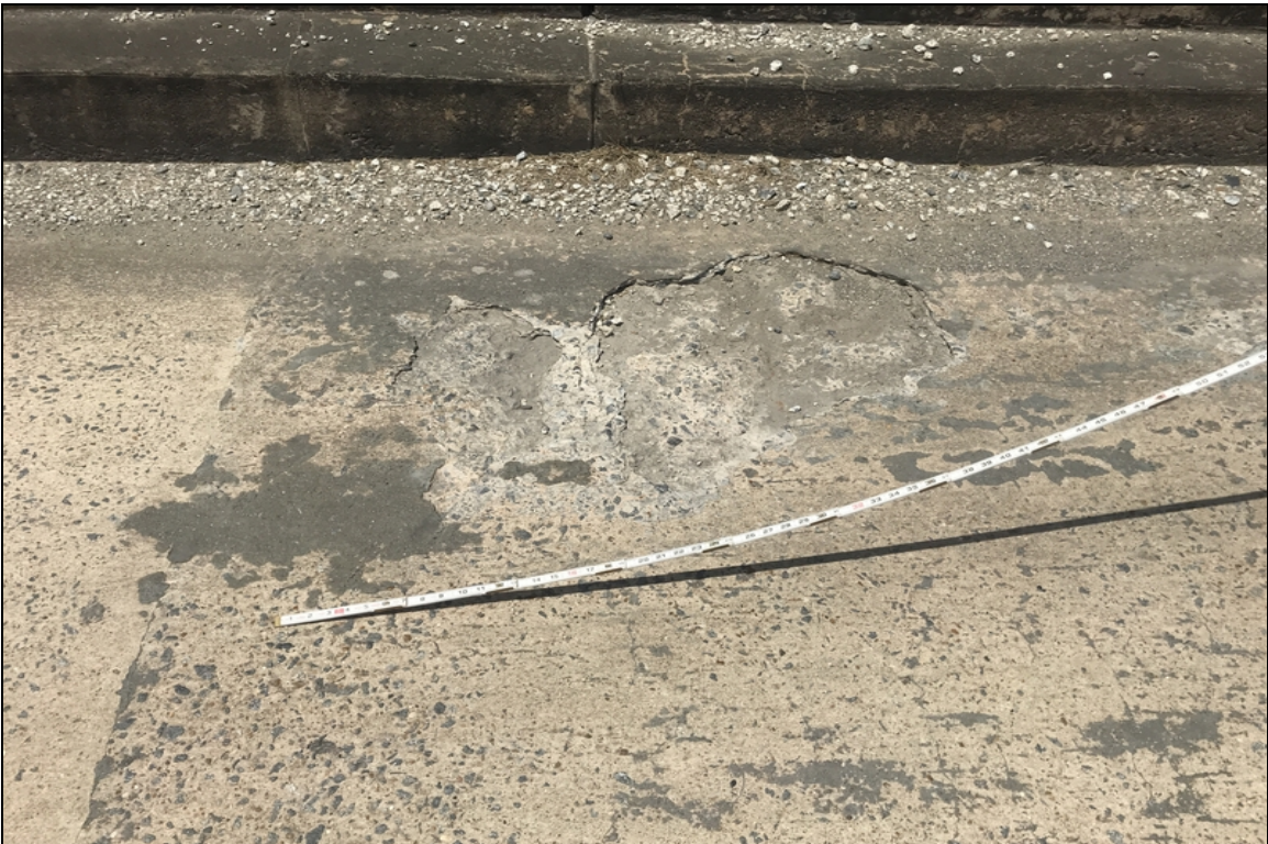
Deck span 2 has spall.
