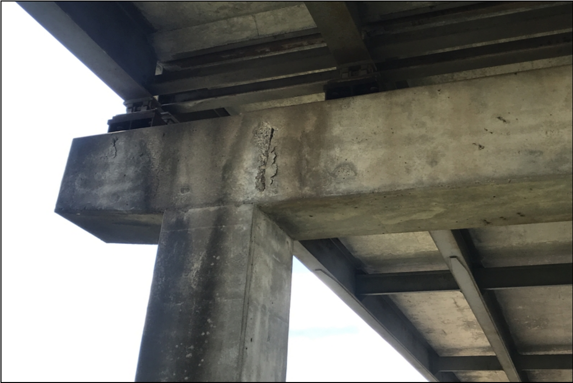
Bent 3 cap ahead has spall with exposed rebar.
