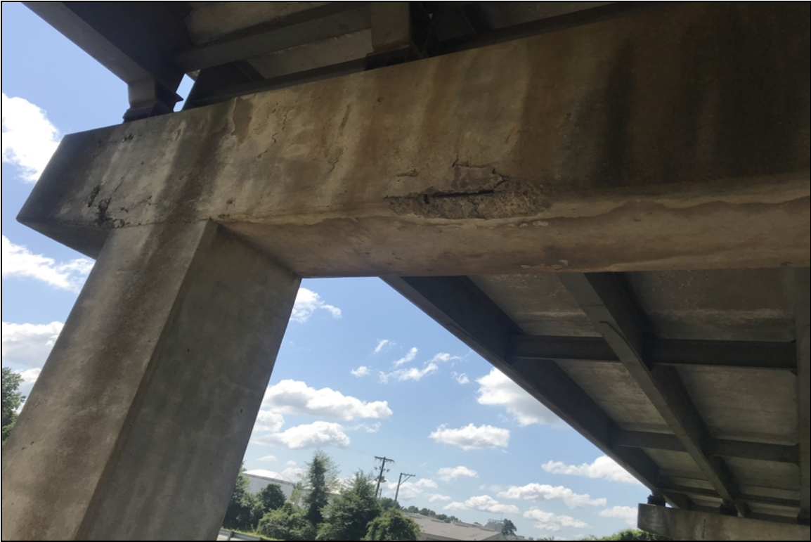
Bent 4 cap ahead has spalls with exposed rebar.
