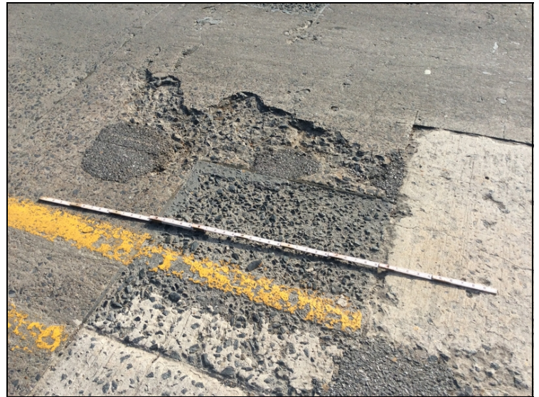
Span 2 spalls with exposed rebar.
