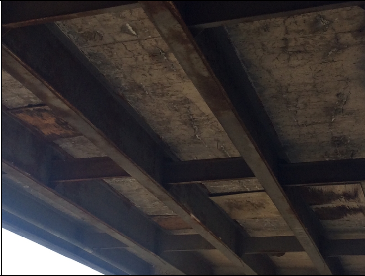
Span 3 soffit cracks with effloresces and rust stains.
