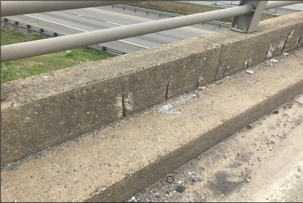
Spalls with exposed rebar, Span 4 right bridge rail
