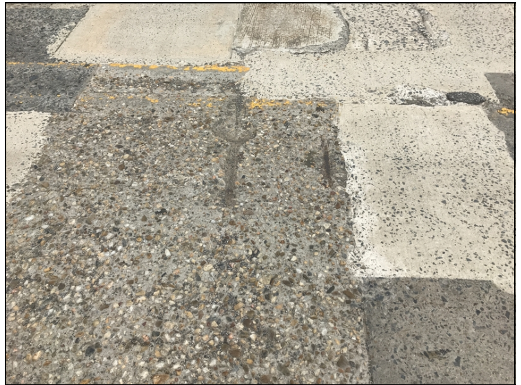
Span 3 spalls with exposed rebar
