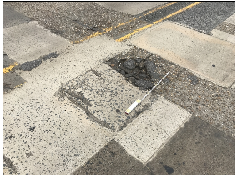
Span 3: large open spall with exposed rebar.
