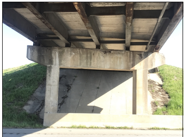
Bent 4, backside of cap is spalled and delaminated at the top.
