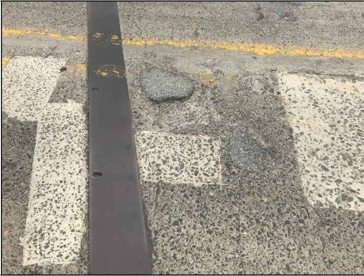
Span 3 spall with exposed rebar
