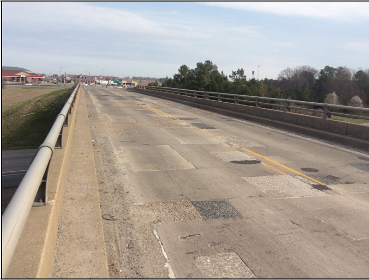
View of the deck with patched areas in all spans.
