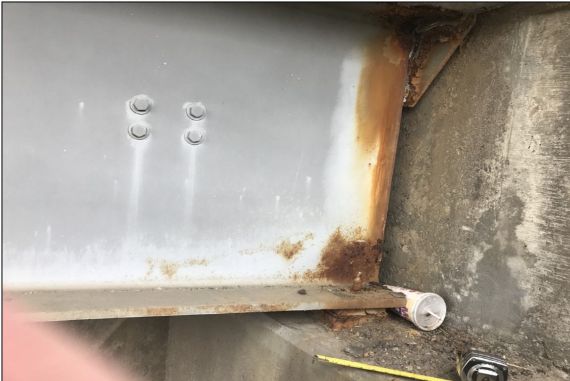
Bent 1 beam 1 typical beam end condition
