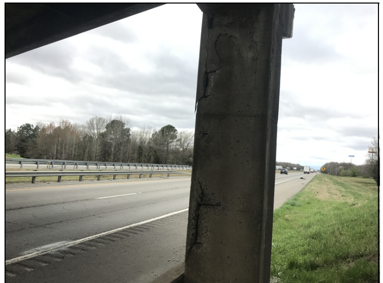
Bent 4 column 1 large spalls with exposed rebar
