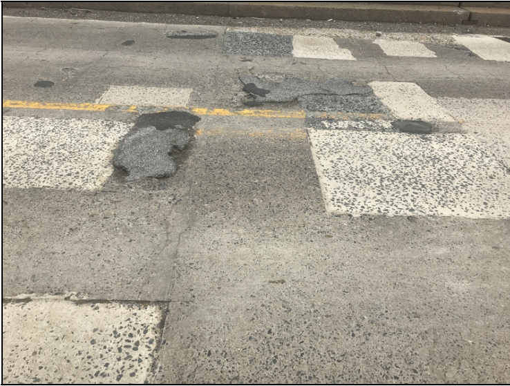
Span 2 spalls filled with asphalt
