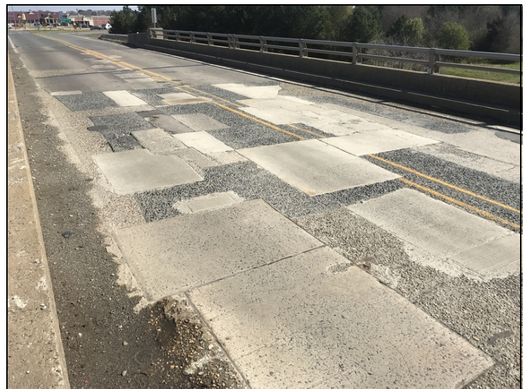
Span 3: majority of span is patched with most of the patches are beginning to deteriorate.
