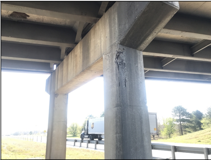
Bent 3, column 1: large spall with exposed rebar.
