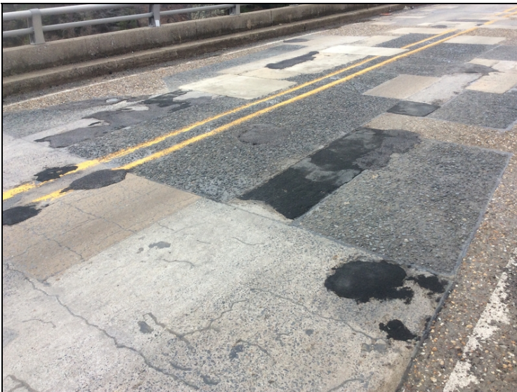
Span 3 spalls filled with asphalt.
