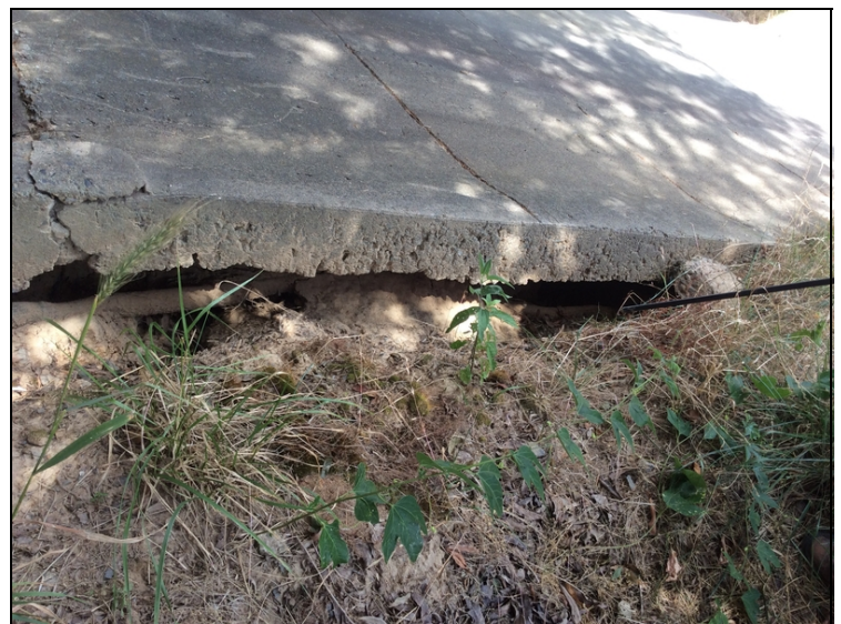
Large void under slope paving at bent 1.
