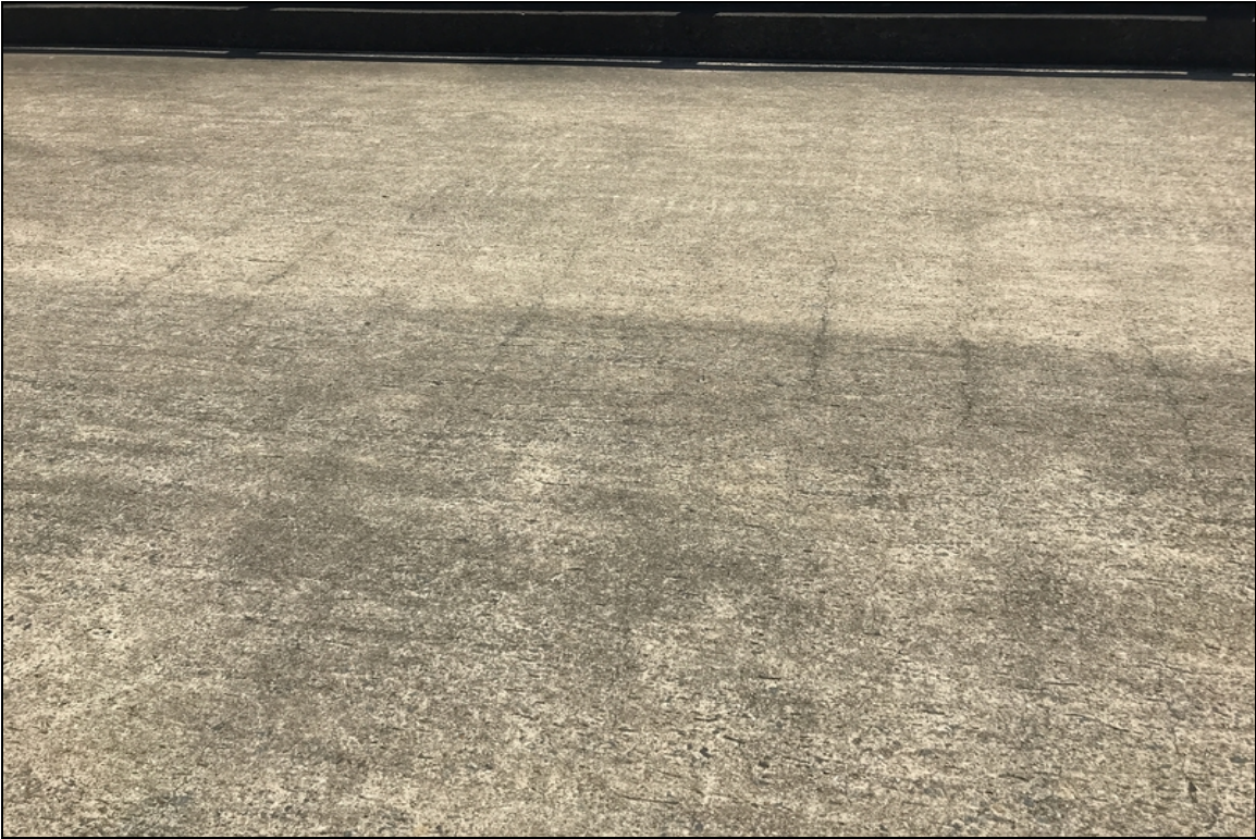
Span 4 longitudinal cracks up to 0.015"
