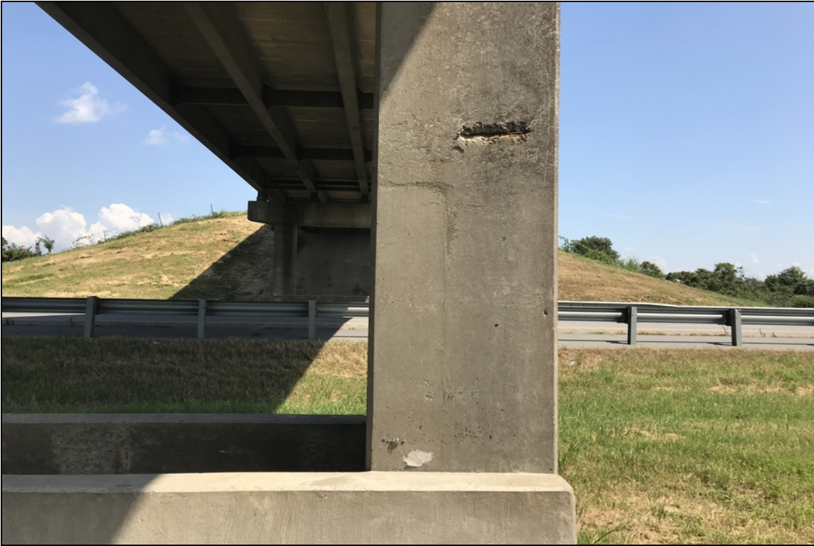
Bent 3 column 2 spall with exposed rebar
