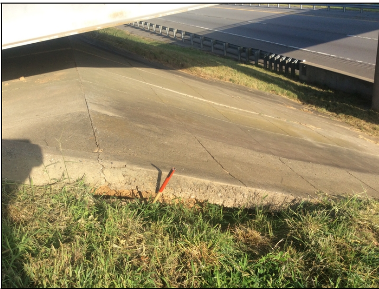
Large void under slope pavement at bent 1
