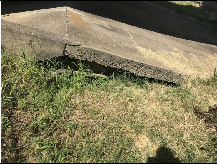
Large void under slope pavement at abutment 1.
