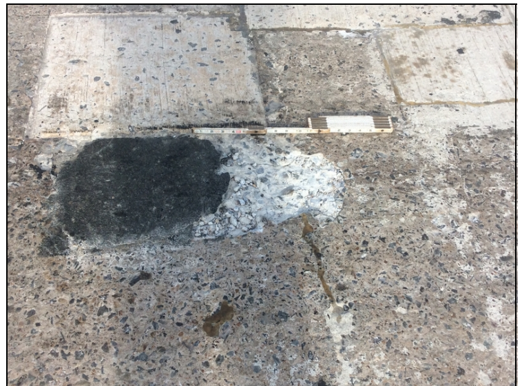
Span 2 has spall in deck.
