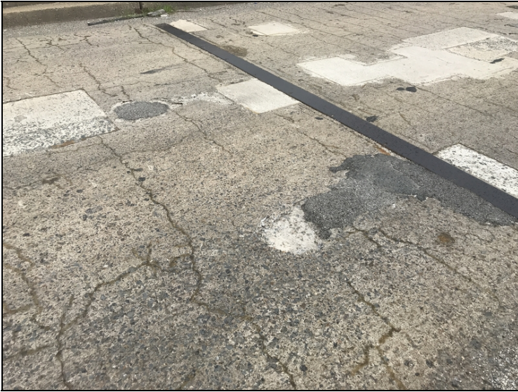
Span 1: large open spall and asphalt patches.
