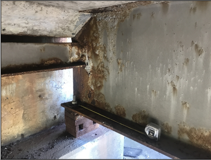
Span 1 beam 1 active corrosion
