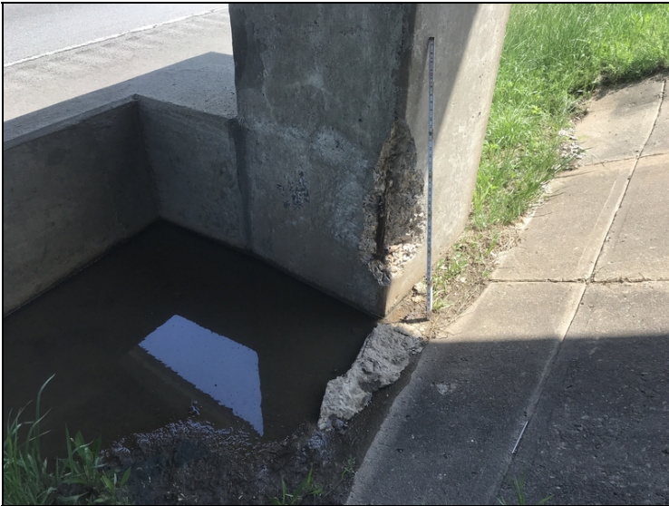
Bent 2, column 2: spall with exposed rebar
