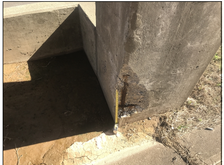
Large spall with exposed rebar on right column at bent 2
