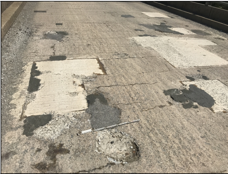
Span 3: multiple large spalls with exposed rebar and spalls with asphalt patches
