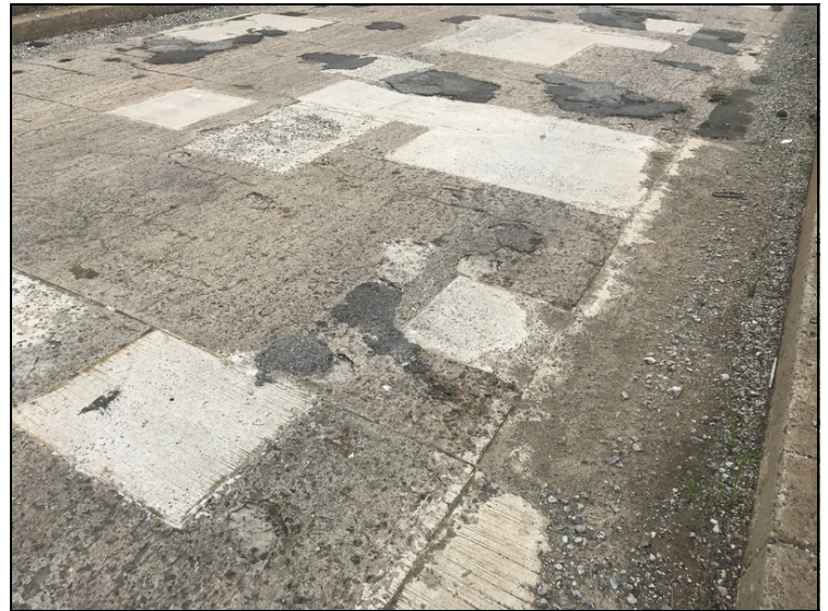
Span 3: numerous open spalls and asphalt patches.
