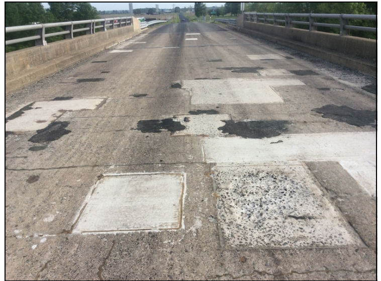
Span 3 has spalls and spalls filled with asphalt.
