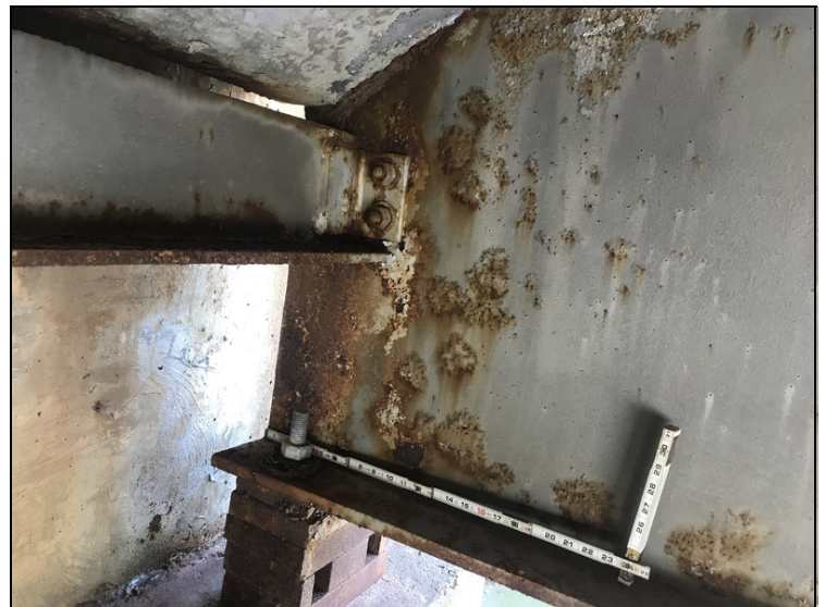
Span 1, girder 1: the beam end has flaking paint and active corrosion with areas of measurable section loss near the haunch
