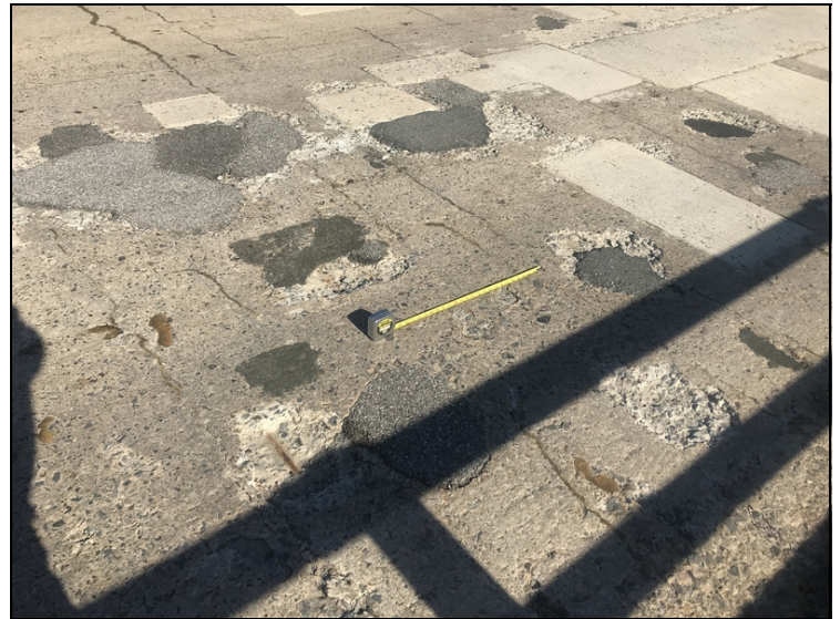
Span 2 multiple large spalls with exposed rebar and spalls with asphalt patches
