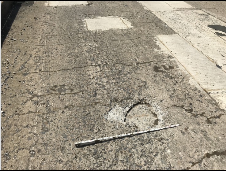
Span 1,northbound lane: large spall with exposed rebar
