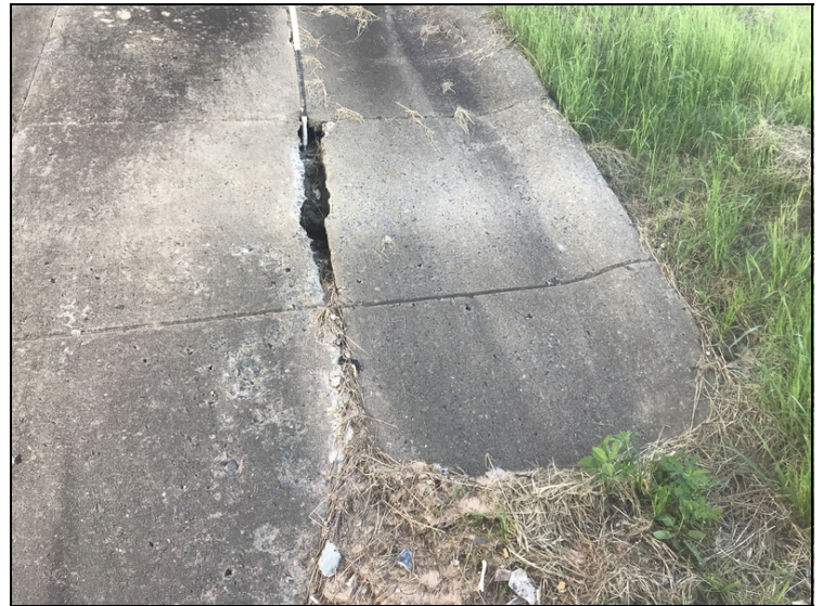
Slope paving under left side of span 1 is undermined from erosion.
