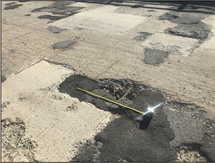
Span 3 multiple large spalls with exposed rebar and spalls with asphalt patches
