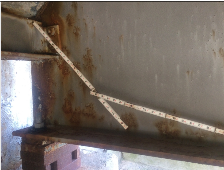
Span 1 beam 1 active rust with moderate pitting at upper web.
