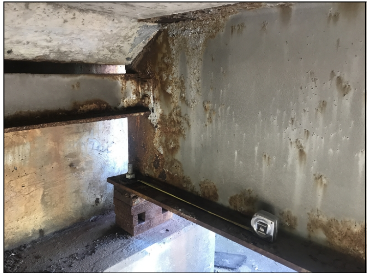
Span 1 beam 1 active corrosion
