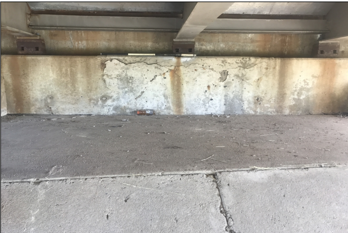
Bent 5 large delam in center of abutment
