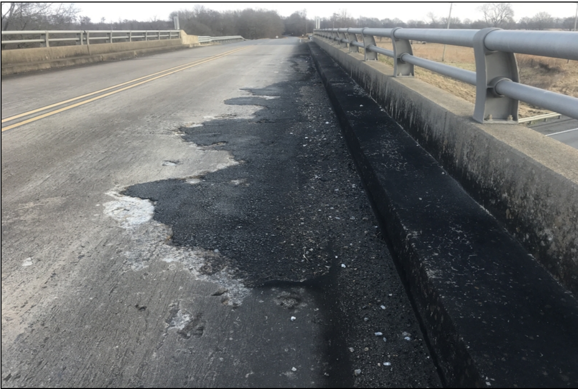
Span 3 deck has spalls filled with asphalt.
