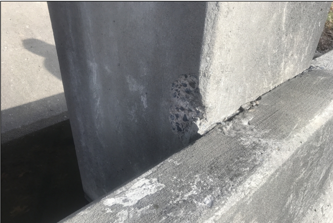
Bent 4 column 2 has spall.
