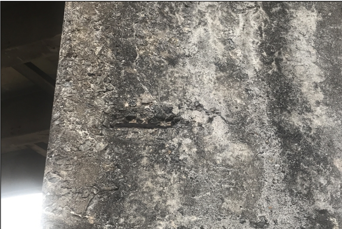
Bent 3 column 1 has spall with exposed rebar.
