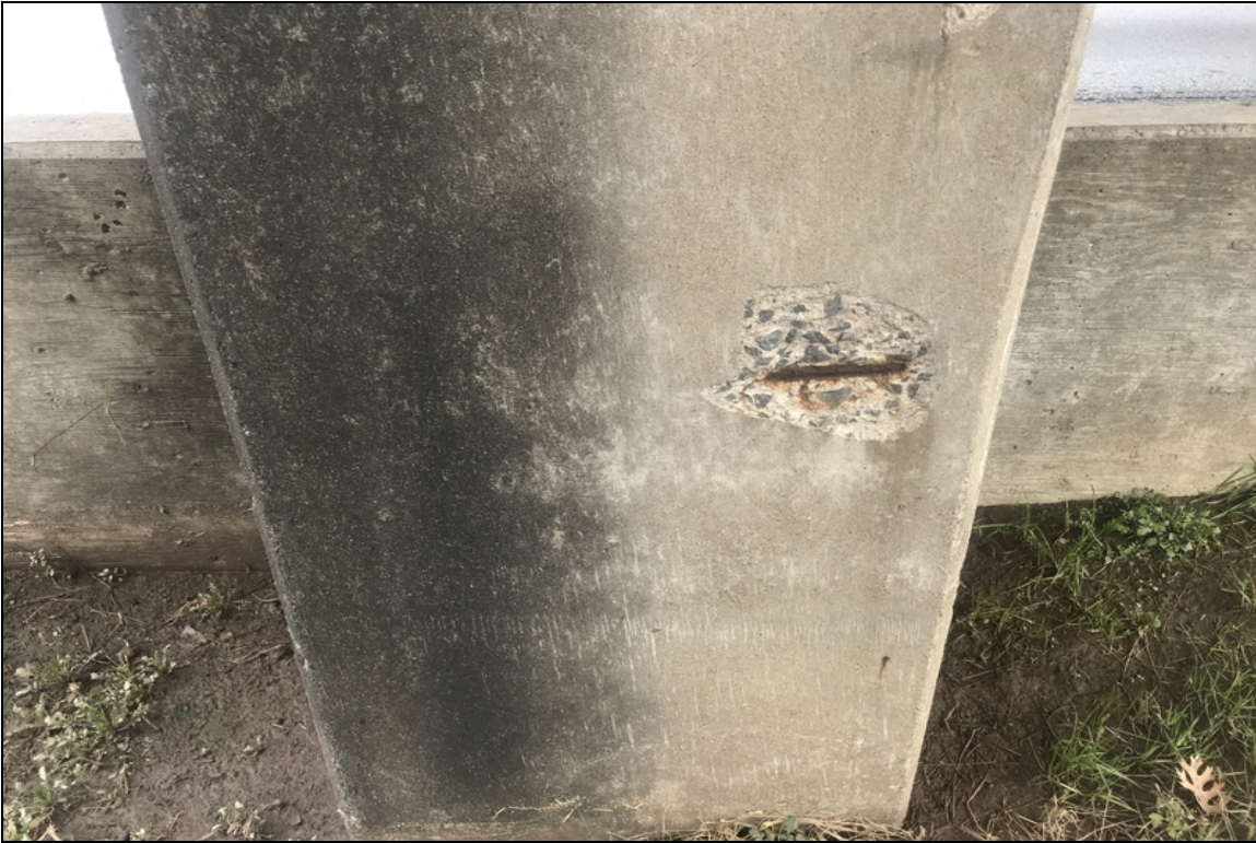
Bent 2 column 1 has spall with exposed rebar.
