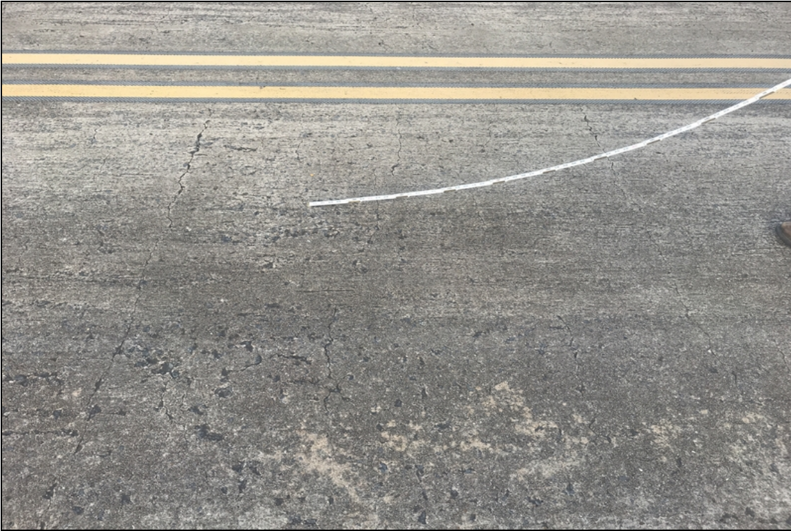
Deck span 3 has Longitudinal cracks up to 1/8". Common all spans.
