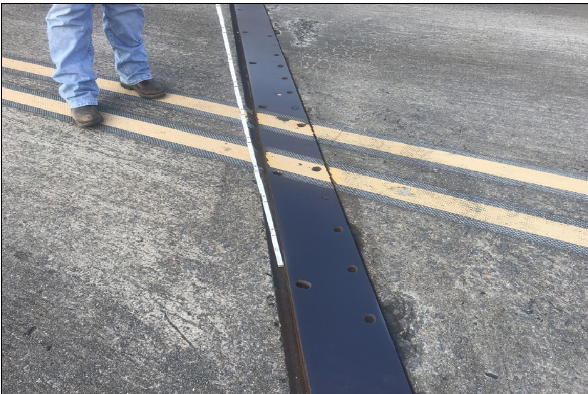
Sliding plate joint at bent 2 loose under traffic.
