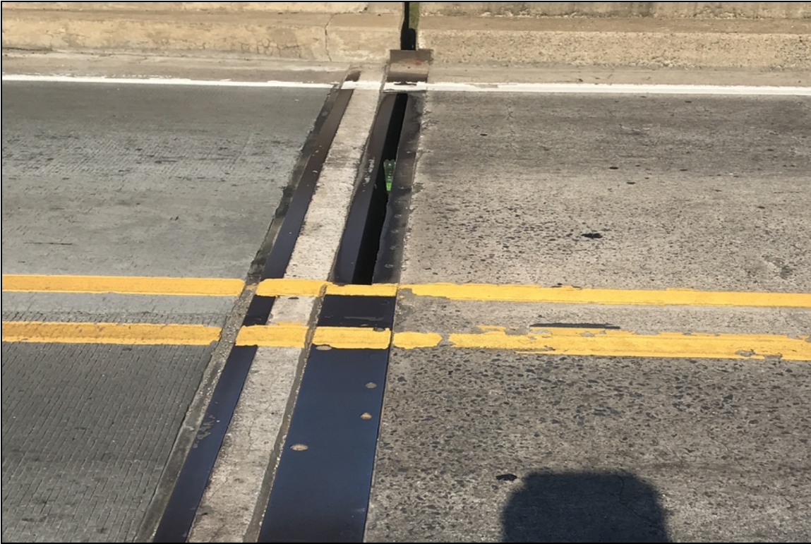
Bent 1 sliding joint plate missing.
