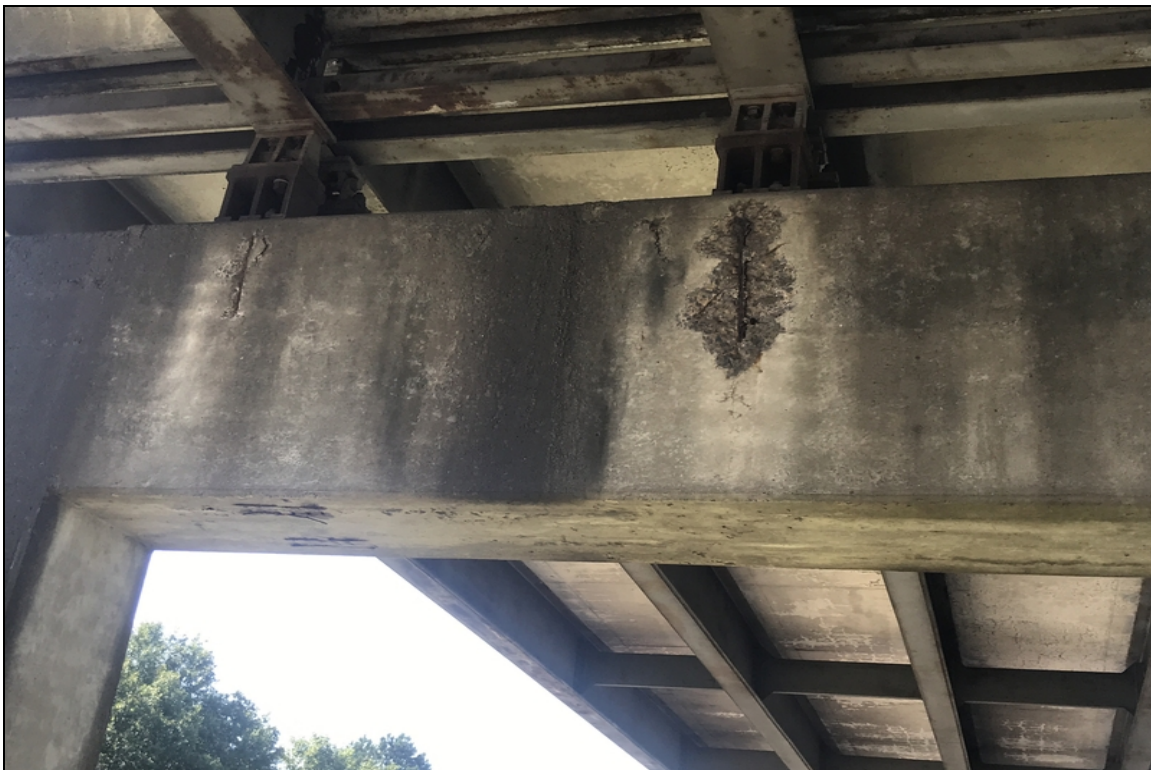
Bent 3 cap ahead face spall with exposed rebar.
