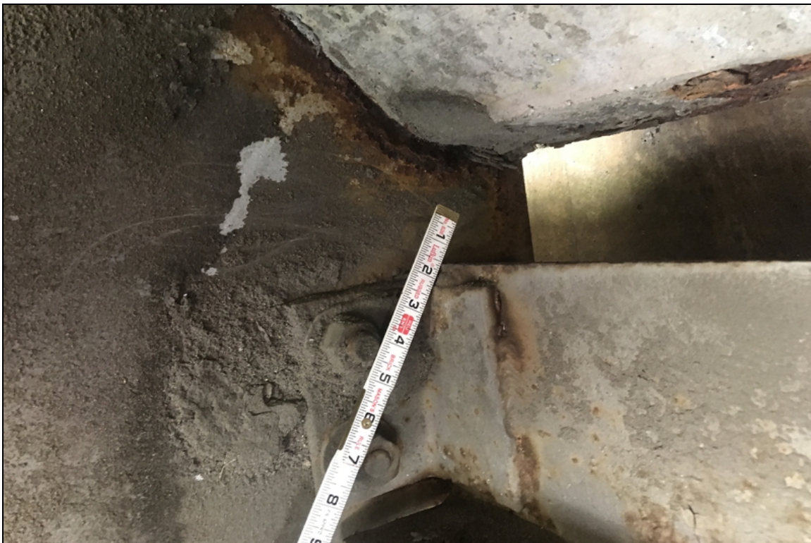
Bent 1 beam 3 active corrosion with pitting to upper web. Common all beam ends.
