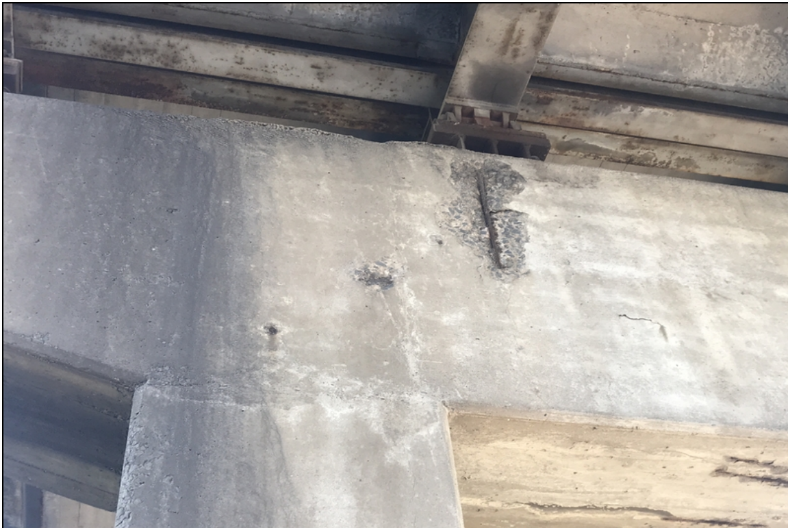
Bent 4 cap back spall with exposed rebar.
