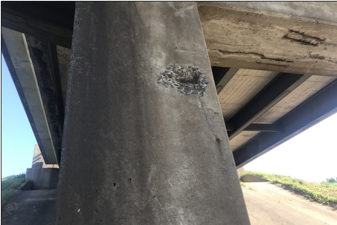
Bent 4 column 1 spall with exposed rebar.
