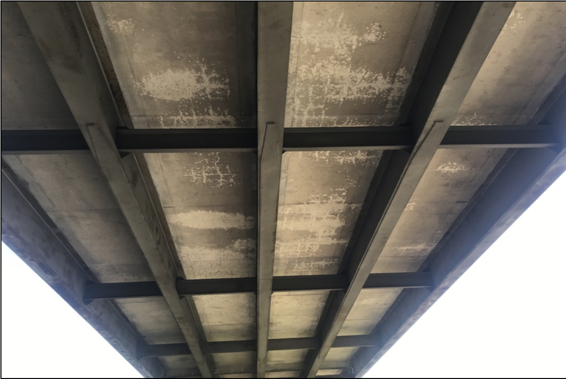
Span 2 soffit has areas of map cracks.
