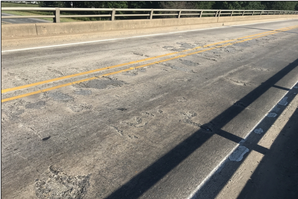
Span 2 spalls with exposed rebar.
