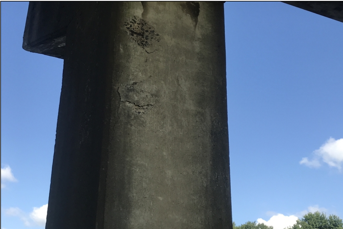
Bent 3 column 1 spall with exposed rebar right side.
