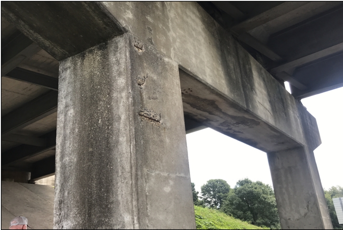
Bent 4 column 1 has spalls with exposed rebar.
