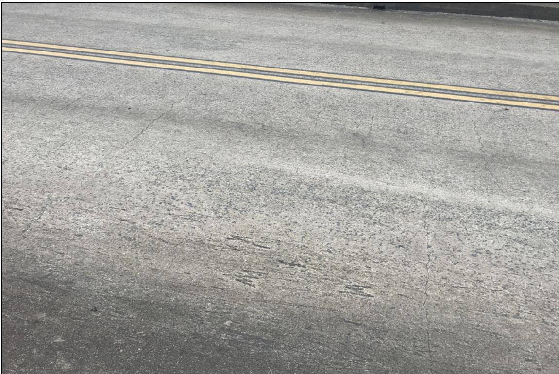
Deck span 4 has large unsealed transverse cracks. Common all spans.
