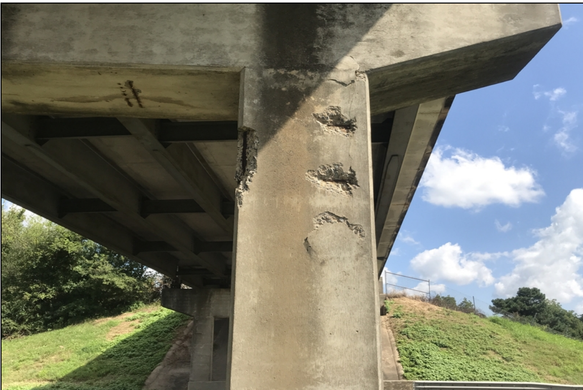
Bent 3 column 2 has spalls with exposed rebar.
