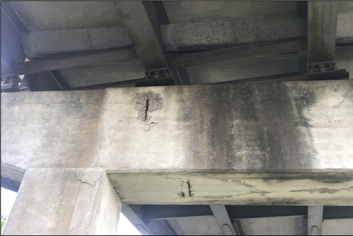
Bent 3 cap back has spall with exposed rebar.
