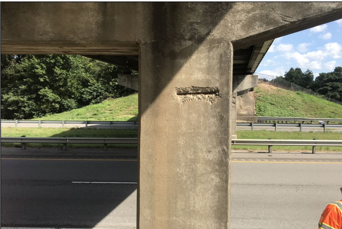
Bent 2 column 2 has spall with exposed rebar. Common column 1.
