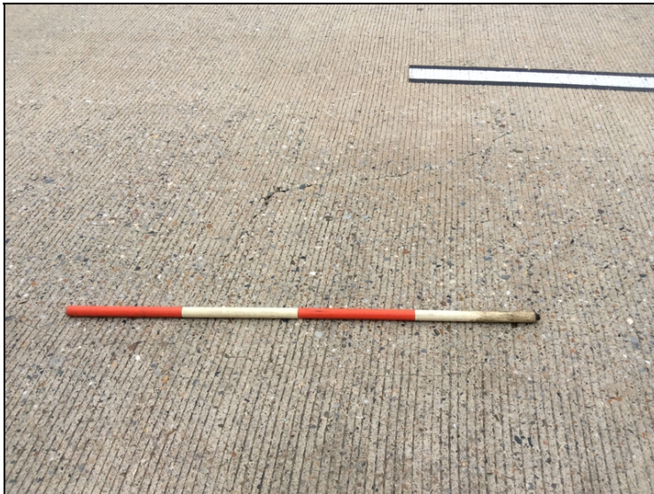
Span 6, deck cracks up to .050".
