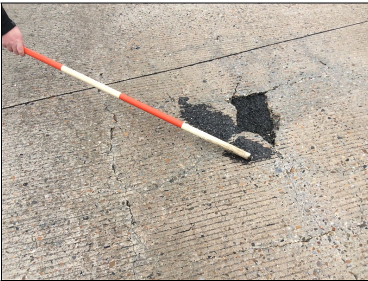
Span 2, spall filled with asphalt.
