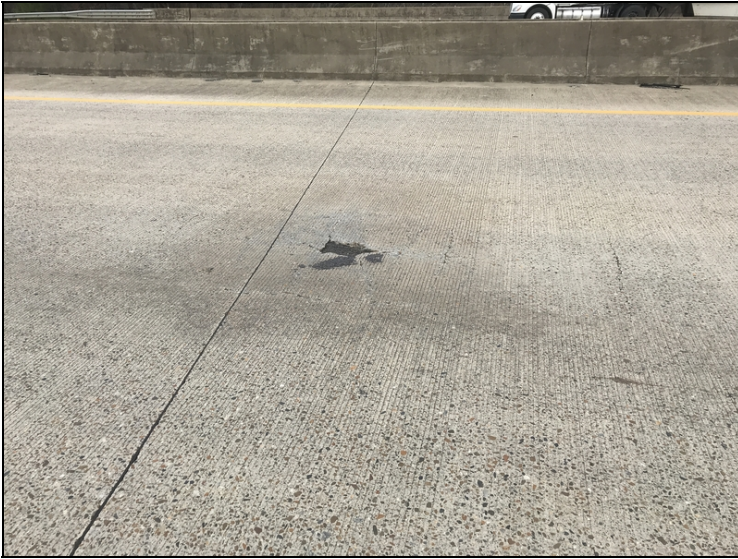
Span 2 right lane pothole.
