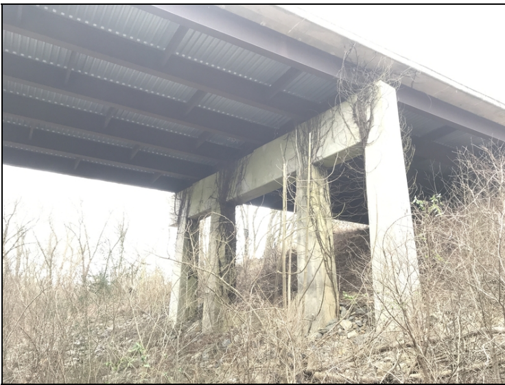
Bent 2, vines growing on columns and cap
