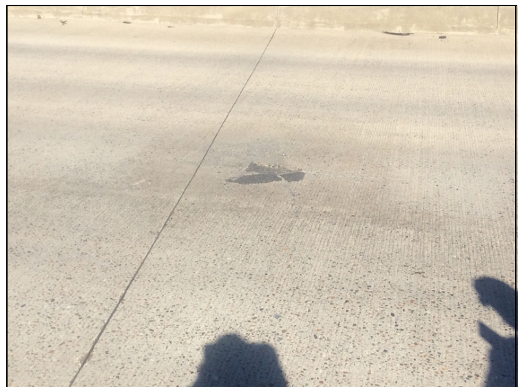
Spall filled with asphalt in deck at span 2.
