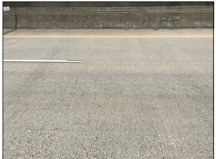
Span 4, large transverse cracks.
