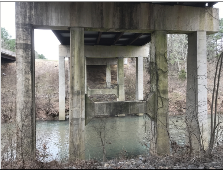
Bent 4, vines on column and cap Span 4, trees growing under bridge.
