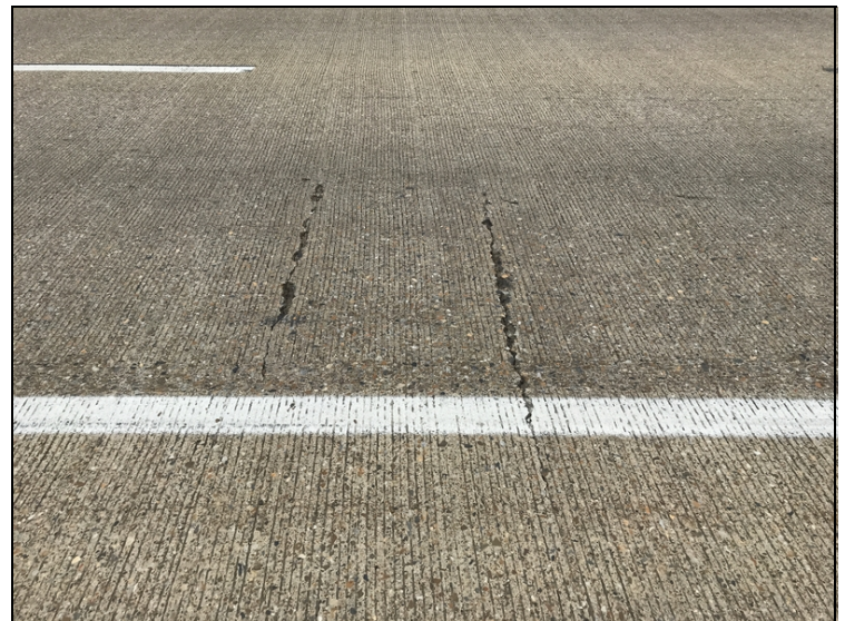
Span 6 left lane, large transverse cracks.
