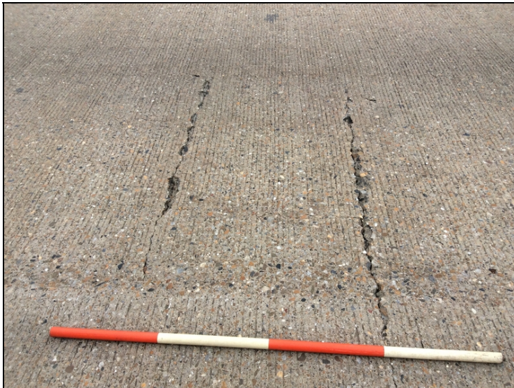
Span 6, 1/8" cracks that have spalled at the top.
