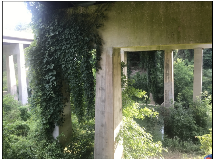
Bent 2 has vines and trees growing under and against bridge.
