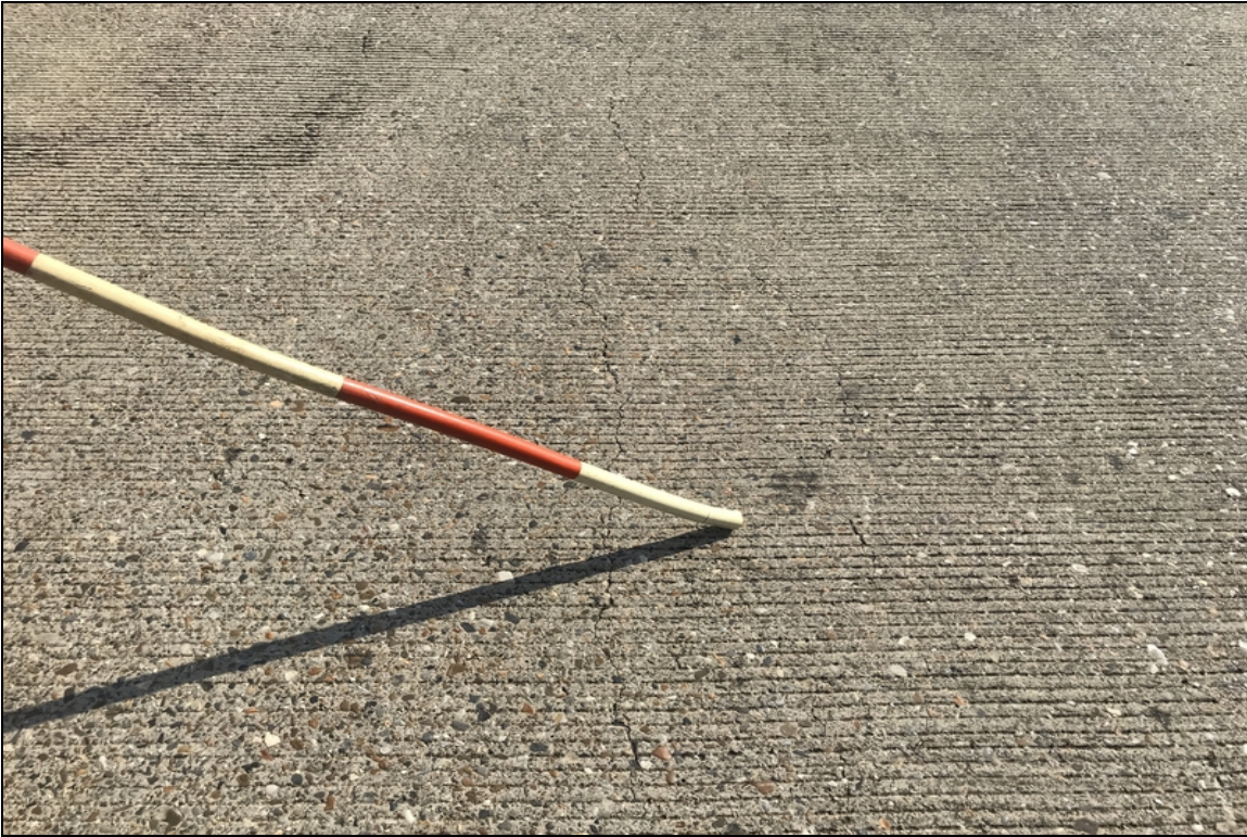
Span 1 has longitudinal cracks in the deck.
