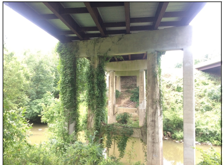
Bent 4, vines growing on columns and cap.
