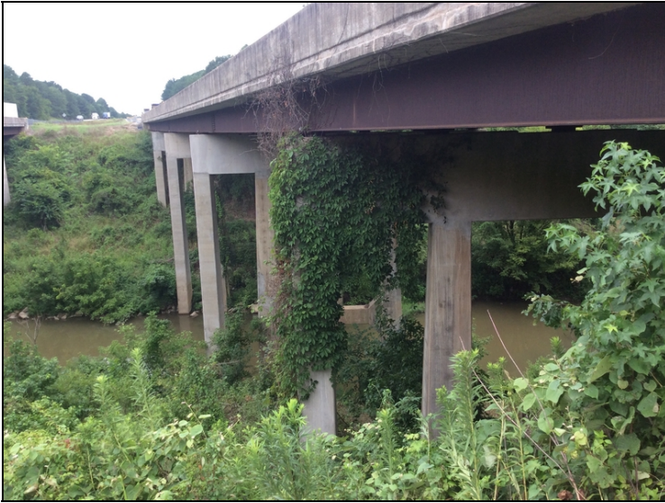
Bent 2, vines growing on column 1, cap and soffit.
