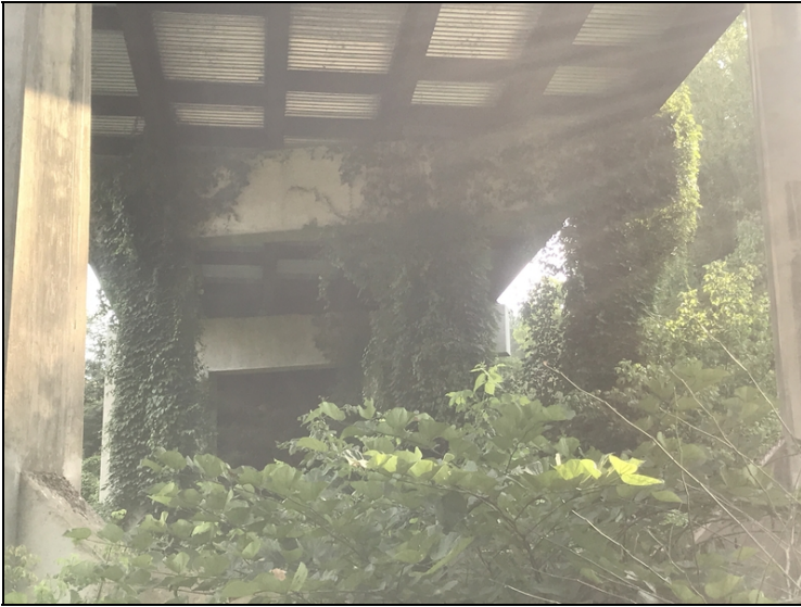
Bent 4 has vines growing on all columns under bridge.
