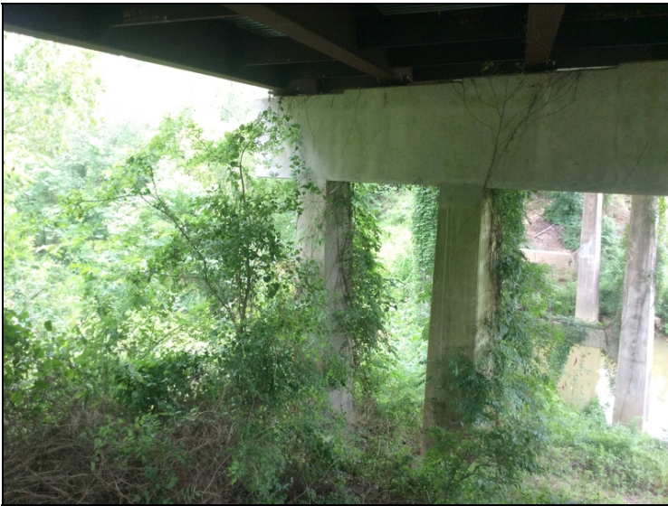
Span 5, bent 5, small trees growing under the bridge, vines growing on columns and cap.
