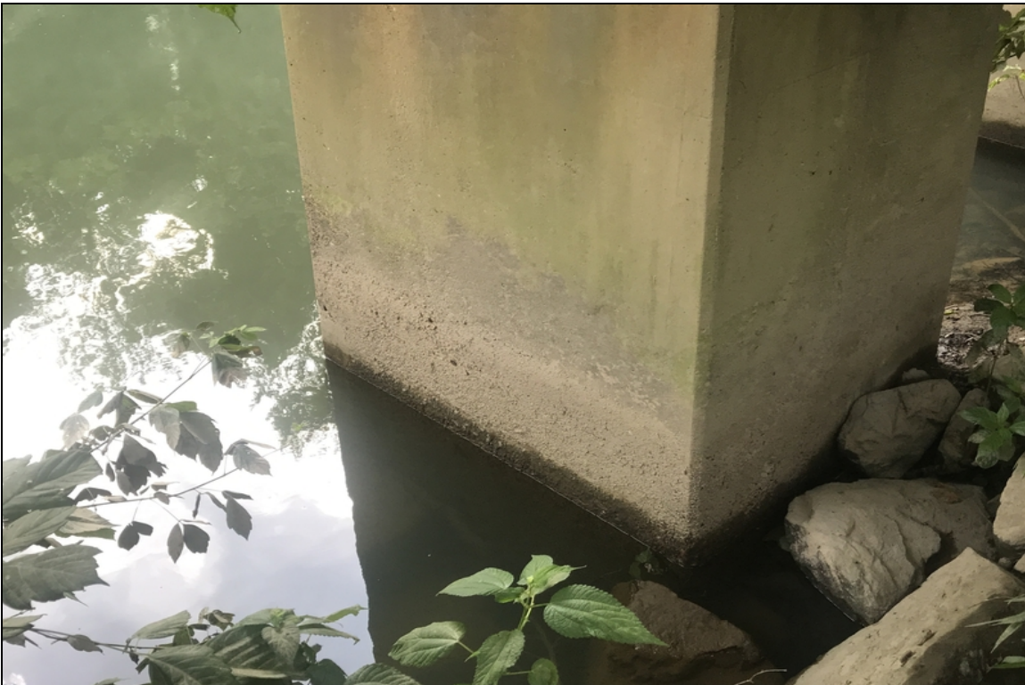
Bent 3 column 3 has abrasion at the bottom of column, common bent 4 columns.
