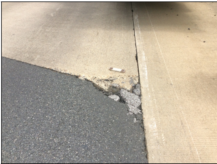
Large spall at the west approach right lane.
