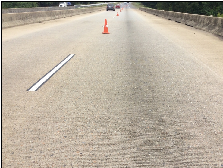
Both edge stripes on the bridge are worn and not visible.
