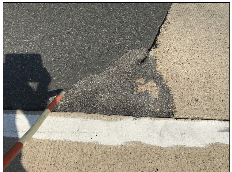
State forces have patch spall in West approach slab.
