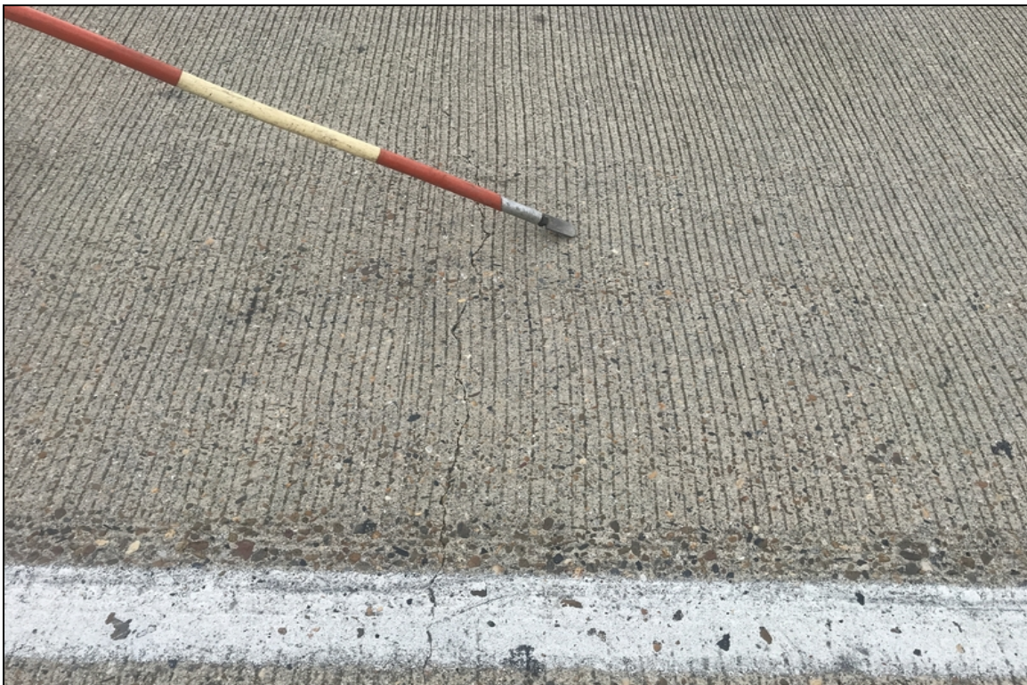
Span 1 has transverse cracks in the deck.
