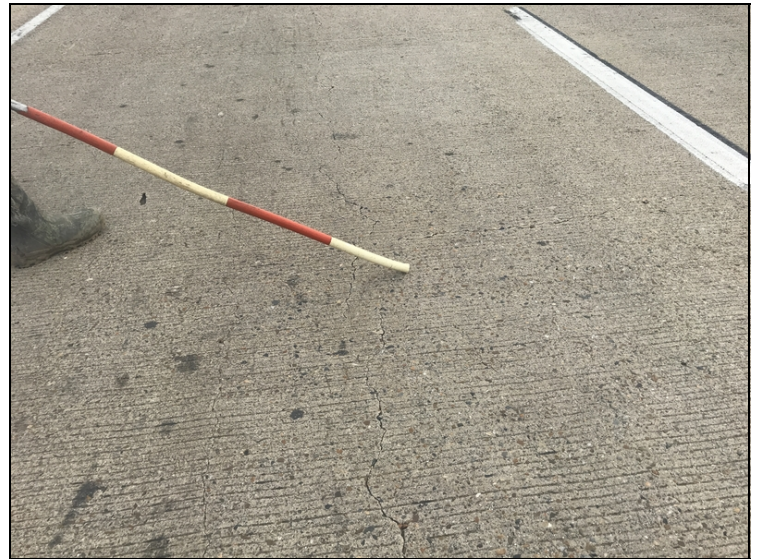
Span 3 deck has longitudinal and transverse cracks in the deck.
