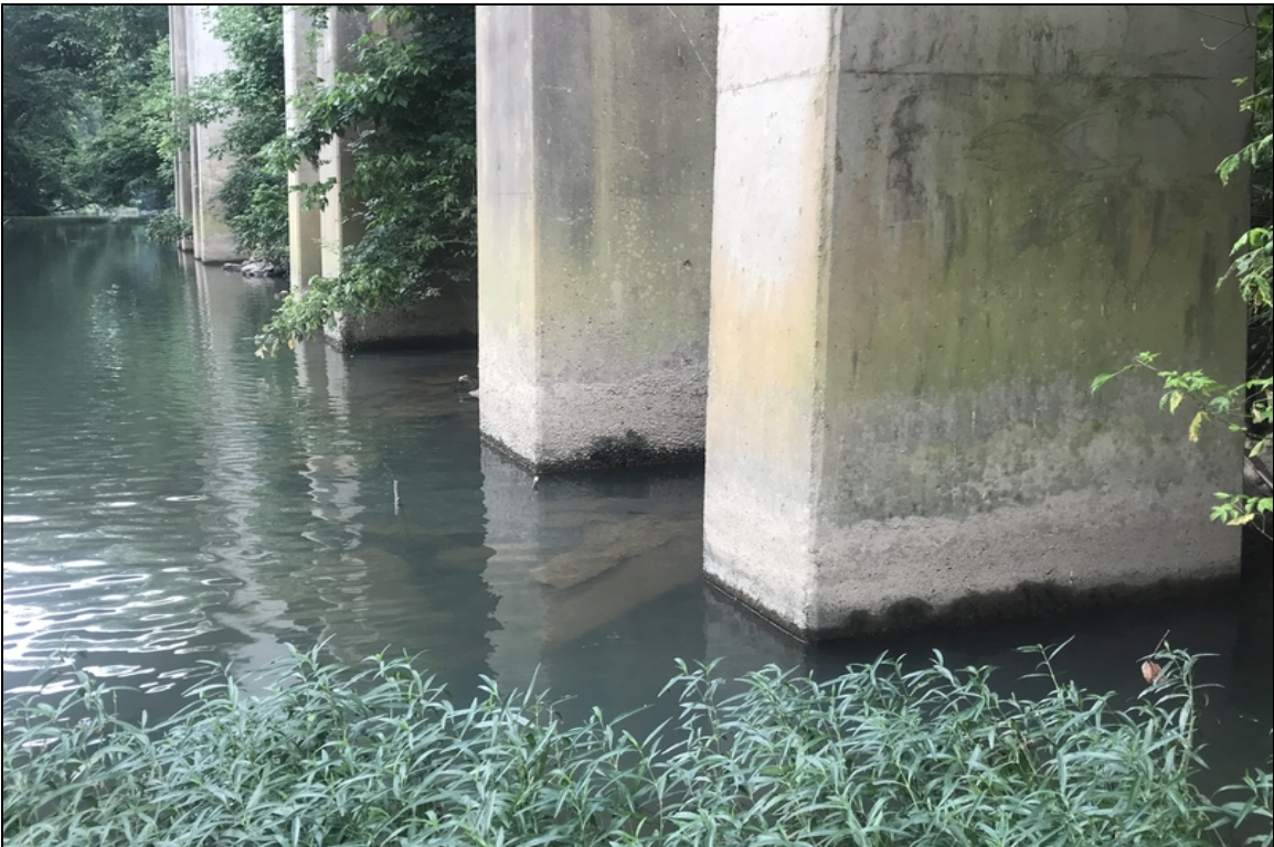
Bent 3 columns have abrasion, common bent 4.
