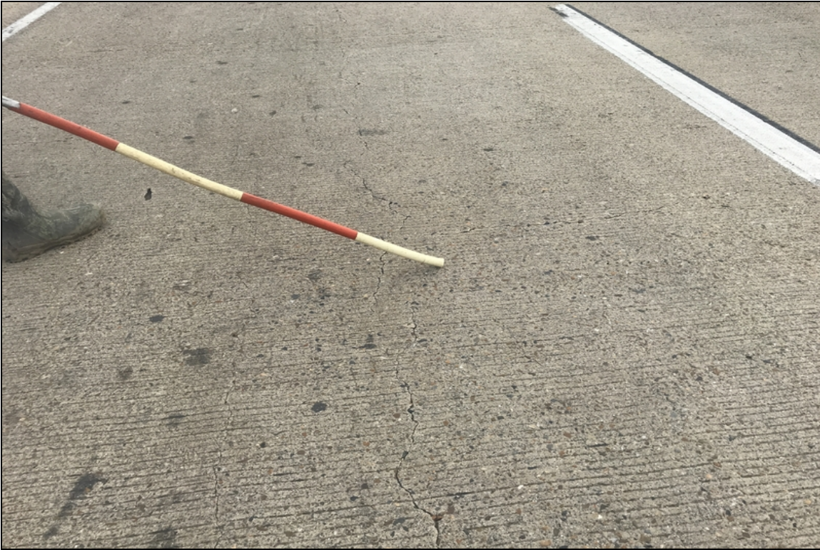
Span 3 deck has longitudinal and transverse cracks in the deck.
