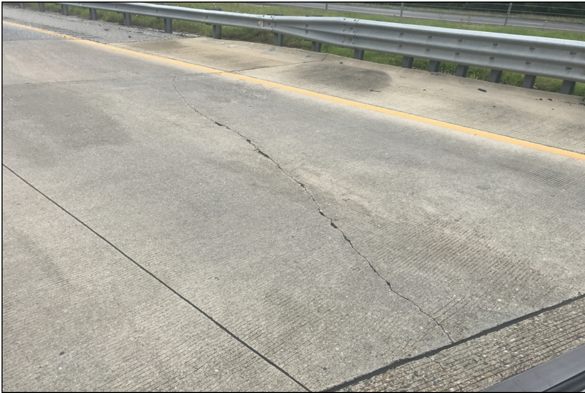
East approach slab has large unsealed longitudinal crack.
