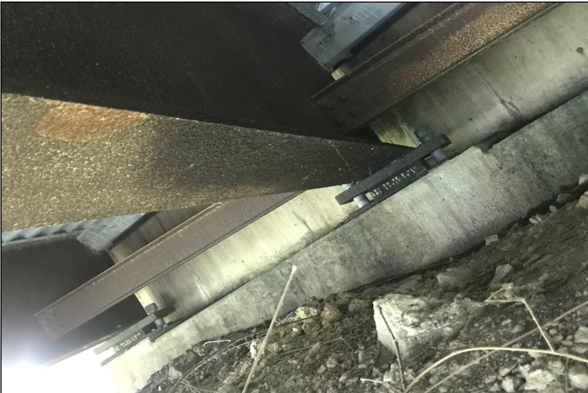
Span 1 beam 4 has small flakes of rust on the bottom flange.
