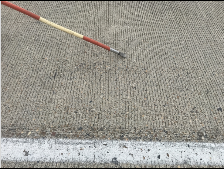
Span 1 has transverse cracks in the deck.
