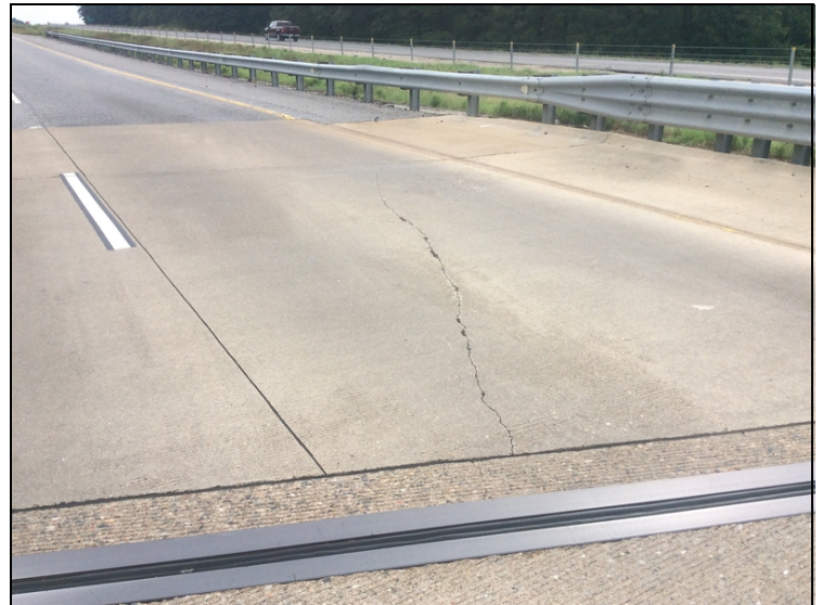
Large longitudinal crack east approach left lane.
