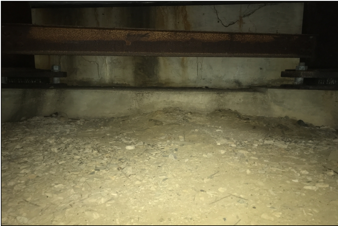
Bent 6 abutment has cracks with efflorescence in the back wall.
