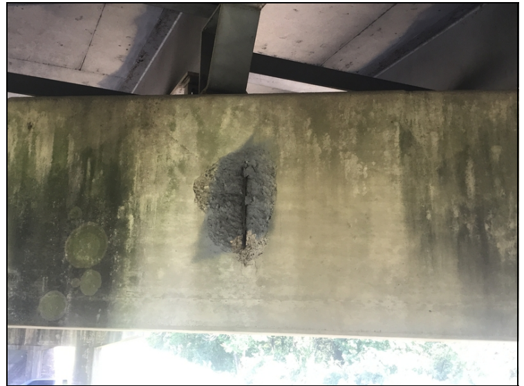
Bent 4 cap ahead has spall with exposed rebar.
