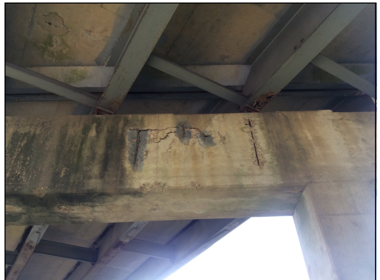
Bent 3 cap spalls with exposed rebar
