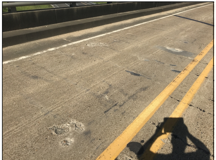
Deck span 4 has spalls in the right lane.
