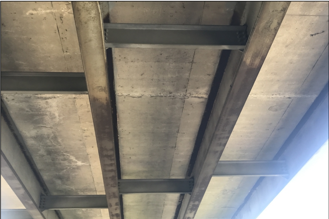
Span 2 soffit over west bound traffic small delams.
