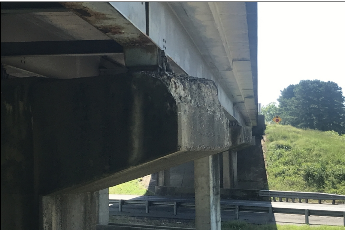
Bent 2 cap right side has spall with exposed rebar.
