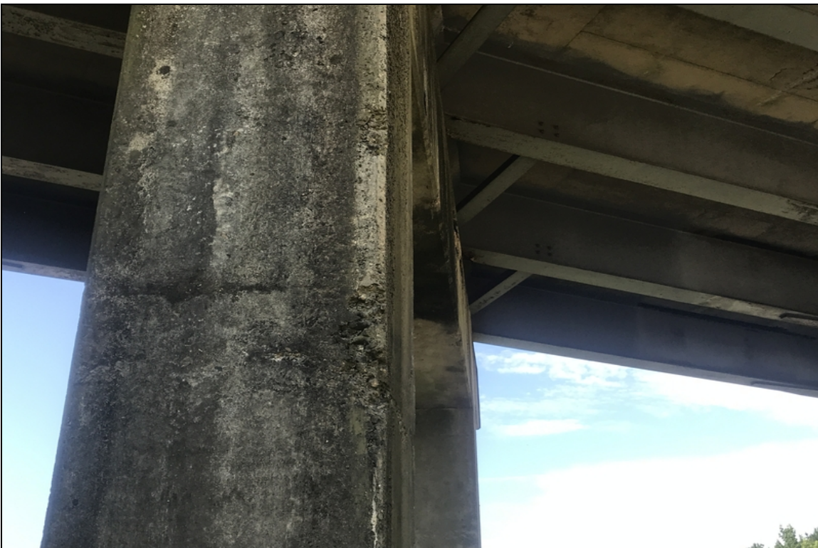
Bent 3 column 1 has spalls.
