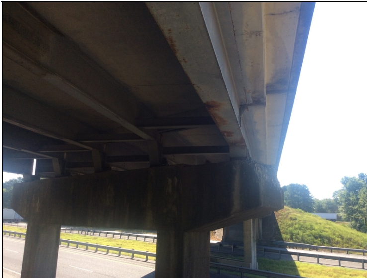
Bent 2 right side, end of cap is deteriorating exposing the reinforcing steel.
