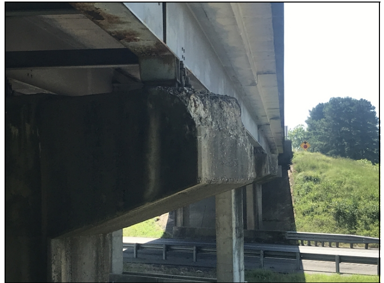
Bent 2 cap right side has spall with exposed rebar.
