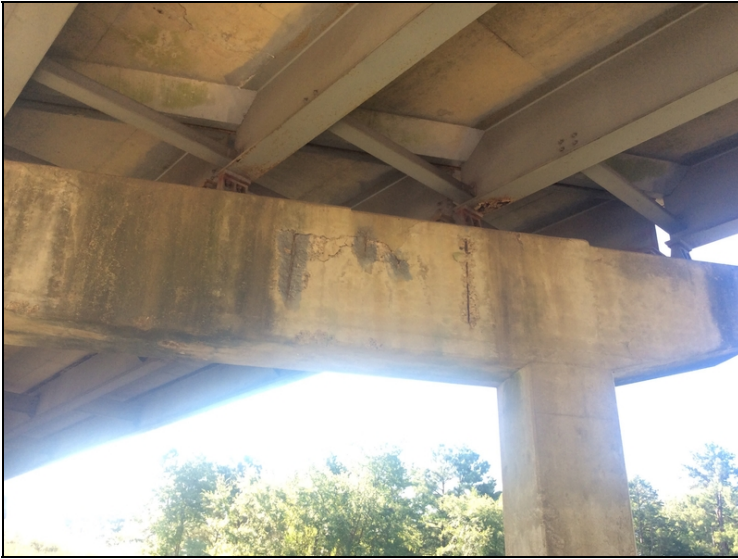
Bent 3, 9' of spall with exposed reinforcing steel that has section loss.
