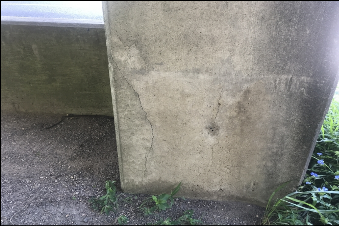
Bent 2 column 2 has cracks near the bottom of the column.
