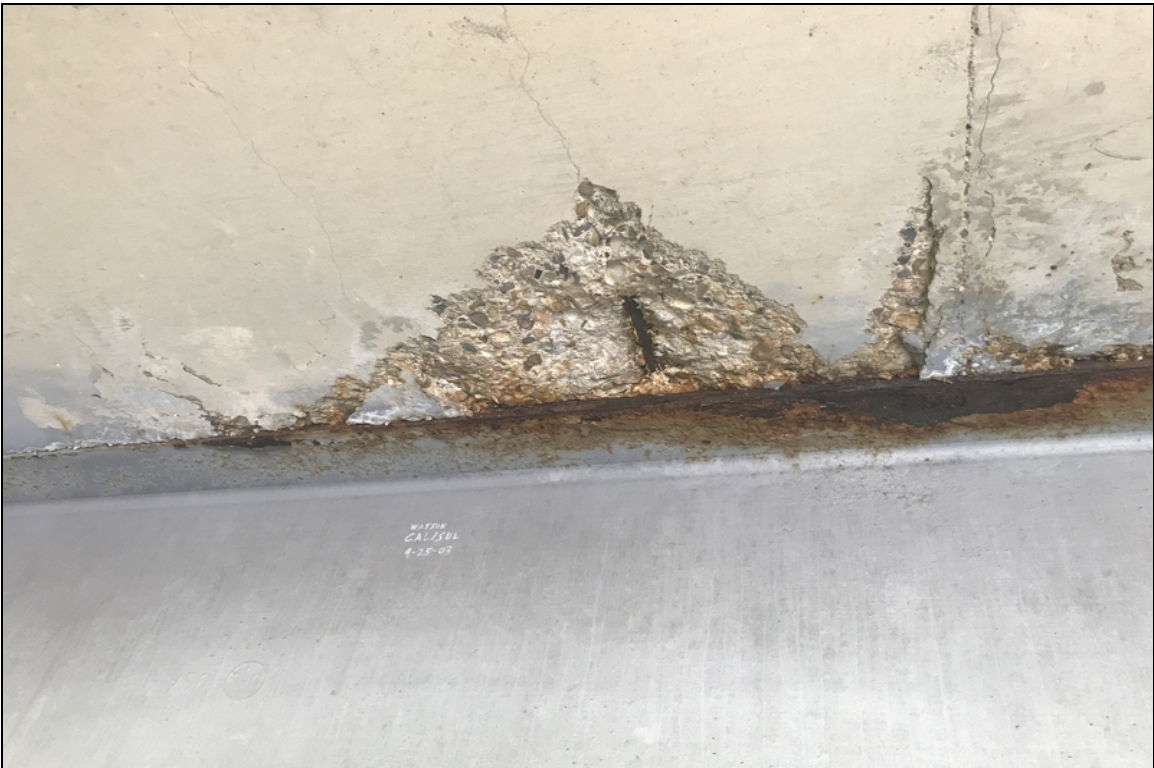
Span 1 soffit bay 1 has spall with exposed rebar.
