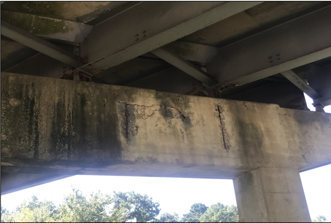
Bent 3 cap back has spalls with exposed rebar.
