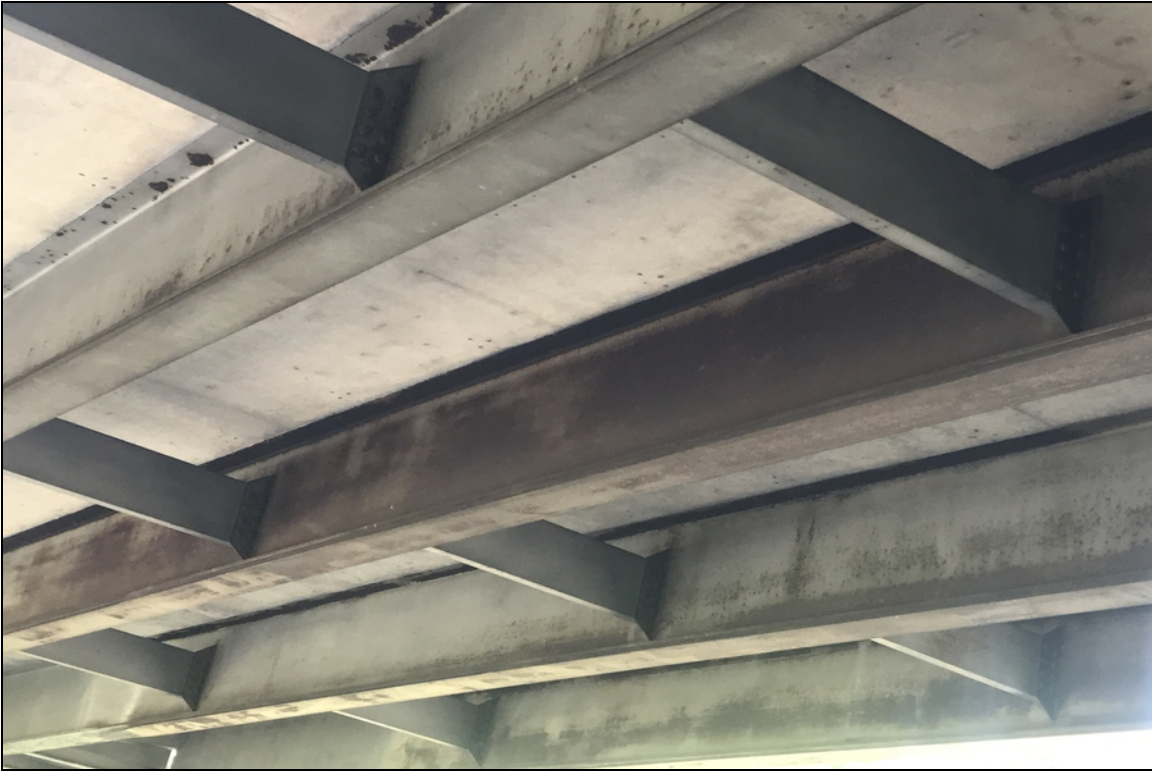
Span 2 beam 3 has surface rust mid span.
