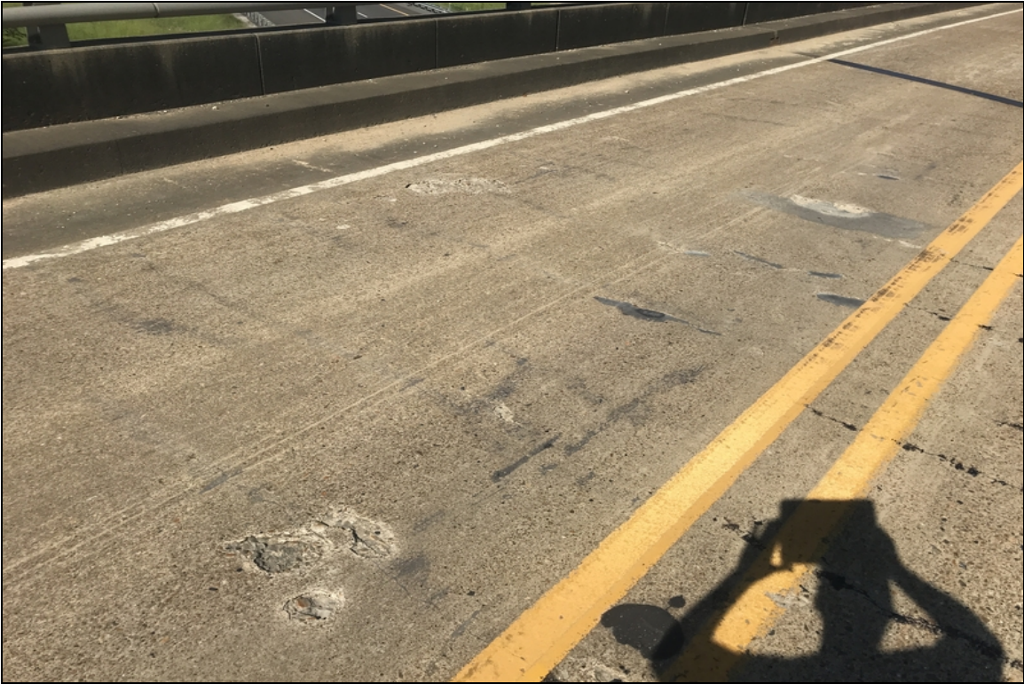
Deck span 4 has spalls in the right lane.
