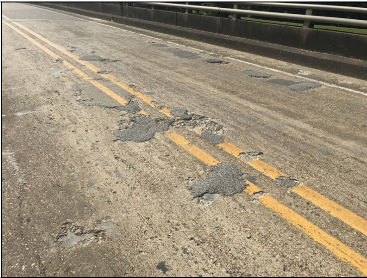
Deck span 2 has spalls and spalls filled with asphalt.
