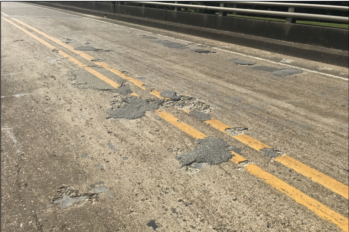
Deck span 2 has spalls and spalls filled with asphalt.
