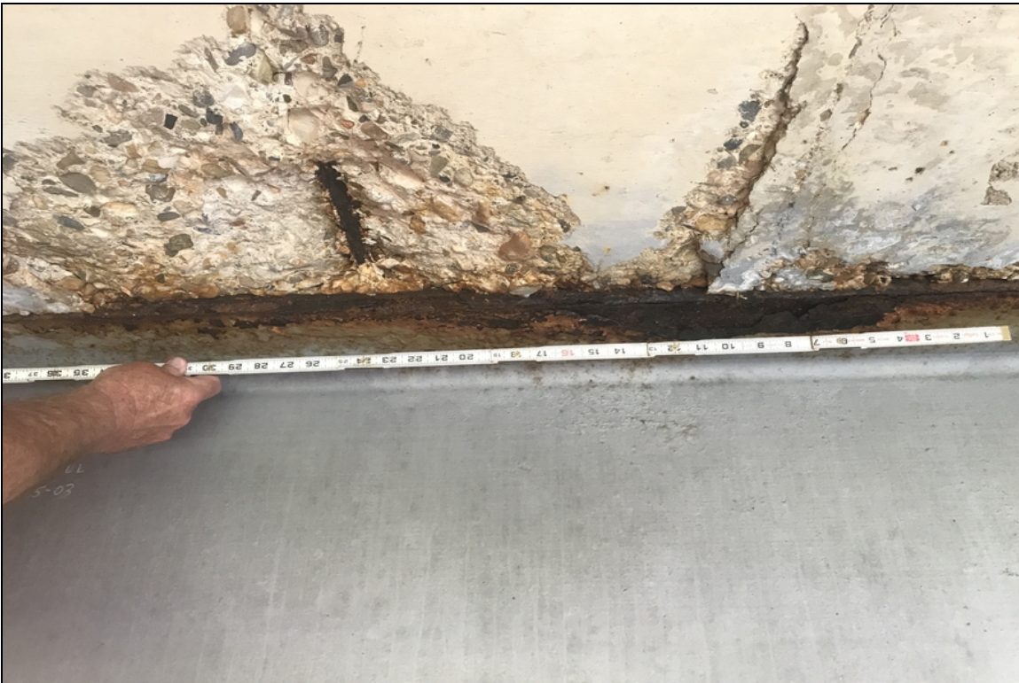
Span 1 beam 1 has corrosion, pitting up to 1/16".
