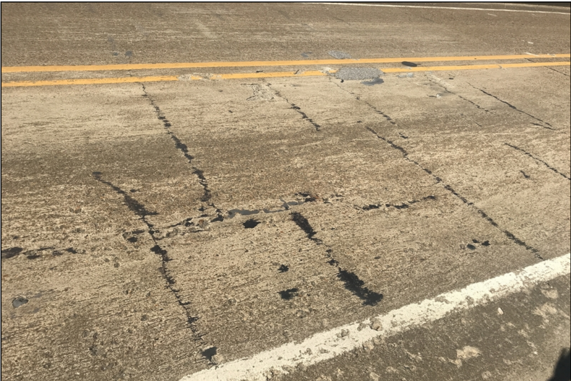
Deck span 3 has sealed transverse cracks, common all spans.
