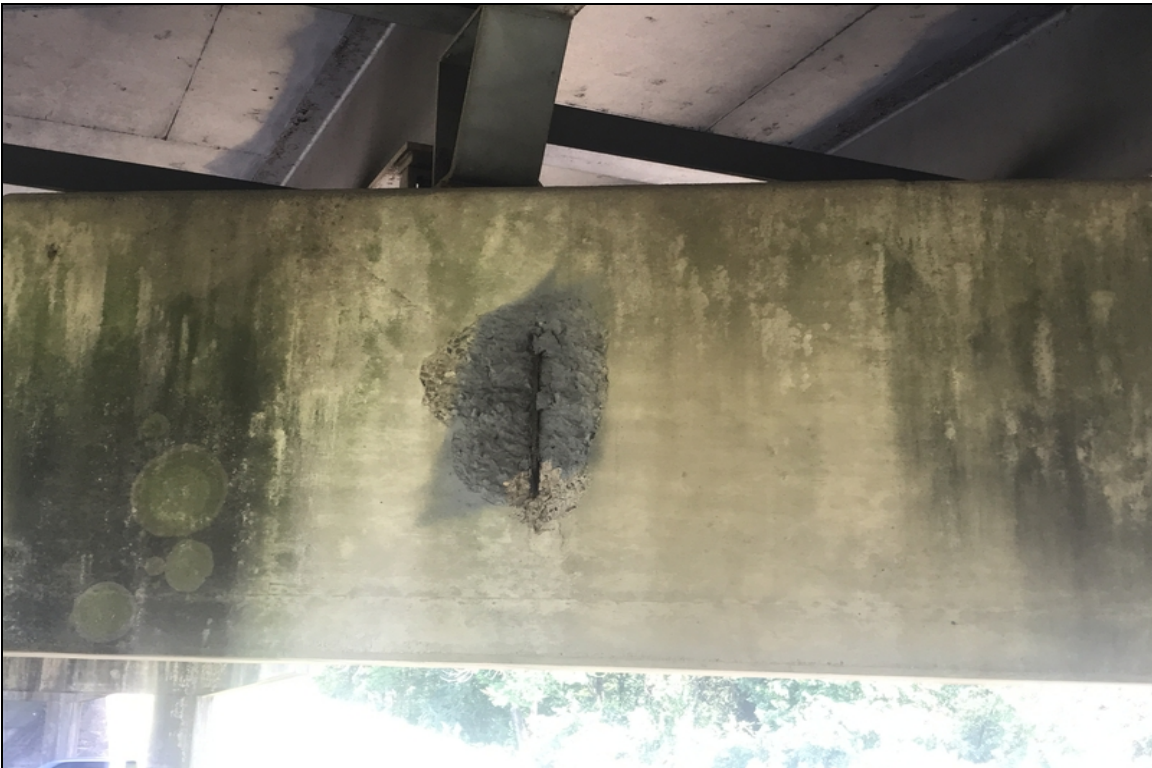
Bent 4 cap ahead has spall with exposed rebar.
