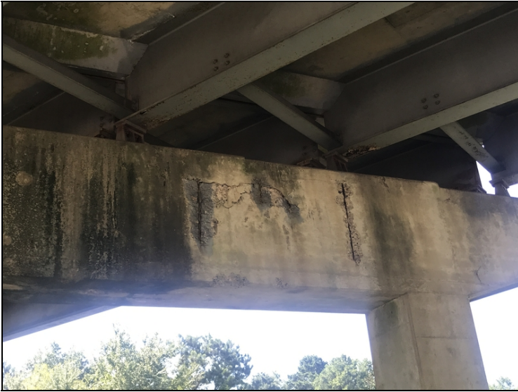
Bent 3 cap back has spalls with exposed rebar.
