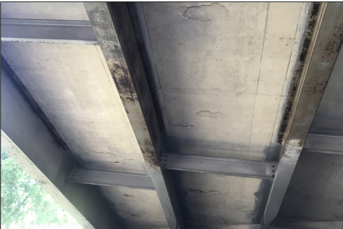
Soffit span 4 has spalls, spalls with exposed rebar, and delams in the soffit.
