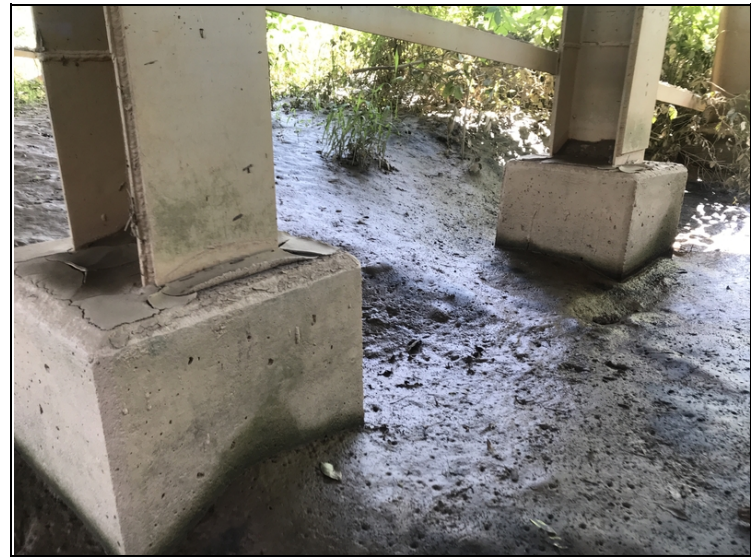
Bent 3 Pile at top of encasement, dirt and silt causing rust to form.
