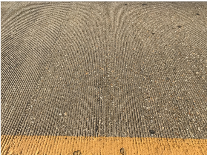
Span 3, transverse crack.
