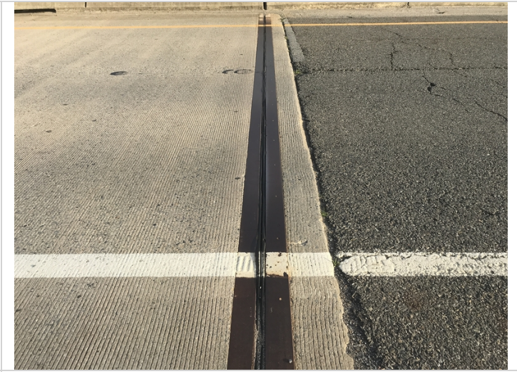
Bent 6, joint seal is bulging and damaged.
