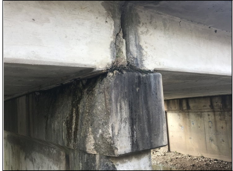
Left ahead end of Bent 6 has loss 2 inches of bearing area.
