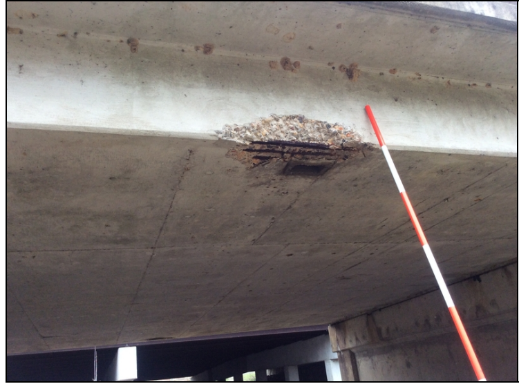
Span 4 right side spall with exposed rebar.
