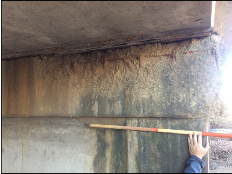
Bent 6 ahead side: large spall with exposed rebar.
