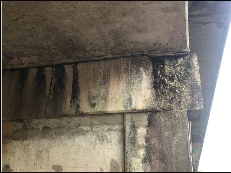
Bt. 4, ahead left en of cap, spall with exposed rebar.
