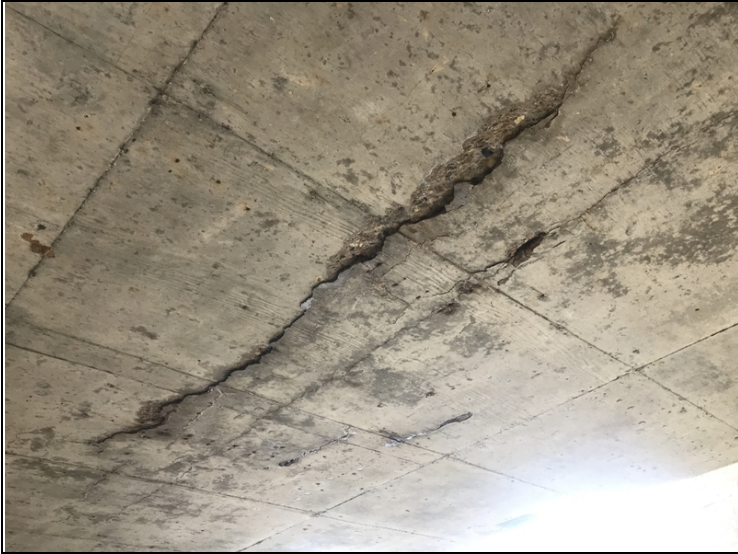
Span 2, delam with rust staining.
