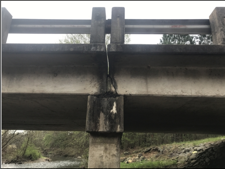
Span 1 left end, at Bt. 2, spall at the end of the slab.
