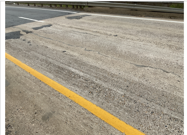
Deck cracks span 6
