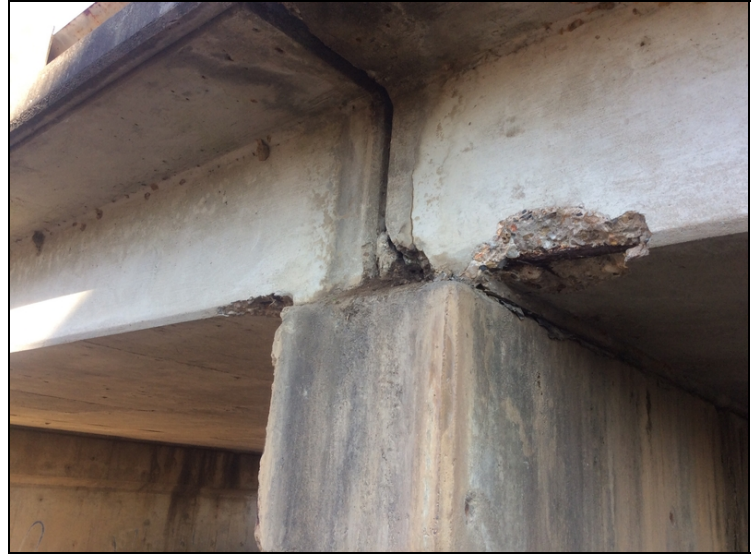
Right side bent 6: the end of span 7 is spalling.
