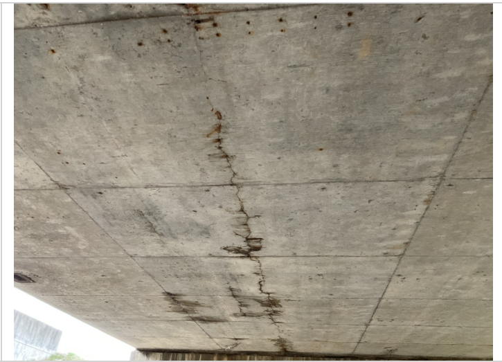
Cracks with rust staining span 5
