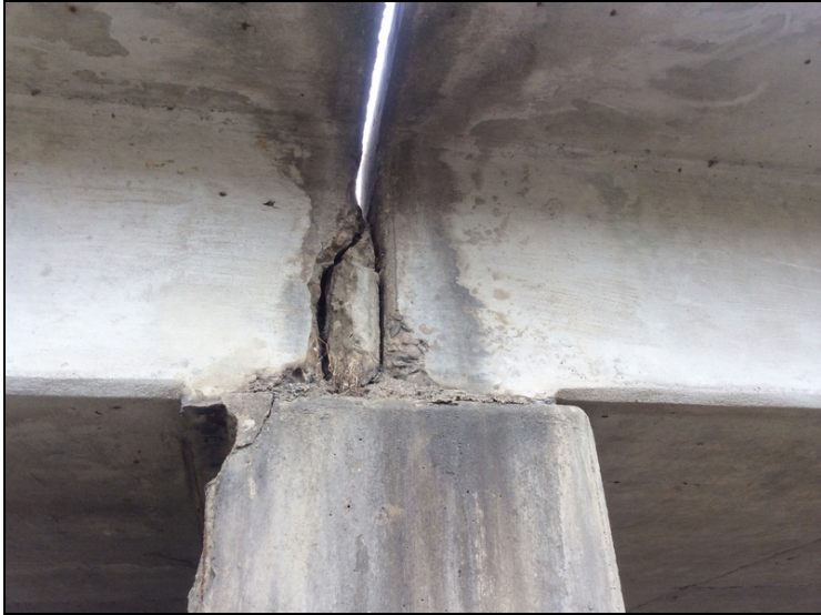
Span 6 left side delamination on end of slab.
