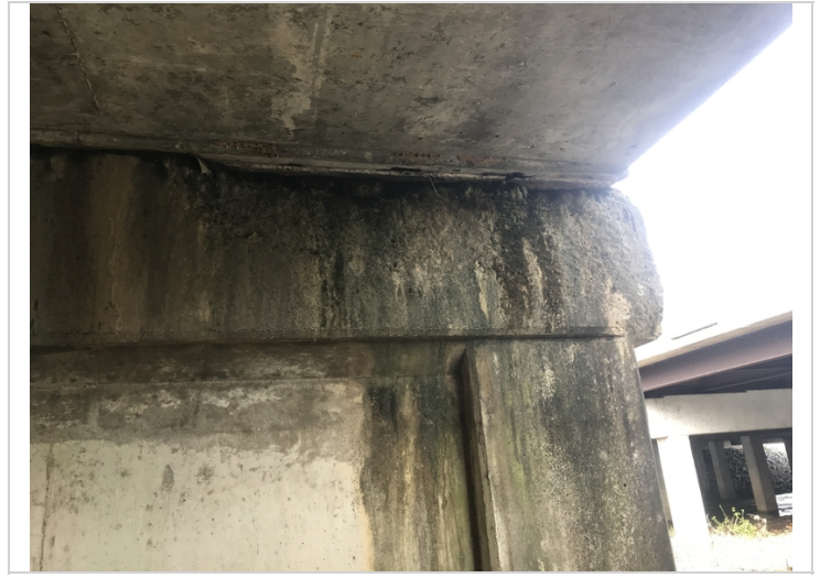
Bt. 6 ahead left end, spall with exposed rebar.
