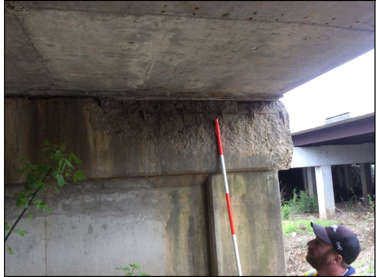
Bent 6 pier wall ahead spall with exposed rebar.
