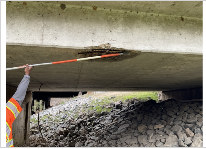
Spall with rebar in span 6
