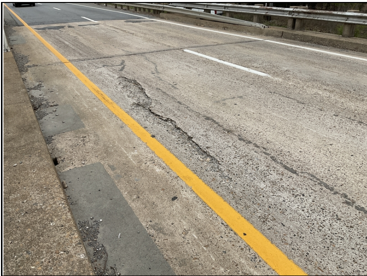
Scaling span 5
