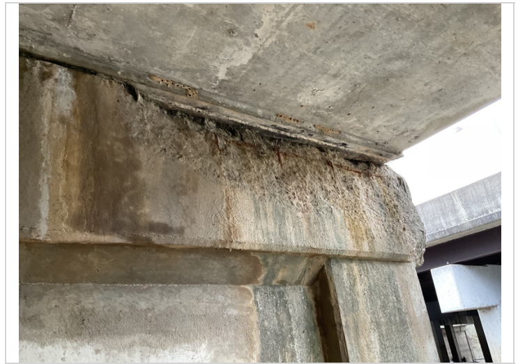
Spall with rebar in the cap at bent 6
