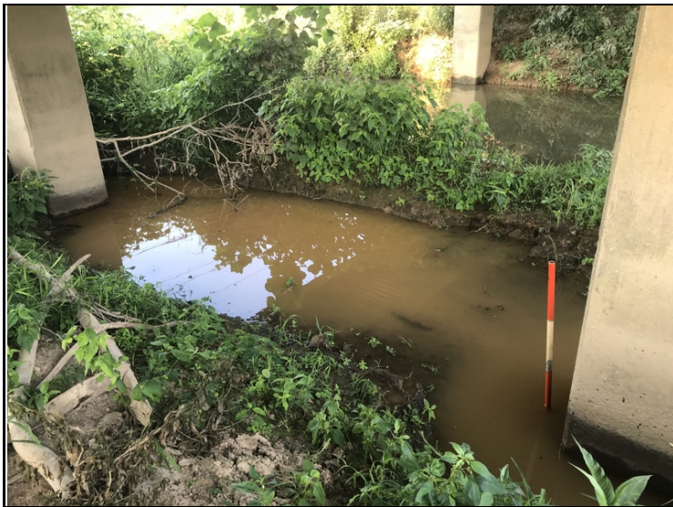
Local scour action at bent 3.
