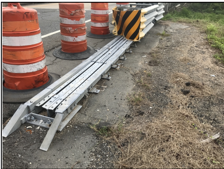
West end of bridge guard rail crash barrier damaged.
