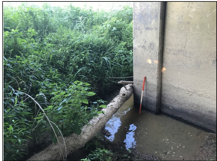
Bent 4: right side of pier 4 local scour action and log resting against pier.
