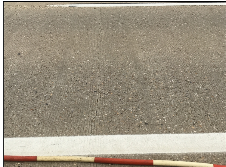
Deck span 4 transverse cracks up to 0.050 wide.
