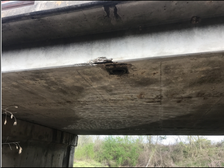
Span 5, right side , exposed rebar.
