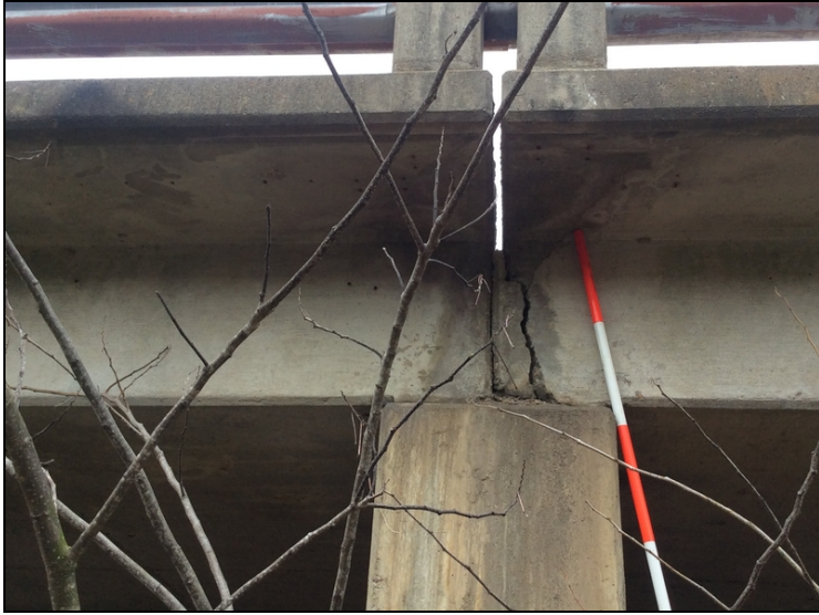
Span 6 at bent 6 right side of slab has large delam
