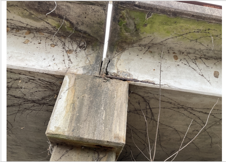
Bent 2 left side large vertical crack and exposed rebar
