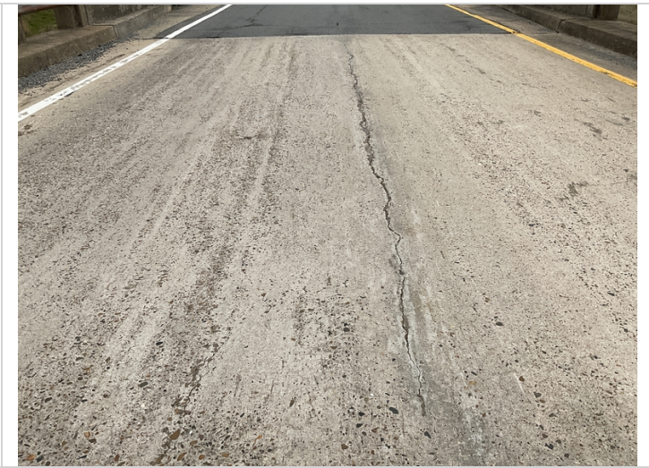
Deck cracks span 6
