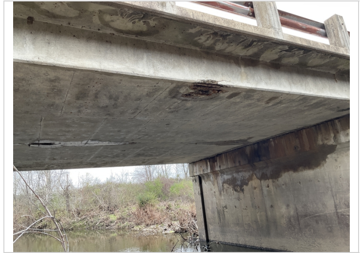
Spall with rebar span 3
