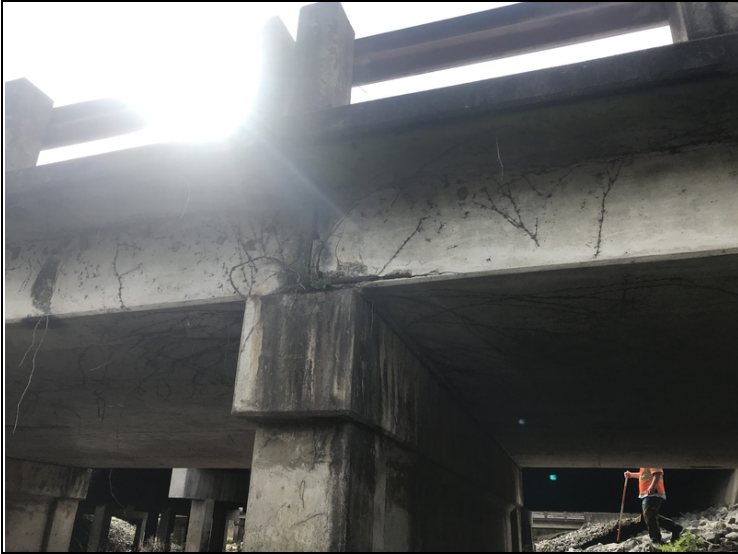
Left end of span 1, Bt. 2, spall with exposed rebar.
