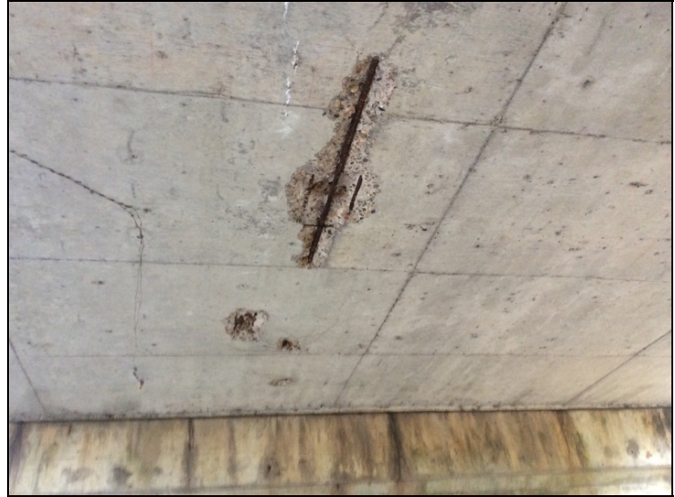
Span 2 spalls with exposed rebar.
