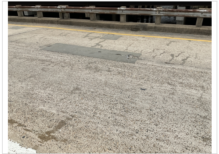
Spall in the deck span 3
