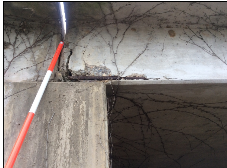
Bent 2 span 1 right side spall with exposed rebar.
