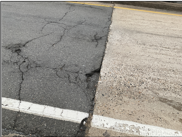
Potholes at bent 7 approach
