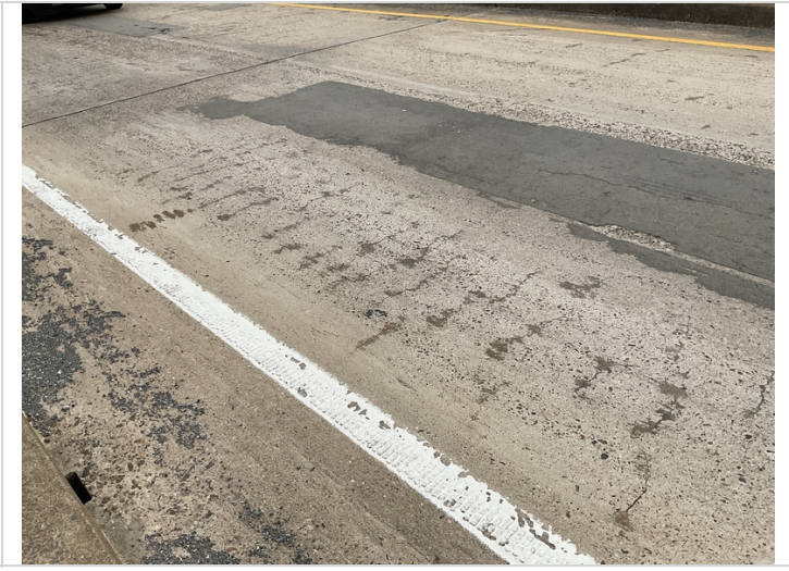
Sealed deck cracks span 2
