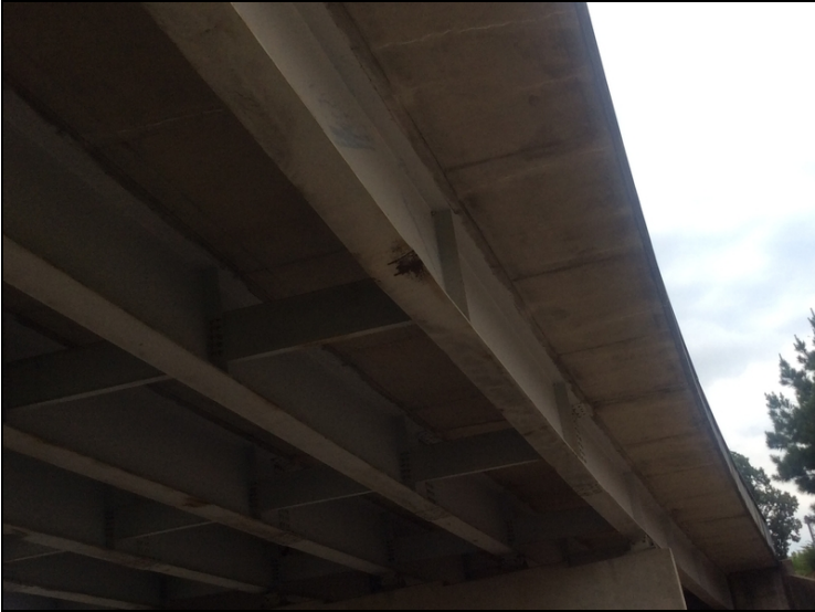
Span 3 girder 6 bottom flange is misaligned due to traffic impact.
