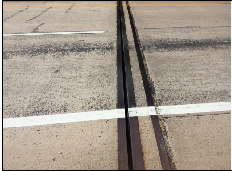
Bent 1 joint seal missing
