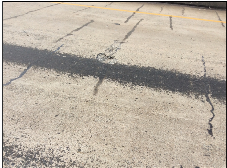
Span 2 spall with exposed rebar
