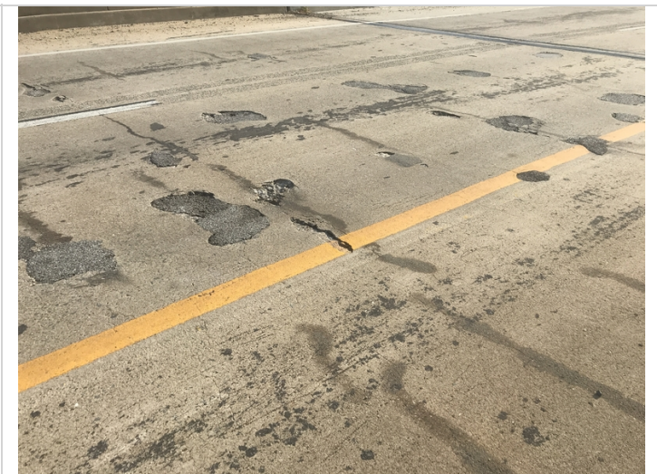
Spalls and spalls filled with asphalt
