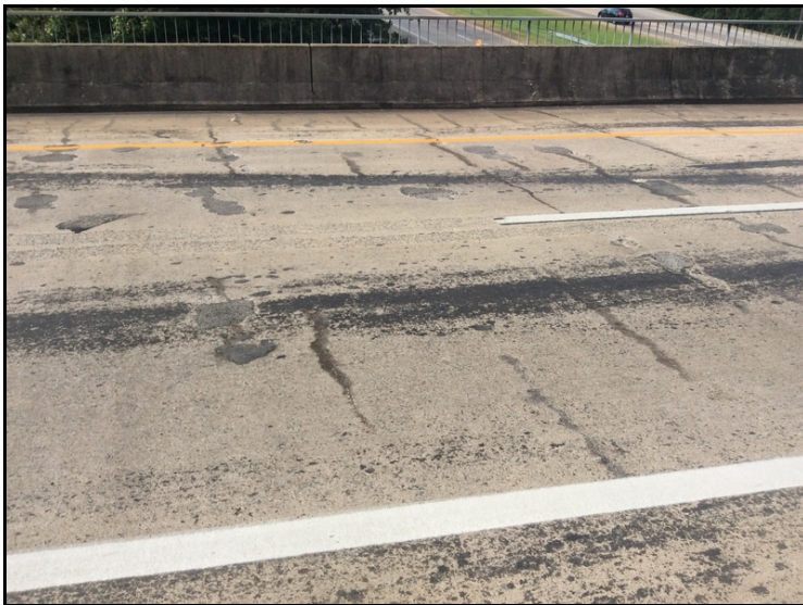
Span 4 spalls filled with asphalt
