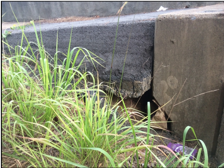
Bent 1 void under approach rail and sidewalk
