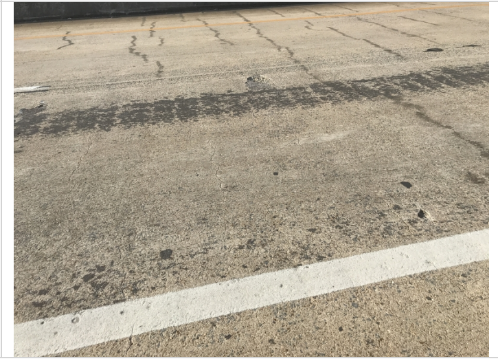
Cracks in span 2
