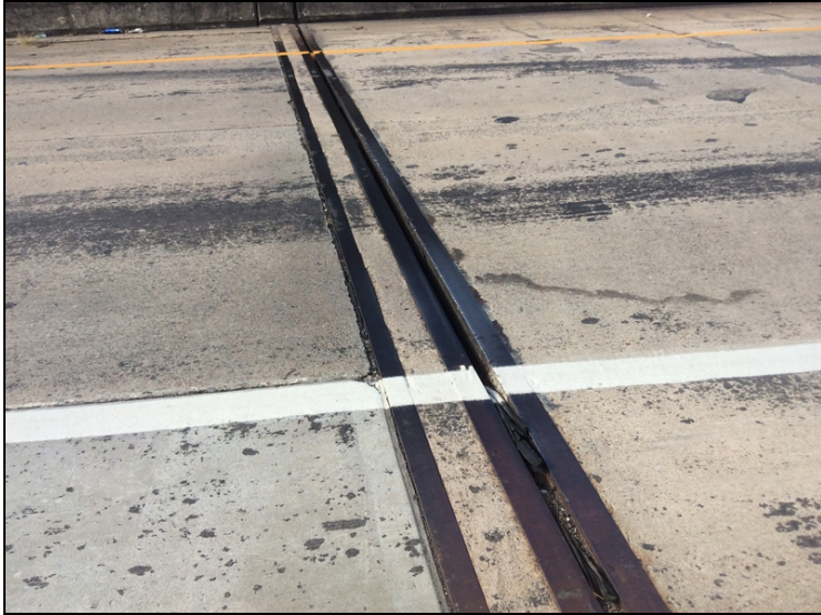
Bent 5 joint seal missing
