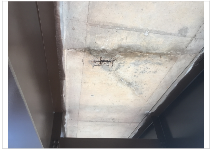
Spalls with rebar in the soffit
