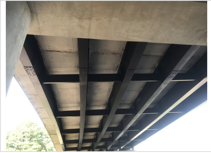
Delamination right of beam 4, second splice plate in span 3
