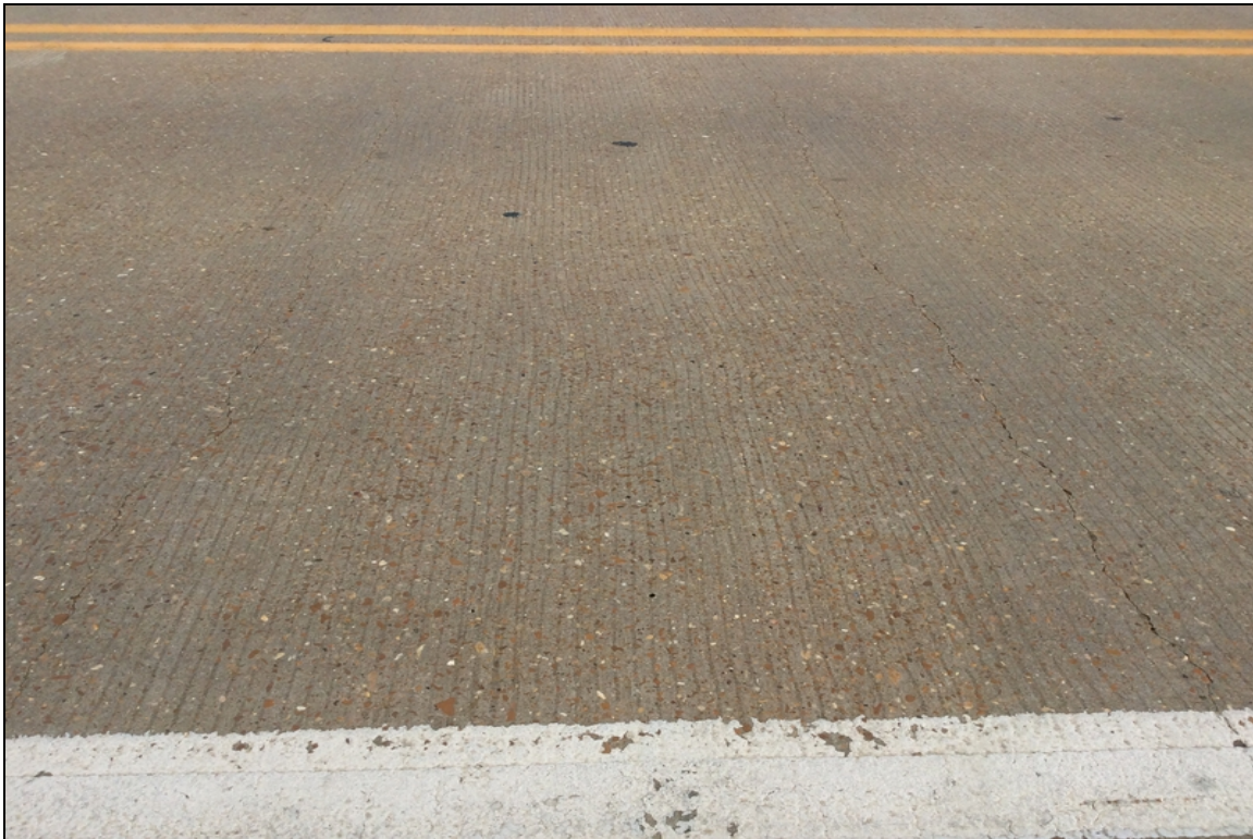
Typical transverse cracking at various spacing throughout the driving surface
