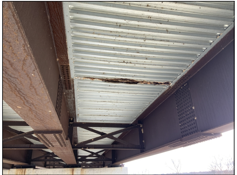
Span 10 at girders 3'4 and 5 active corrosion to sip forms.
