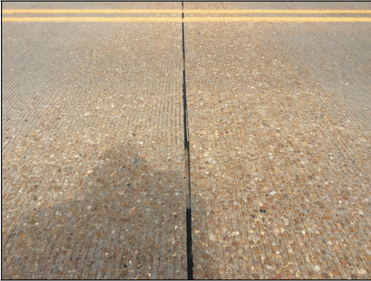
Typical missing and deteriorated saw joints in various locations throughout the structure.
