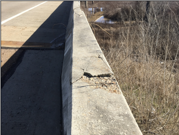
Bent 1 small spall on top of approach bridge rail.
