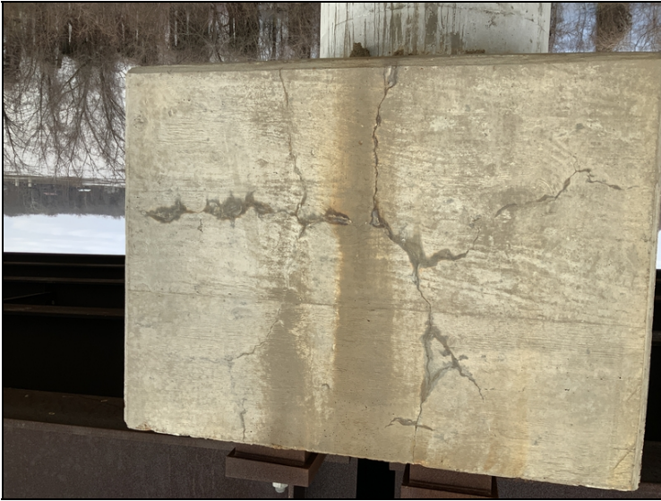
Bent 8 right end of cap epoxy repair that has failed.
