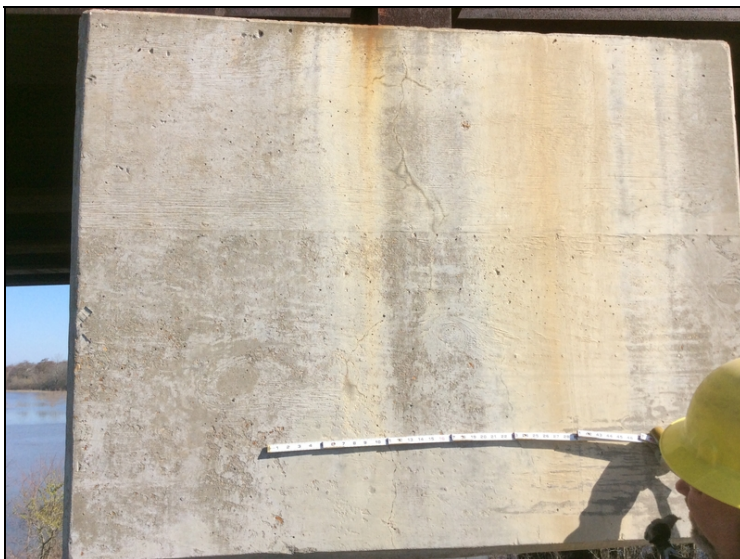
Bent 7 rt. End of cap: small vertical cracking in the ends of the caps
