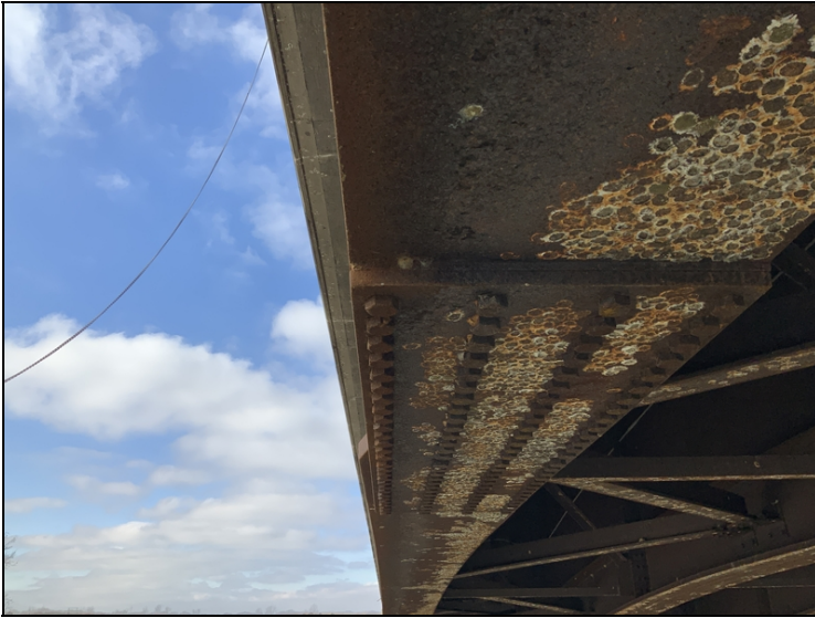
Span 13 girders 1 and 5 active corrosion with flaking rust to bottom flange typical throughout main spans.
