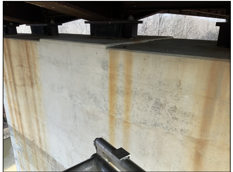
Bent 14 vertical cracking in face of cap typical with all caps.
