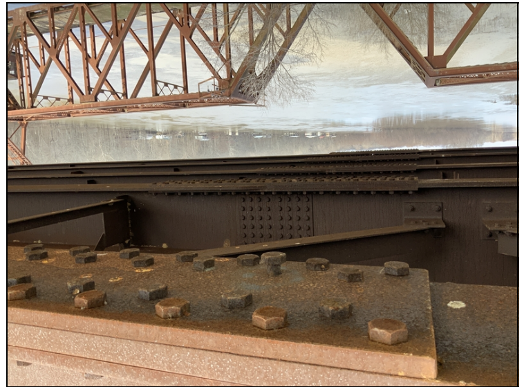
Span 12 first splice plate ahead bent 12 girder 5 loose bolt.
