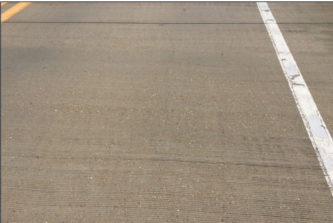
Typical map cracking in random locations throughout the driving surface
