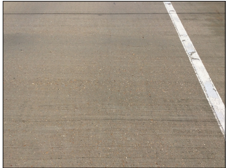
Typical map cracking in spans 12 thru 13
