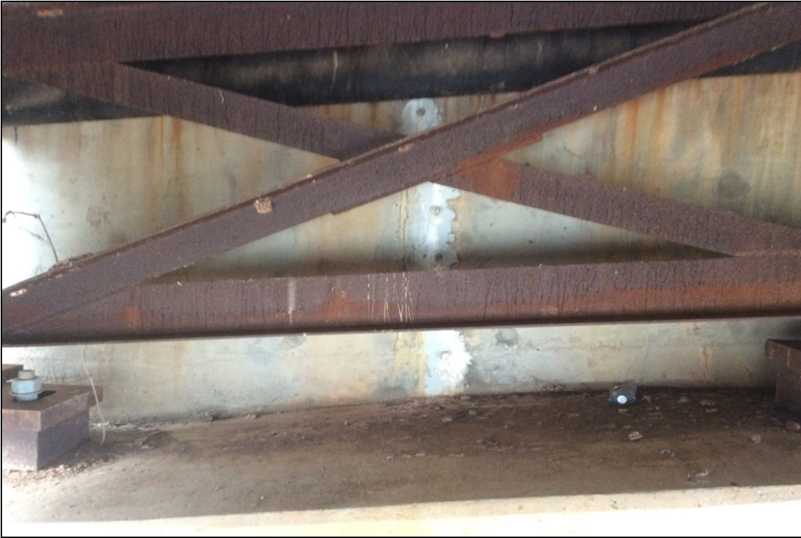
Bent 1 (West Abutment) has 3 epoxy crack in bays 2 thru 4 and are functioning as intended
