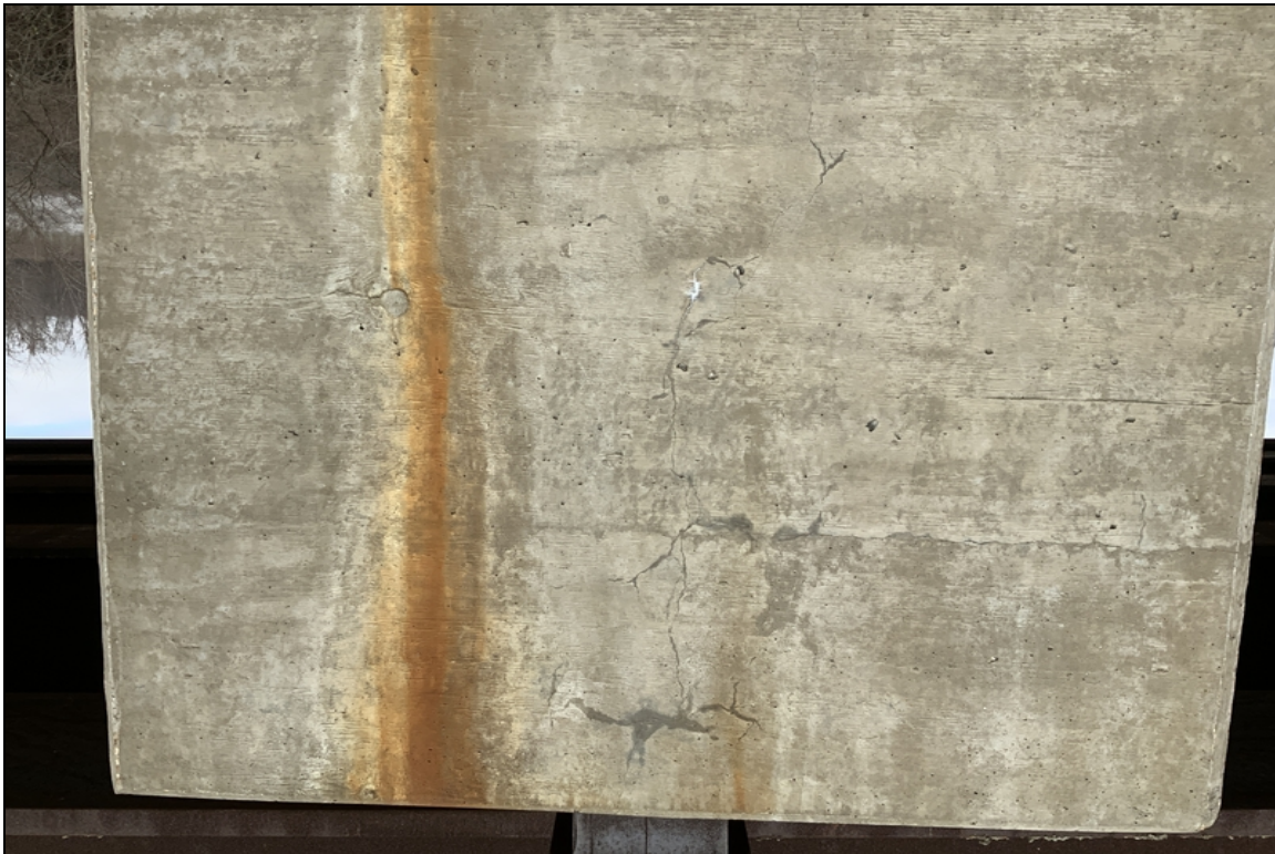
Bent 6 right end of cap map cracking.
