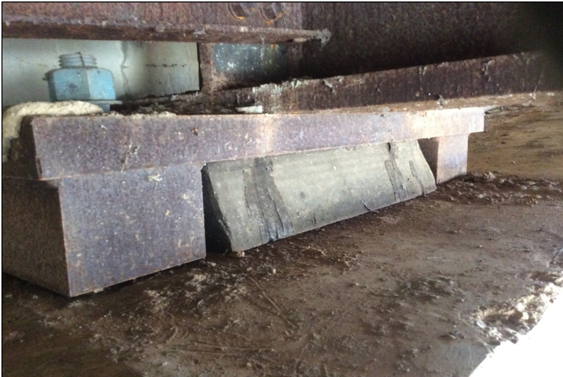
Typical condition of the bearings at the West Abutment
