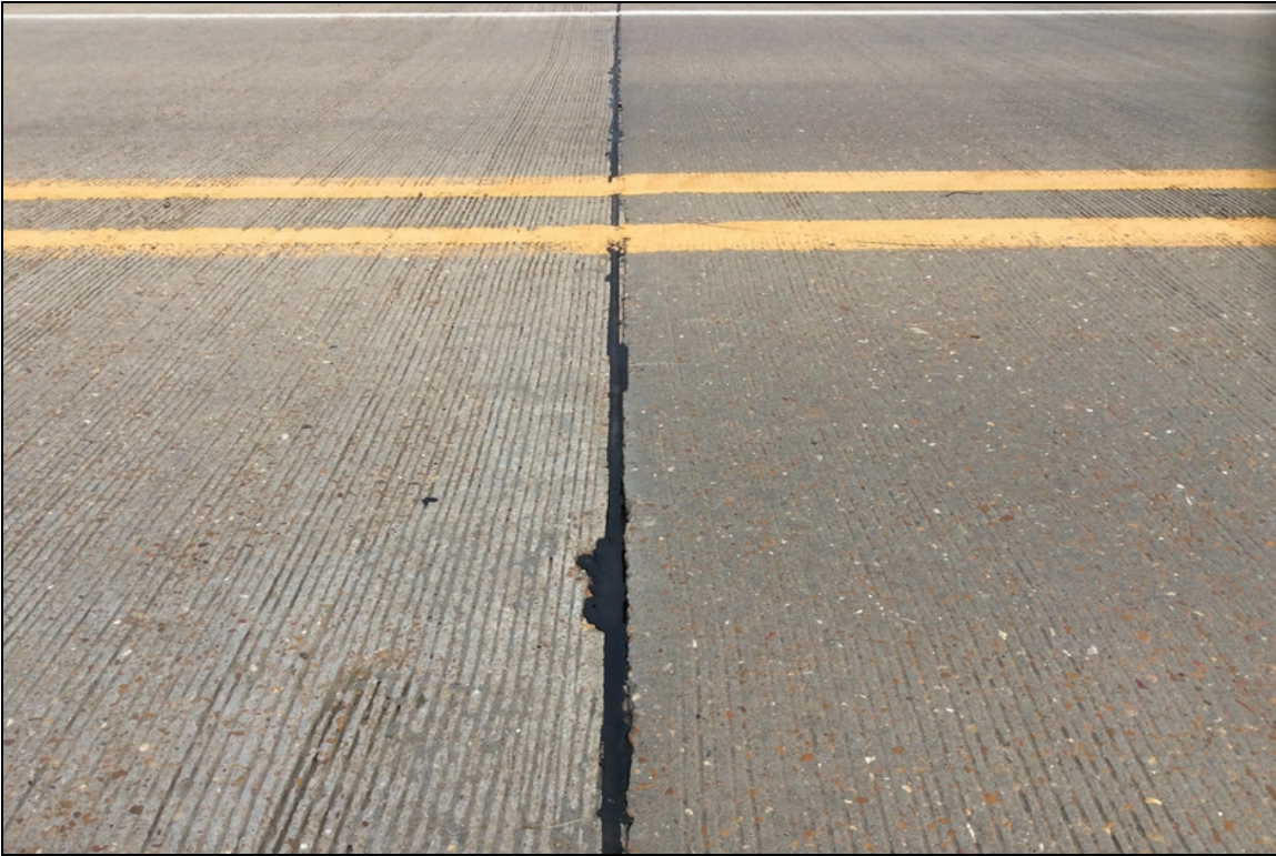
Various saw joints throughout the driving surface has deteriorated and is causing water to leak through and corrode the SIP forms
