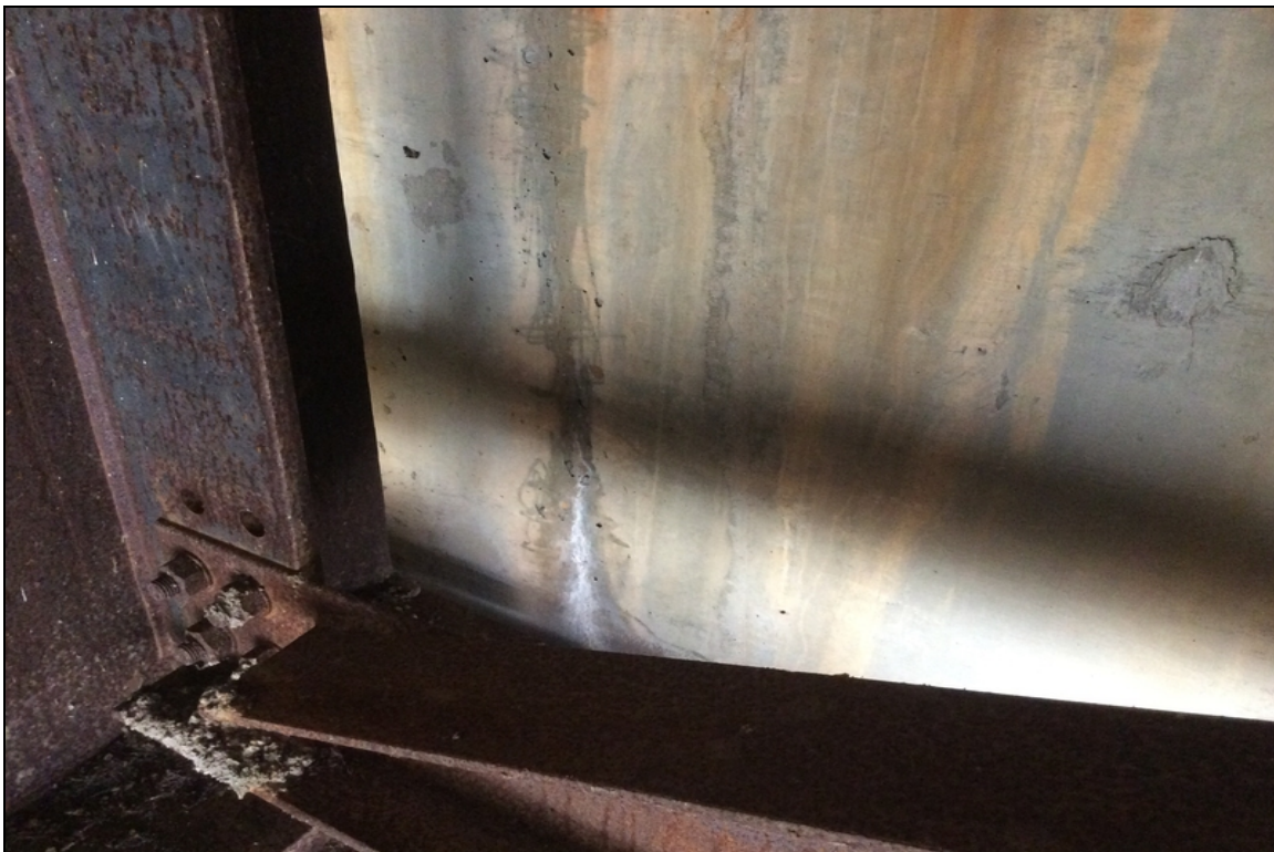
West Abutment has one vertical crack with efflorescence
