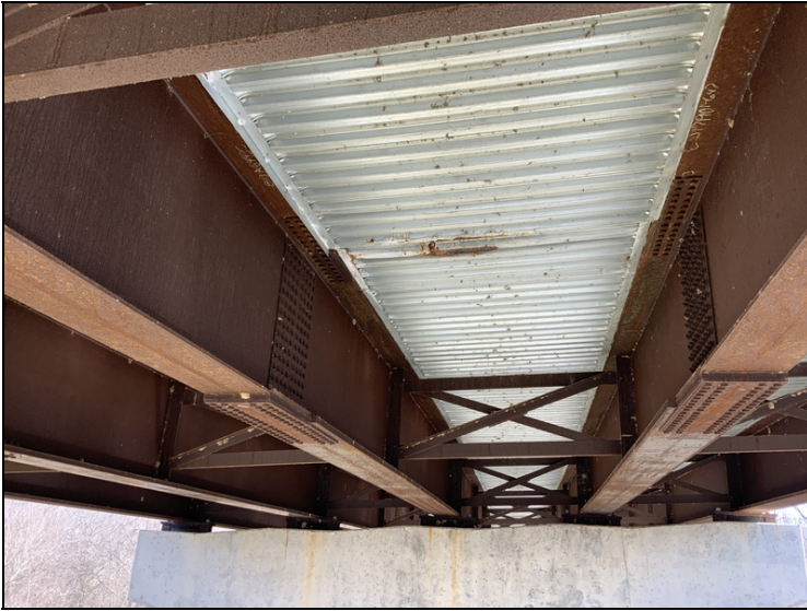
Span 16 between girders 3 and 4 active corrosion to sip forms.
