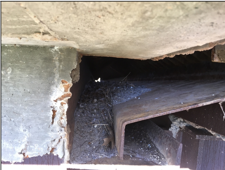
Bent 18 joint partially full.
