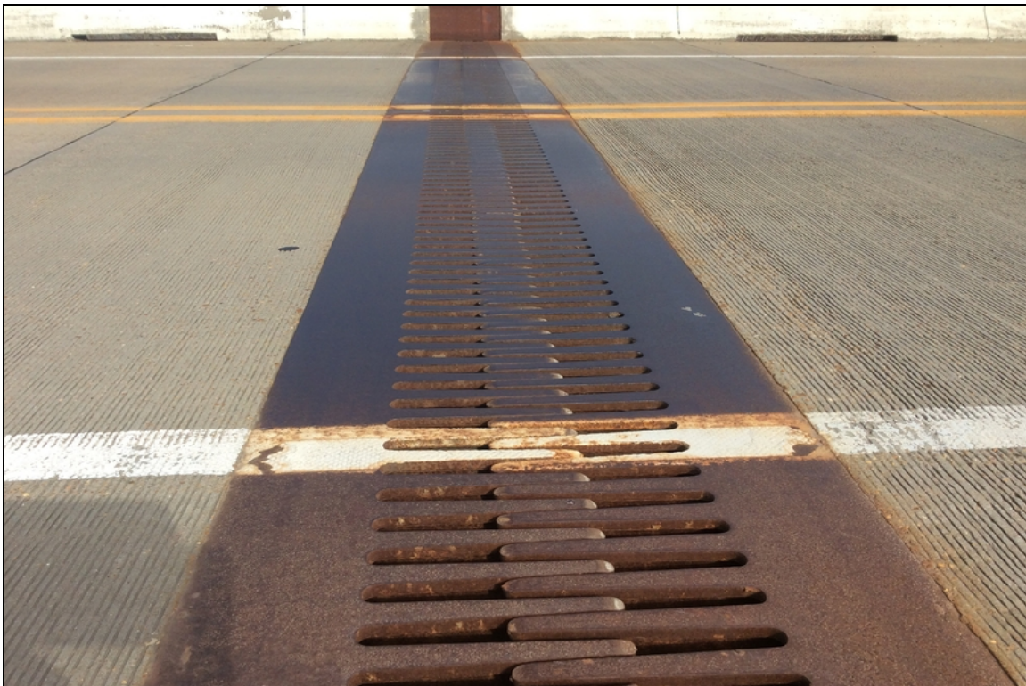
Typical condition of the assembly joints
