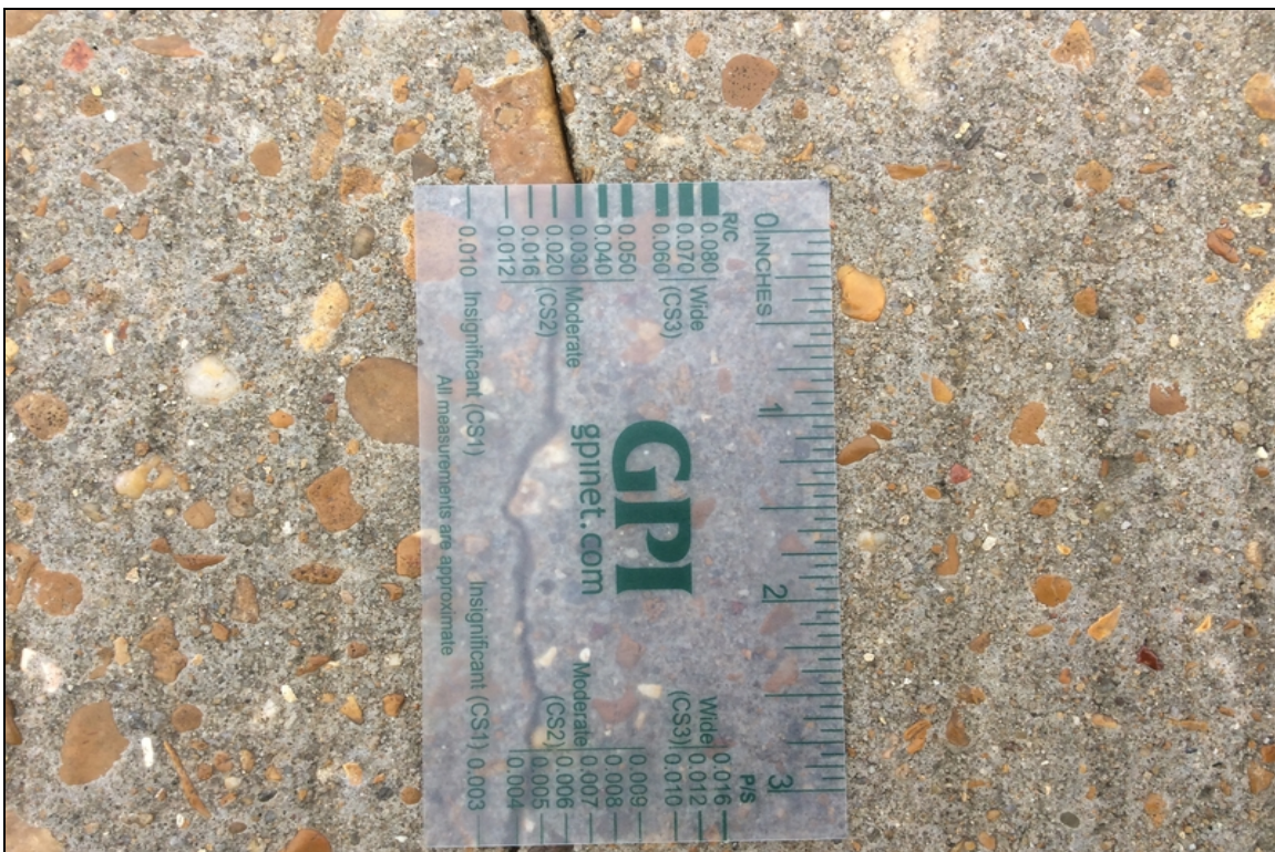
Typical crack width throughout the driving surface
