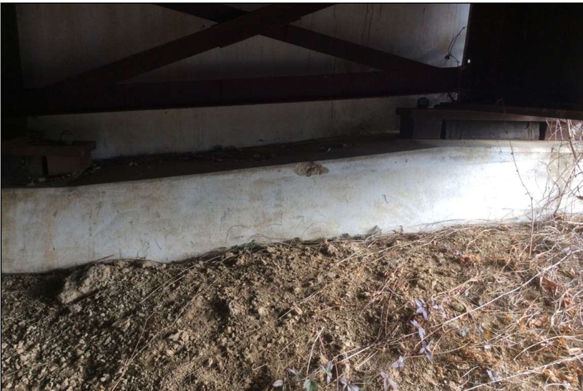
Bent 24 (East Abutment) has one shallow spill along the bridge seat between bay 4
