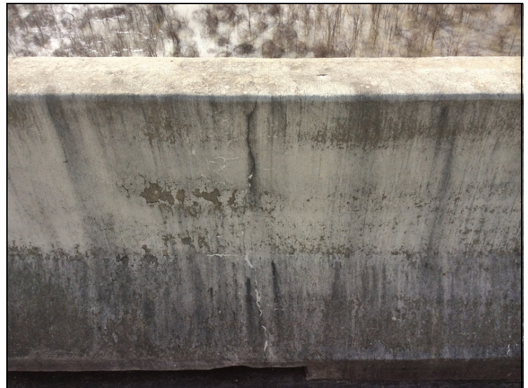
Typical vertical cracking in various locations throughout the structure
