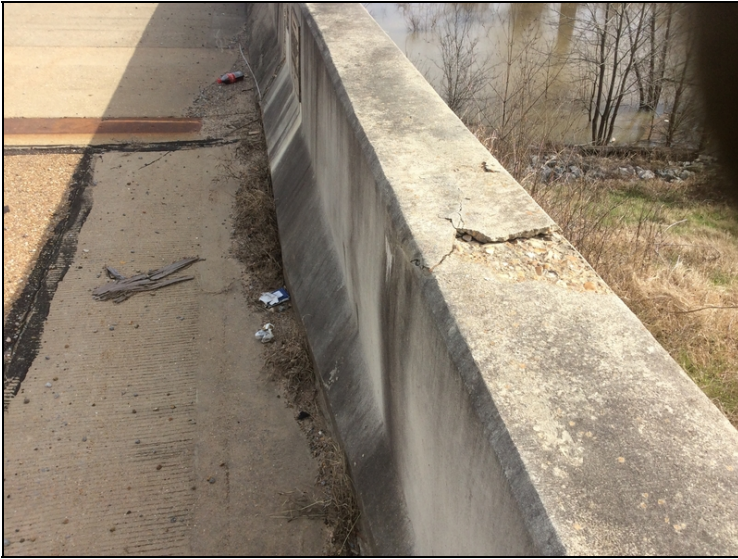
Approach railing at Bent 1 (RT) has one spall on top of the bridge railing
