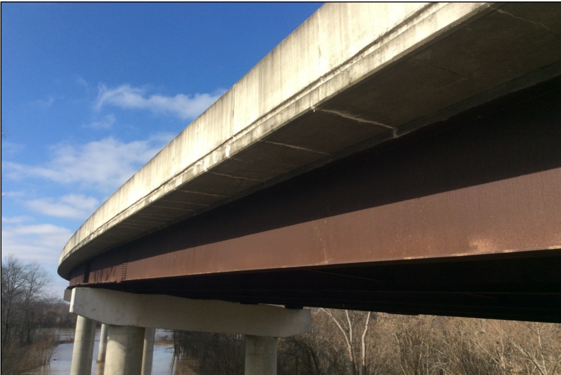
Typical transverse cracking with efflorescence along the overhang throughout the structure (visible from the under surface of the deck)
