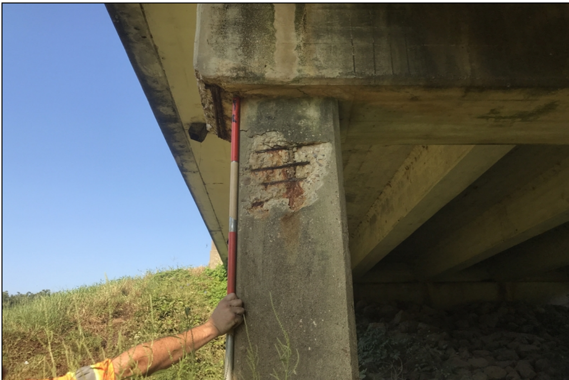
Bent 2, pile 5: spall with exposed rebar
