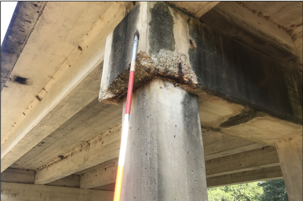
Right side bent 8 cap is spalled with exposed rebar that has significant section loss
