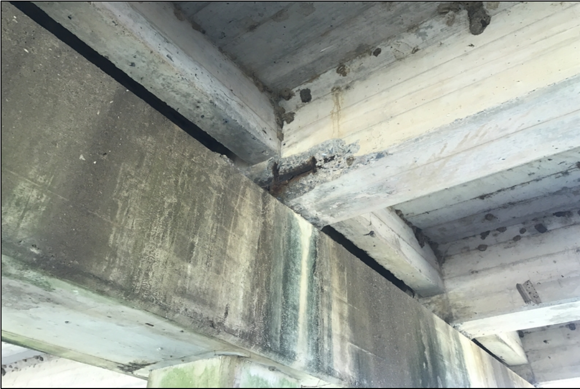
Span 1, girder at bent 2: spall with exposed rebar
