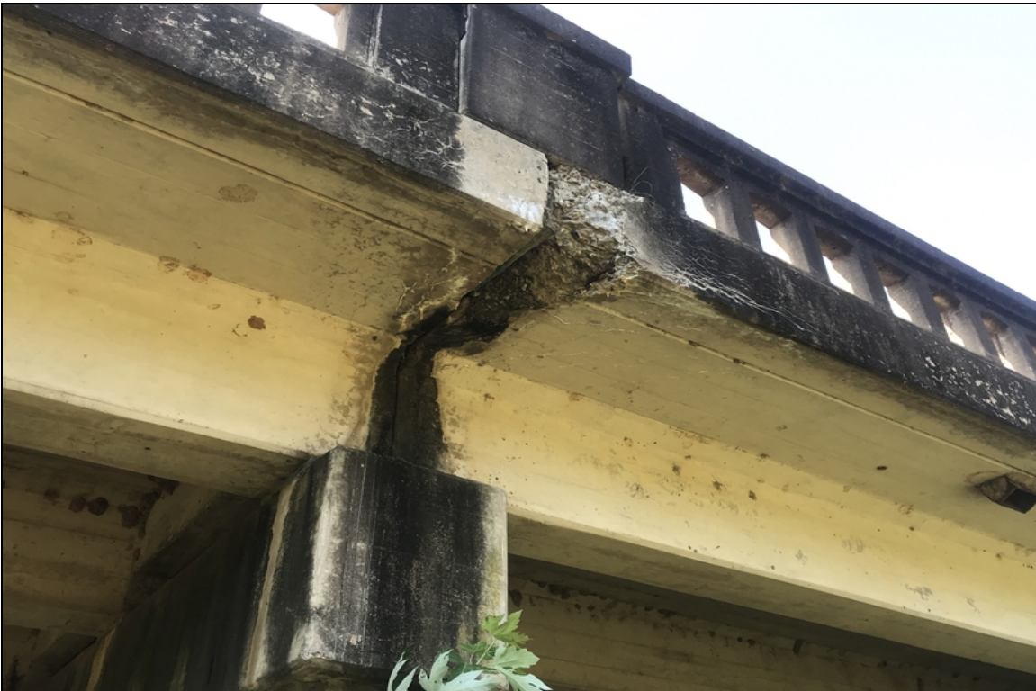
Left side span 1, at bent 2: large spall at the end of the span with exposed rebar
