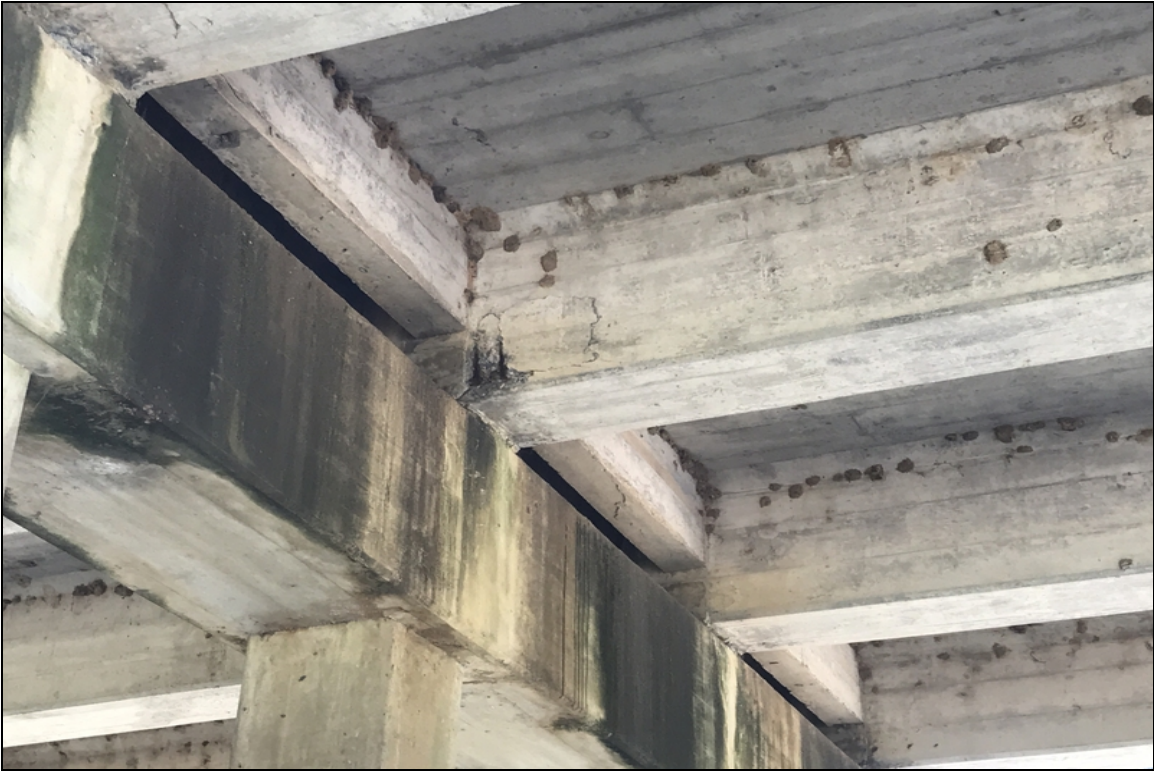
Span 7, girder 3 @ bent 8: spalls with exposed rebar
