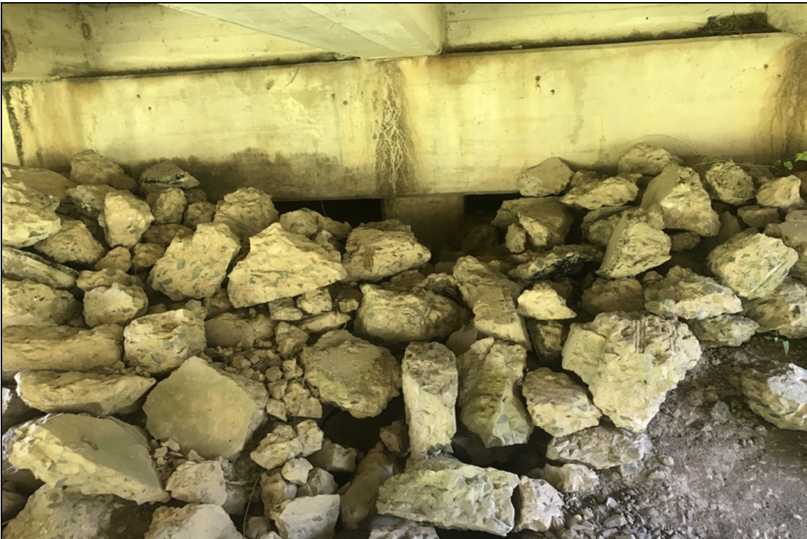
Bent 1: erosion action has exposed pile at the center of abutment
