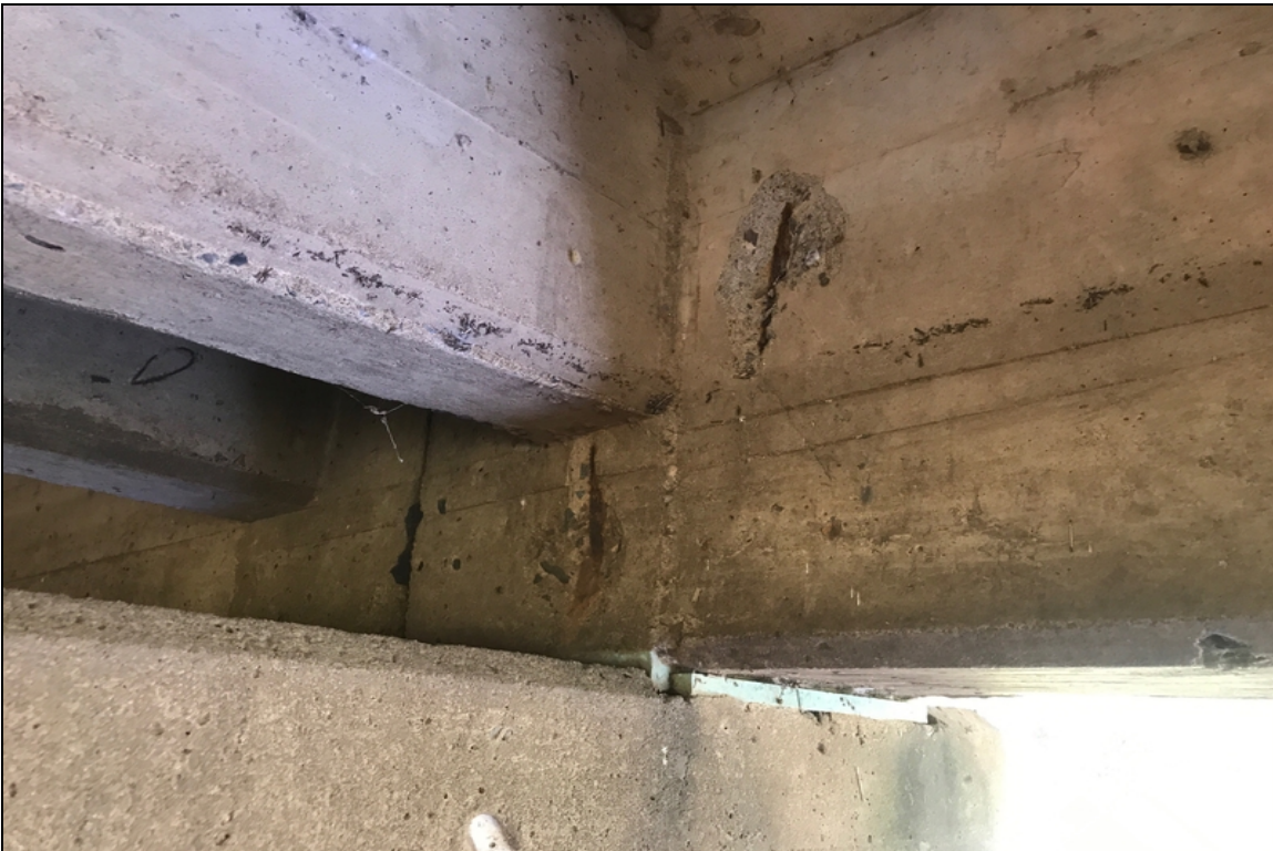
Span 2, girder 1 @ bent 2: couple small spalls with exposed rebar
