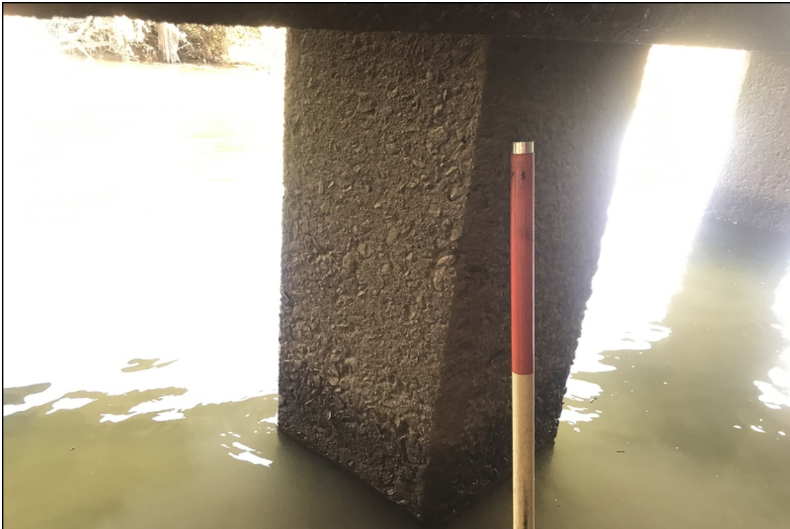
Bent 3, pile 2: pile has heavy abrasion, all pile are in similar condition
