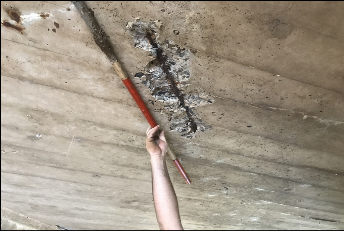
Span 3: soffit has a spall with exposed rebar
