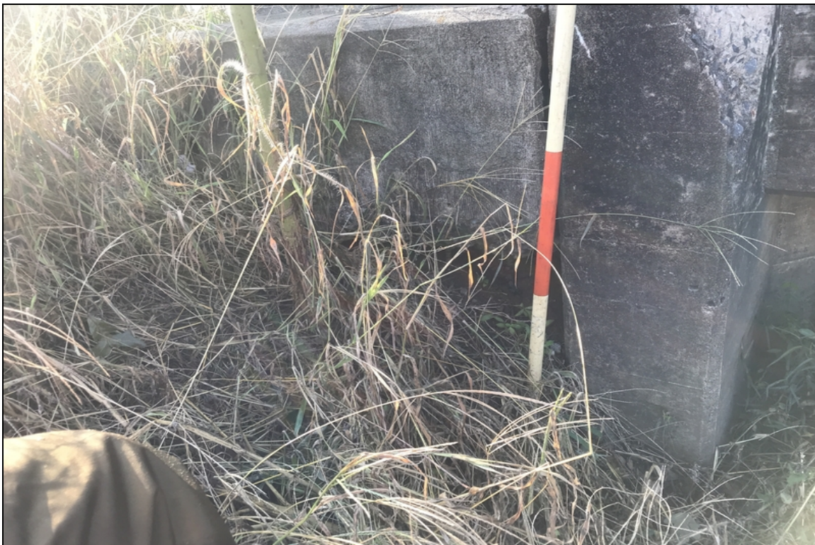
Bent 4: erosion action has undermined the left concrete rail end treatment.
