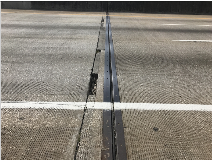
Bent 7 east abutment top of backwall spalls with rebar exposed
