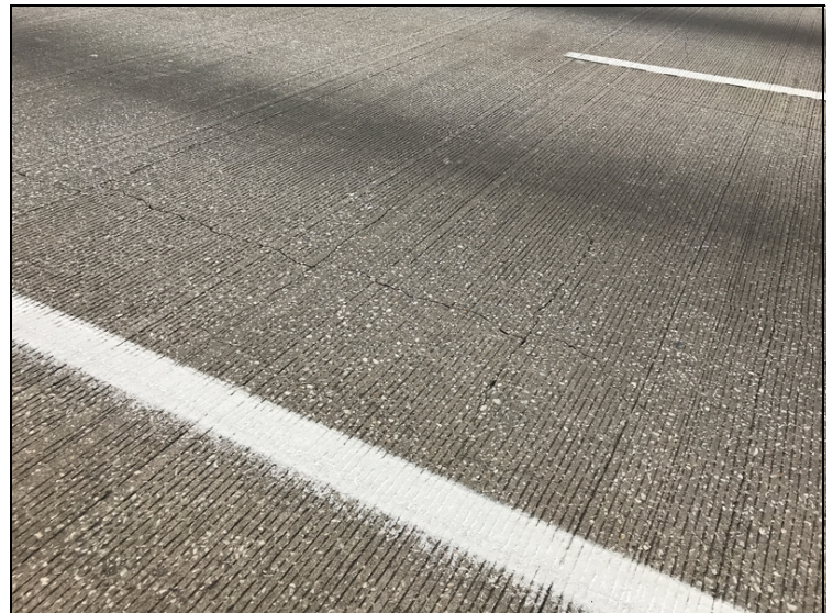
Span 5 Unsealed transverse and longitudinal cracks in all spans up to 0.040 inch
