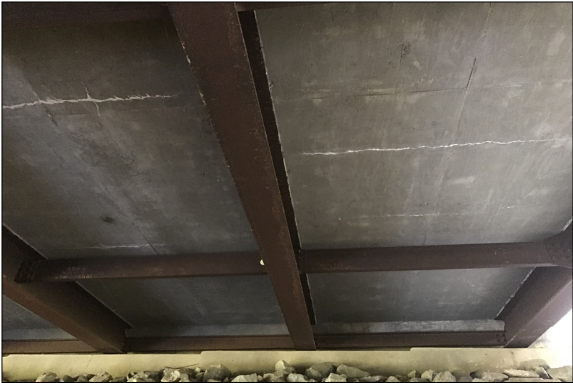
Span 7: soffit with multiple transverse cracks with efflorescence staining.
