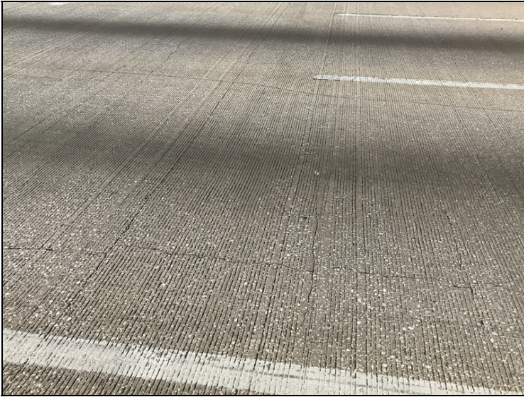
Span 5: unsealed transverse and longitudinal cracking up to 0.040" in width.
