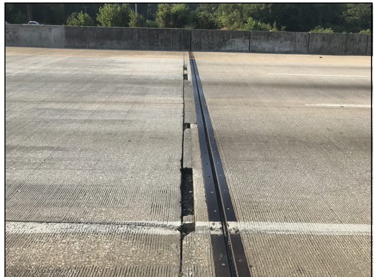
Bent 7: multiple open spalls in the headwall
