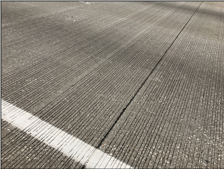
Span 2 Unsealed transverse and longitudinal cracks in all spans up to 0.040 inch
