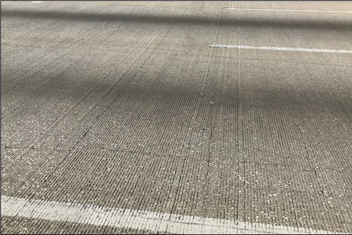
Span 5: unsealed transverse and longitudinal cracking up to 0.040" in width.
