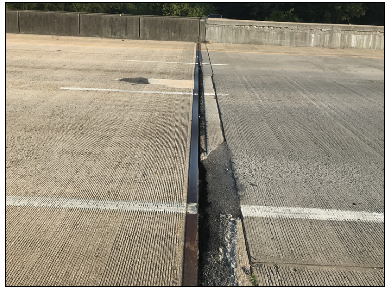
Bent 7: entire joint seal missing, spall filled with asphalt in the right lane, spall filled with asphalt in the center lane, and joint armor missing in the right 2 lanes.
