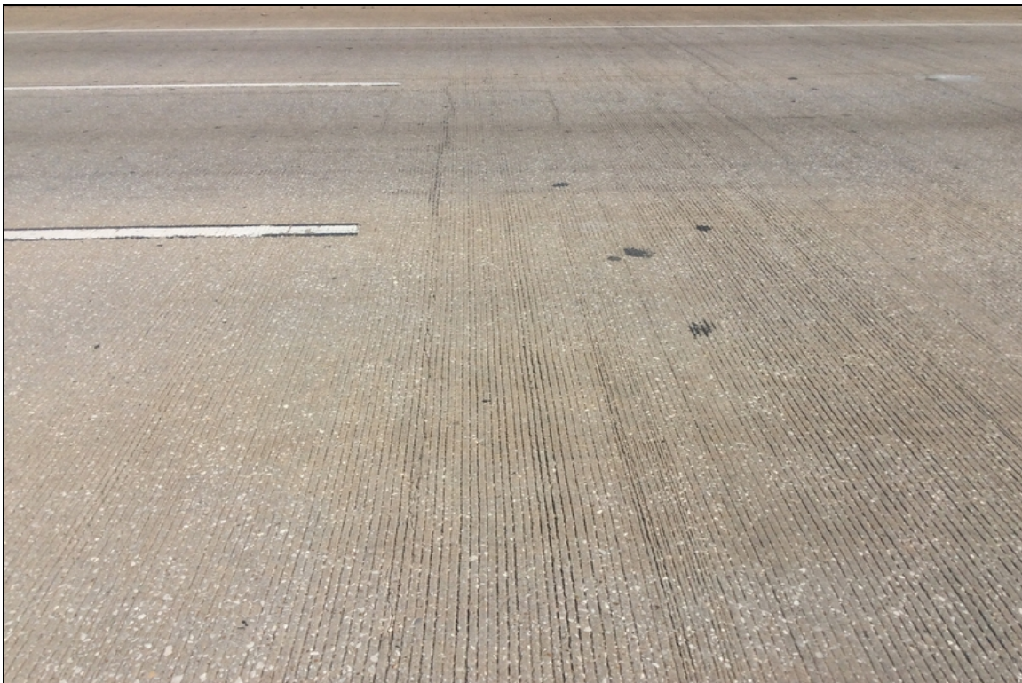
Span 2, large transverse cracks.
