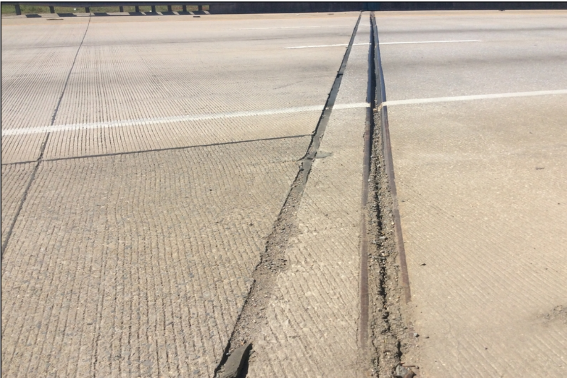
Bent 4 joint impacted by debris.
