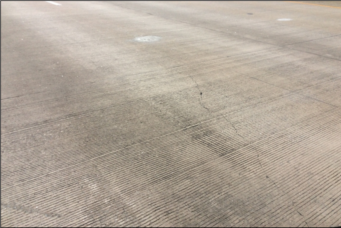
Bent 4 approach slab, large crack.
