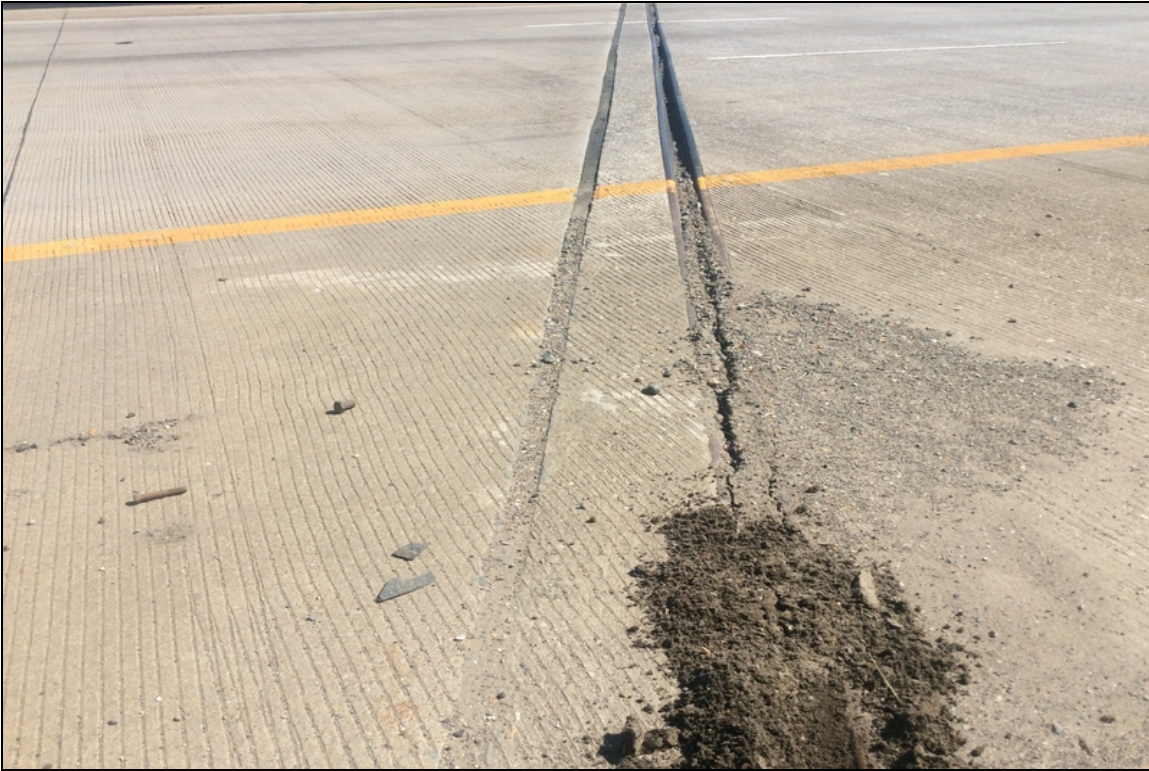
Bent 1 joint impacted by debris.
