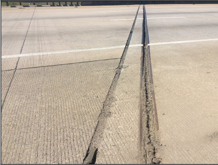
Bent 4 joint impacted by debris.
