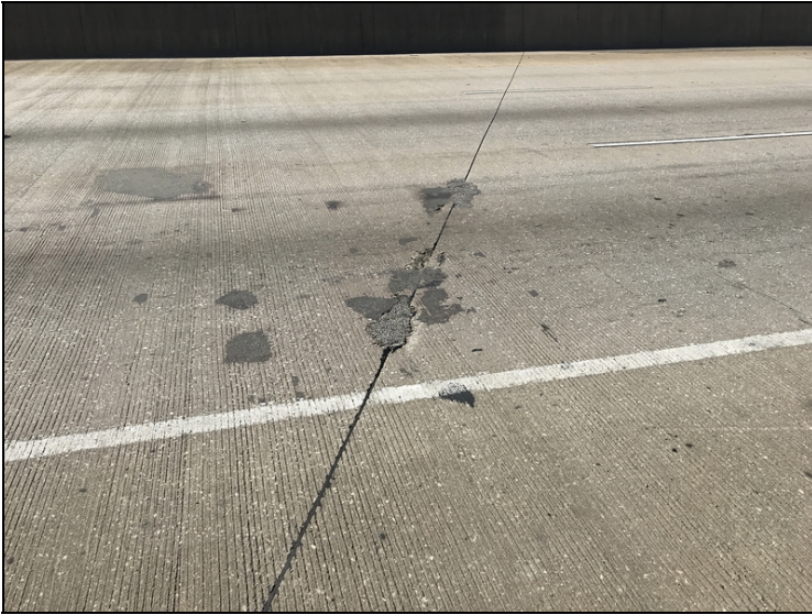
Spalls filled with asphalt over Bt. 3.
