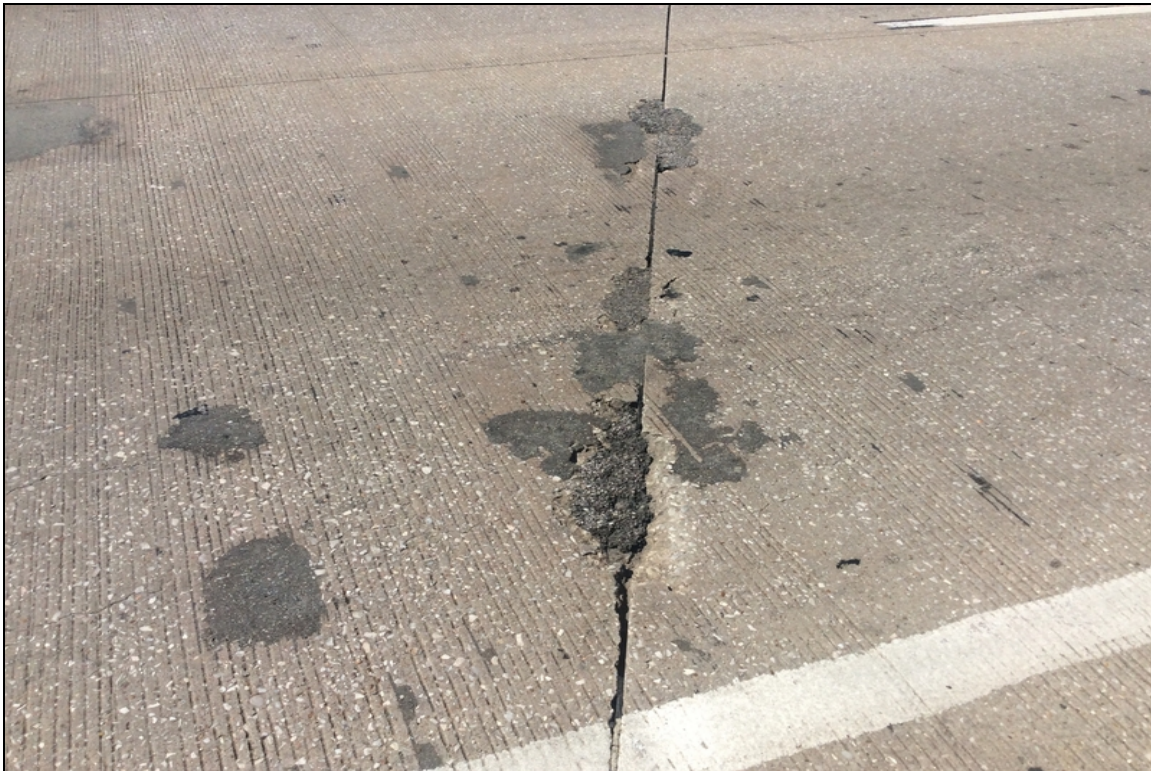
Bent 3, asphalt patches are failing.
