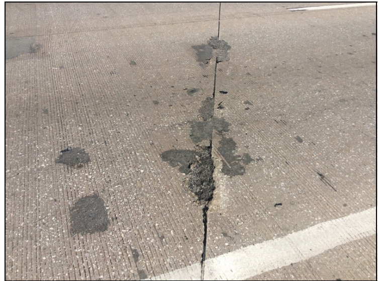
Bent 3, asphalt patches are failing.
