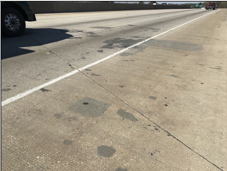
Span 3, spalls patched with epoxy & asphalt.
