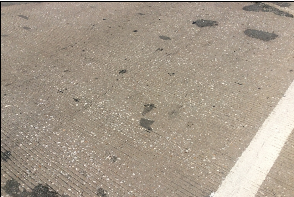
Span 3, large cracks and patches.
