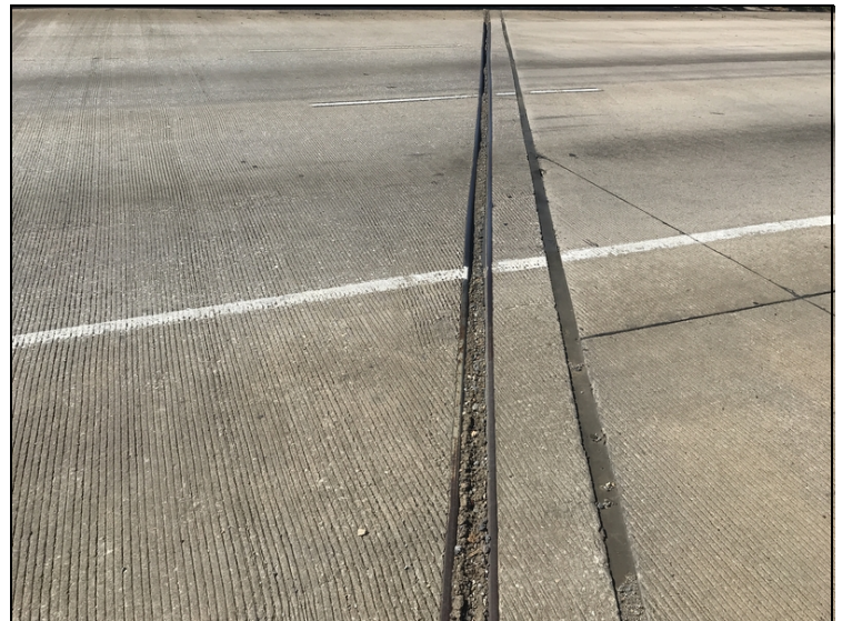
Bt. 1, joint full of debris.
