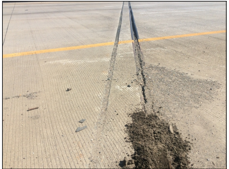
Bent 1 joint impacted by debris.
