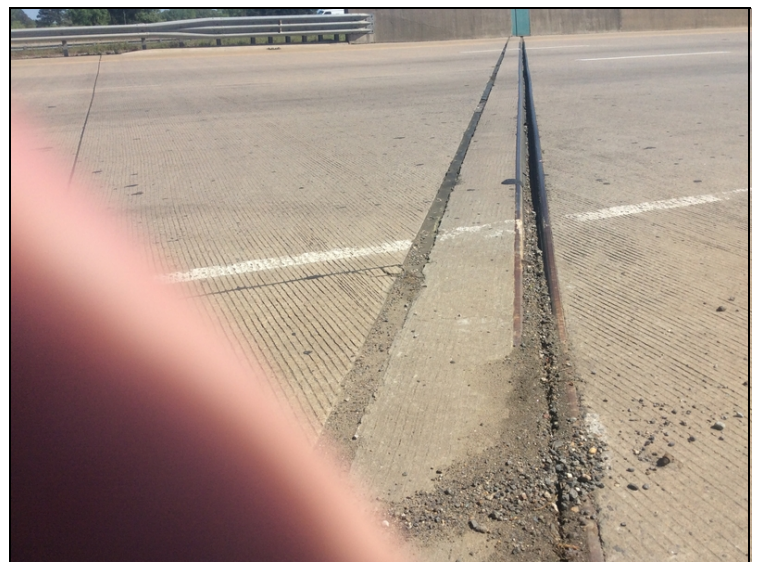
Bent 1, debris impacting the joint.
