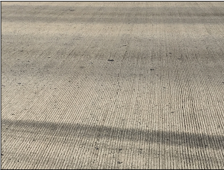
Deck crack up to 0.030".
