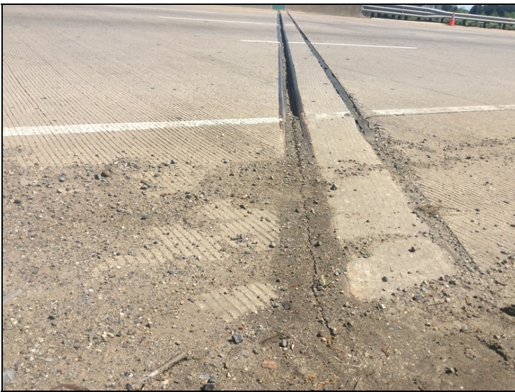
Bent 4, debris impacting the joint.
