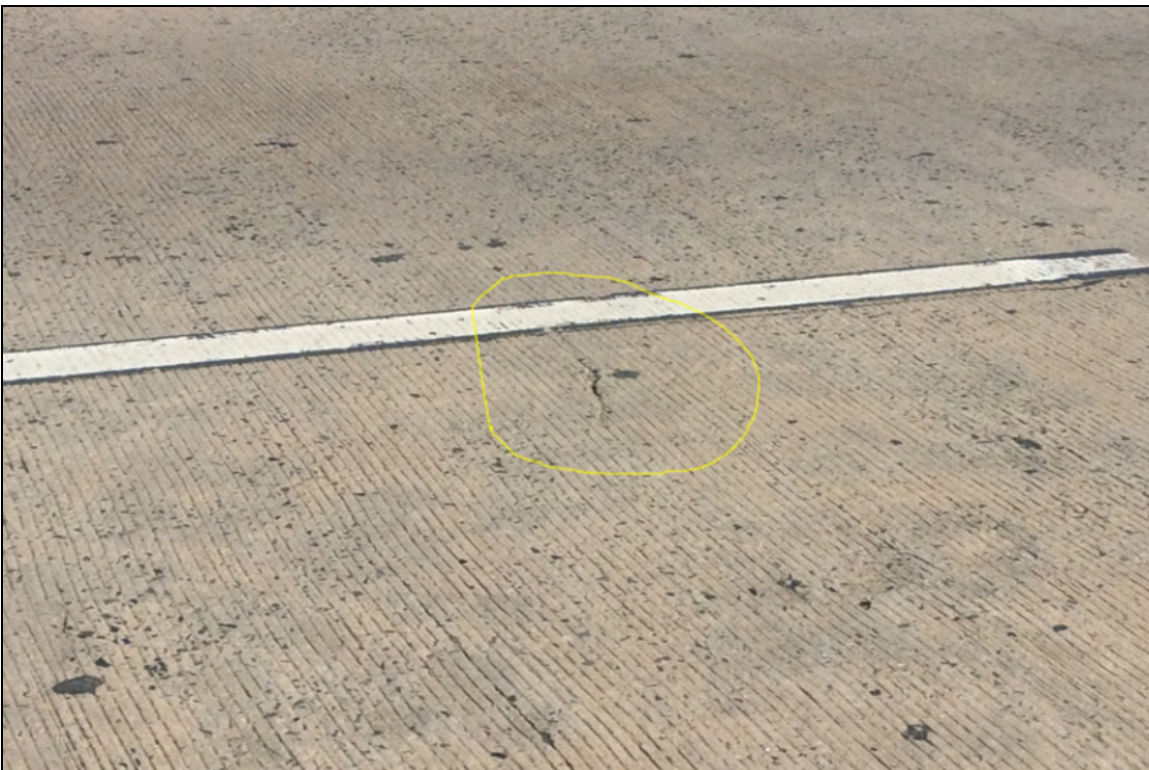
Span 3, large crack.
