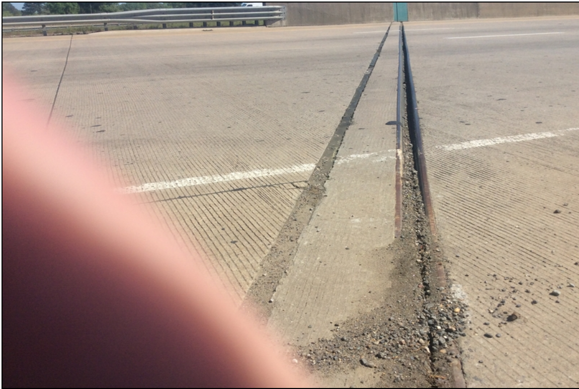
Bent 1, debris impacting the joint.
