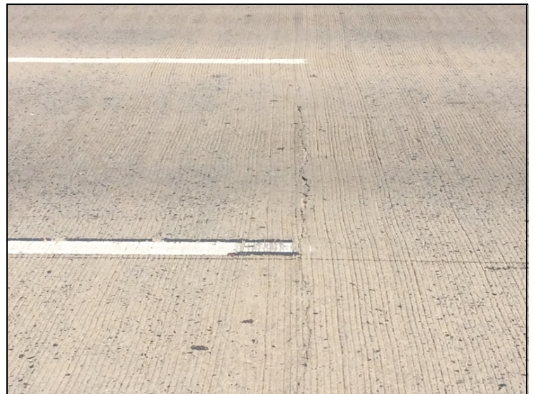
Span 2, large transverse cracks.
