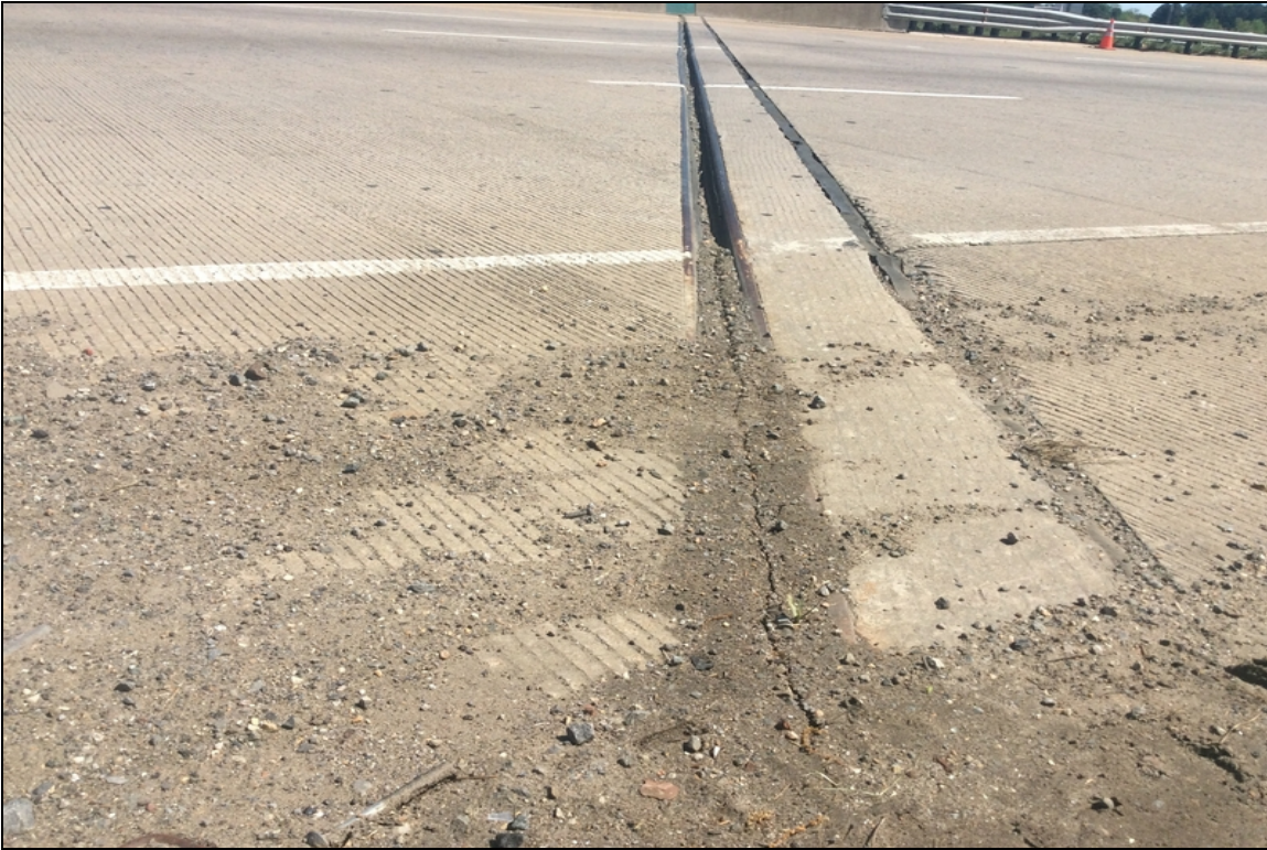
Bent 4, debris impacting the joint.
